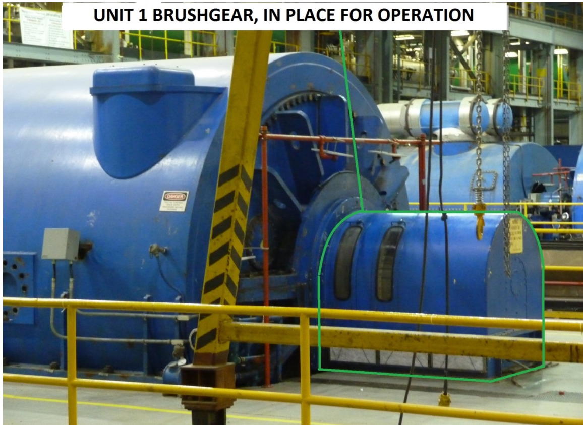
Figure 1- Unit 1 Brushgear Housing
