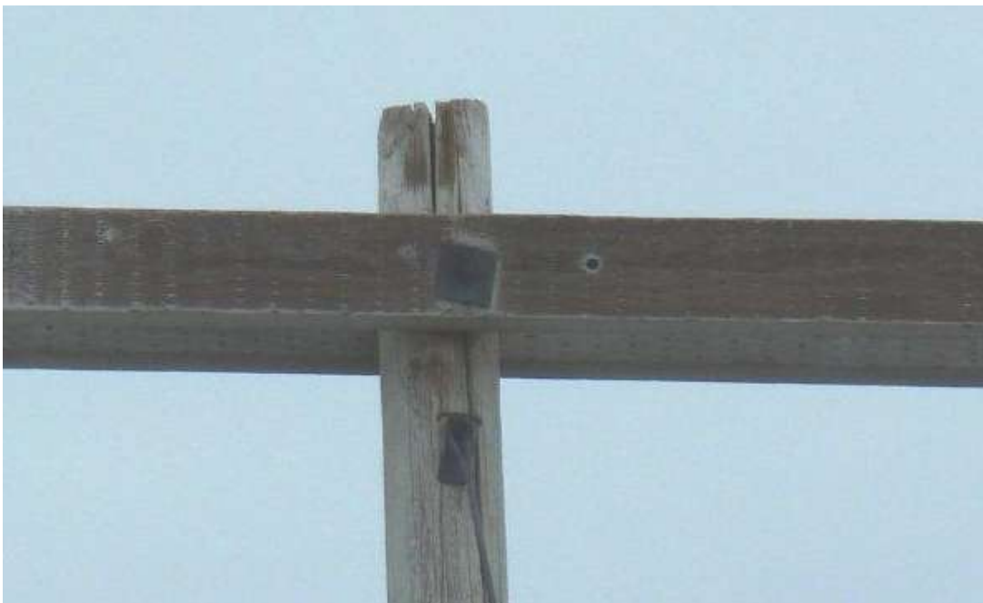
Figure 20 – 68L - Deteriorated pole and crossarm
