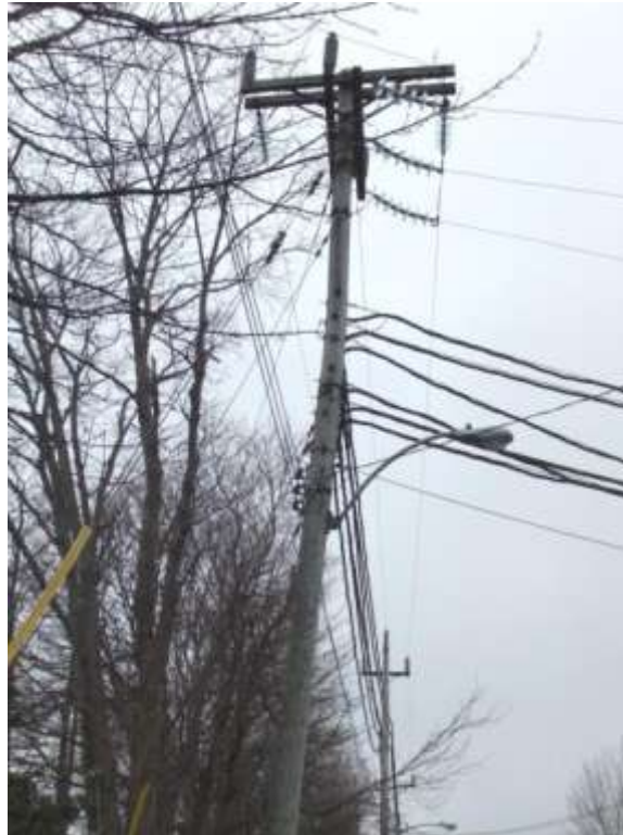
Figure 3 – 12L - Pole bent due to significant loading caused by high voltage aerial cables
