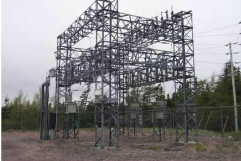
Low Voltage Distribution Bus Structure (Feeder Infrastructure)
