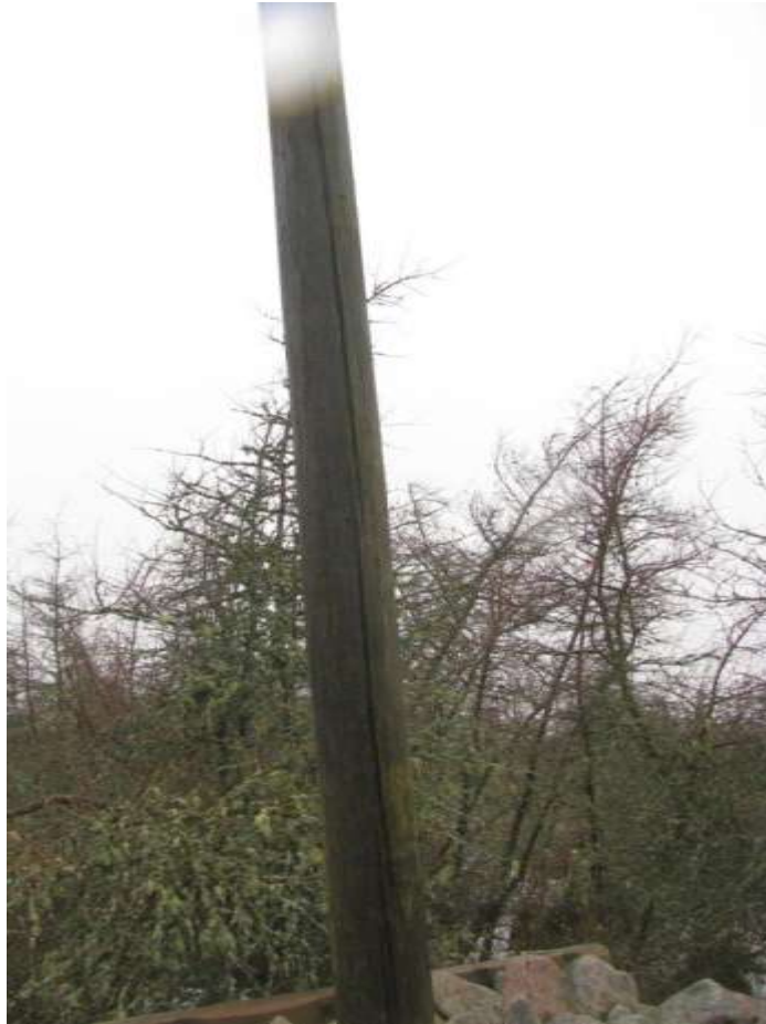
Figure 11 – 18L - Pole with severe checks
