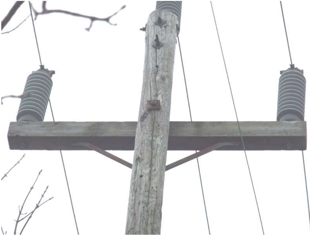
Figure 1 – 12L - Pole showing checking around bolts
