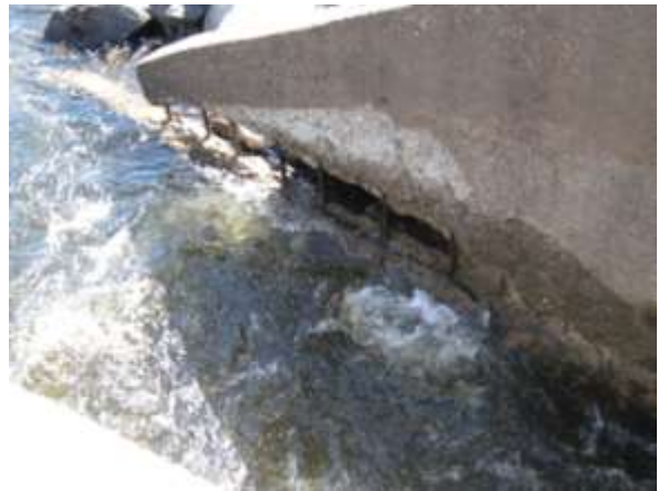
Figure 10 – Deteriorated Wingwall Concrete
