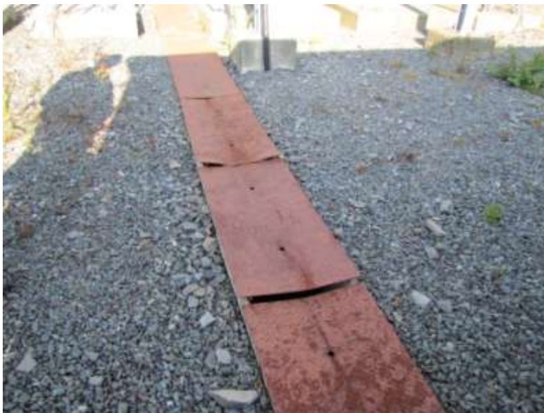
Deteriorated Cable Trench Covers
