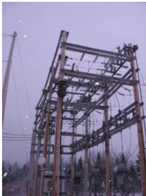
Low Voltage Bus Structure (Wood Poles and Cross Arms)
