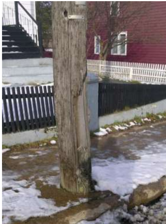
Figure 6 – 13L - Pole showing vehicular or snow plough damage
