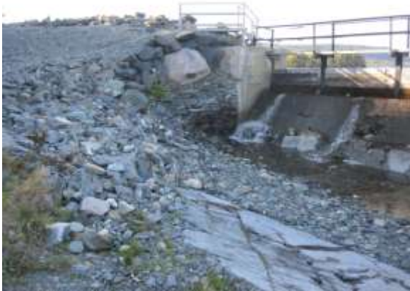
Figure 6 – Deteriorated Concrete and Abutment Prone to Washout
