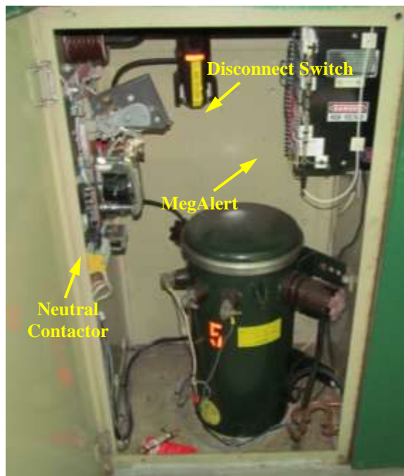
Figure 3 – Neutral Grounding Transformer
