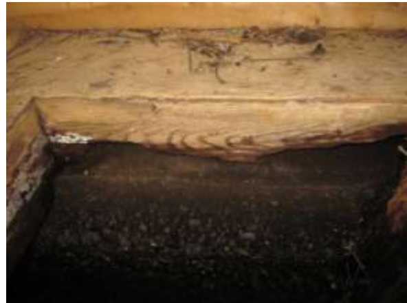
Figure 2 – Deteriorated Timber Deck
