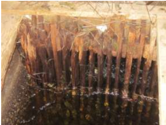
Figure 1 – Deteriorated Trash Rack
