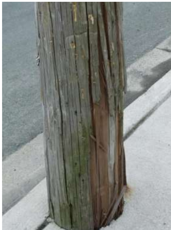
Figure 2 – 12L - Pole showing shell separation and damage
