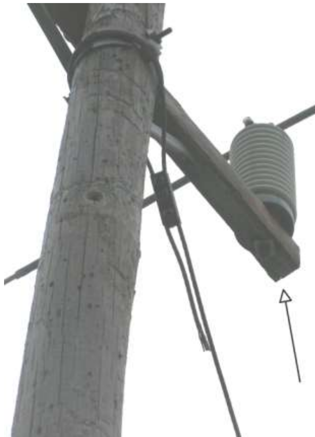
Figure 10 – 18L - Split crossarm and nonstandard guy wire
