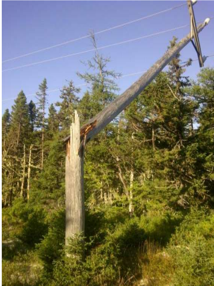
Figure 15 – 35L - Broken pole - Tropical Storm Leslie
