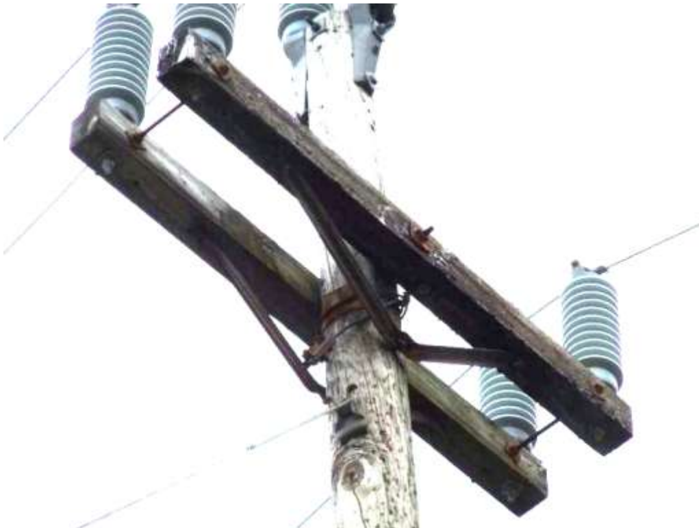
Figure 4 – 12L - Deteriorated Crossarms
