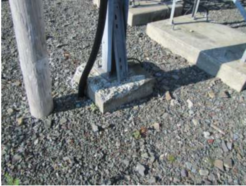
Deteriorated 15kV Pothead Structure Column Foundation
