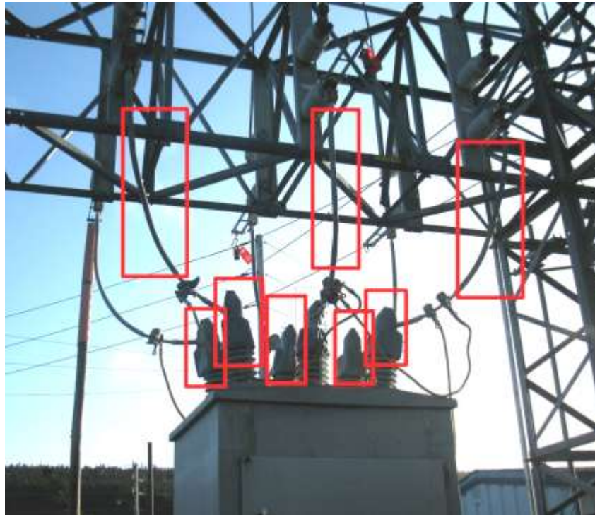
Varmint Protection Example Including Insulated Busing Covers and Leads
