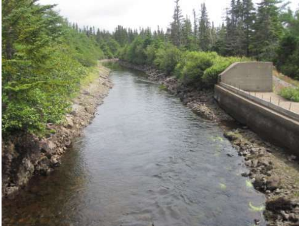
Figure 3 - Minimum operating capacity of approximately 0.9m 3 /s
