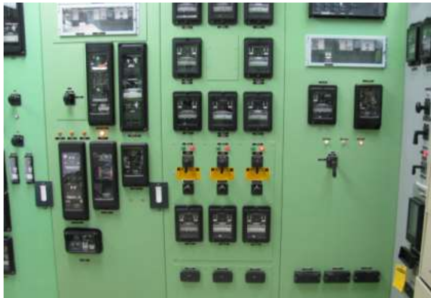
Transmission Line Electromechanical Relay Panels and RTU
