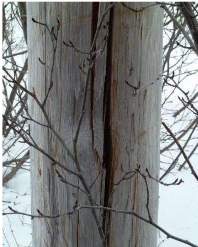
Figure 18 – 68L - Deep check in pole
