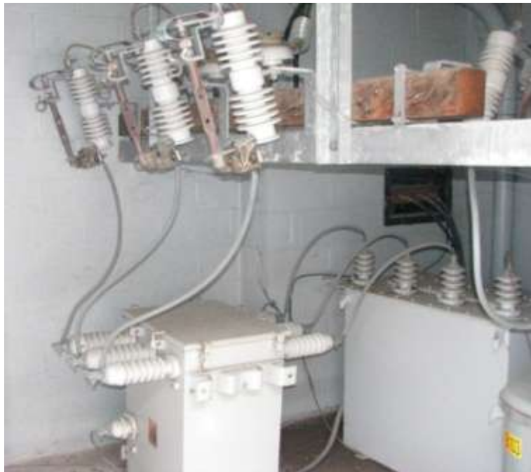
Figure 2: Parks Canada Signal Hill Vault – Metering Tank and Transformer
