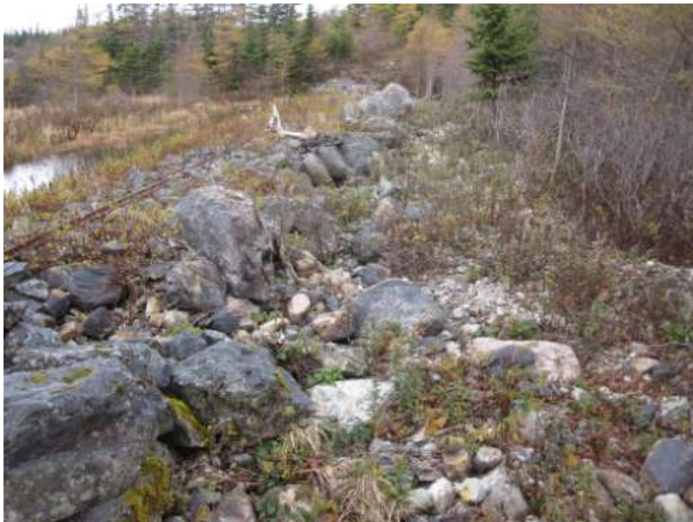
Figure 6 - Poorly Graded Riprap - Cluneys Diversion
