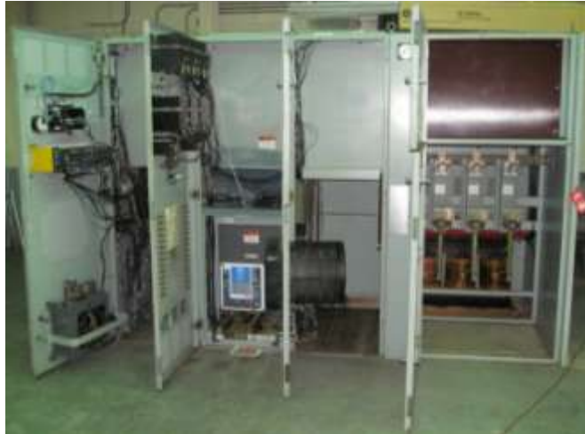
Figure 6 – Switchgear with Doors Open
