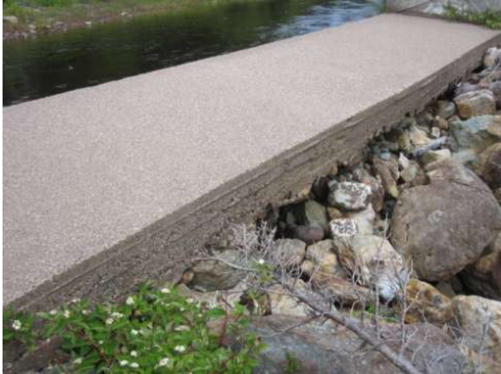
Figure 5 - Typical erosion on a La Manche Canal Spillway
