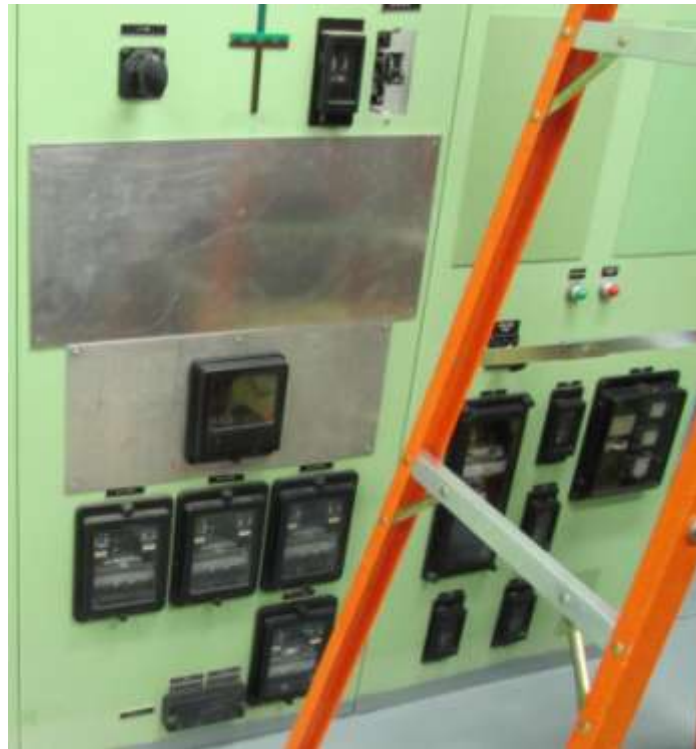
Transformer Protection Panel (Electromechanical Relays)
