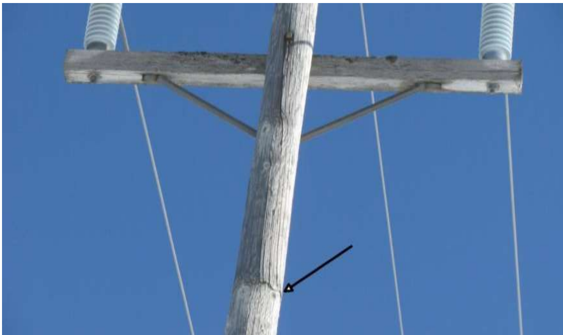
Figure 16 – 35L - Horizontal crack in pole
