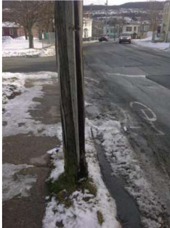
Figure 7 – 13L - Deteriorated pole showing shell separation
