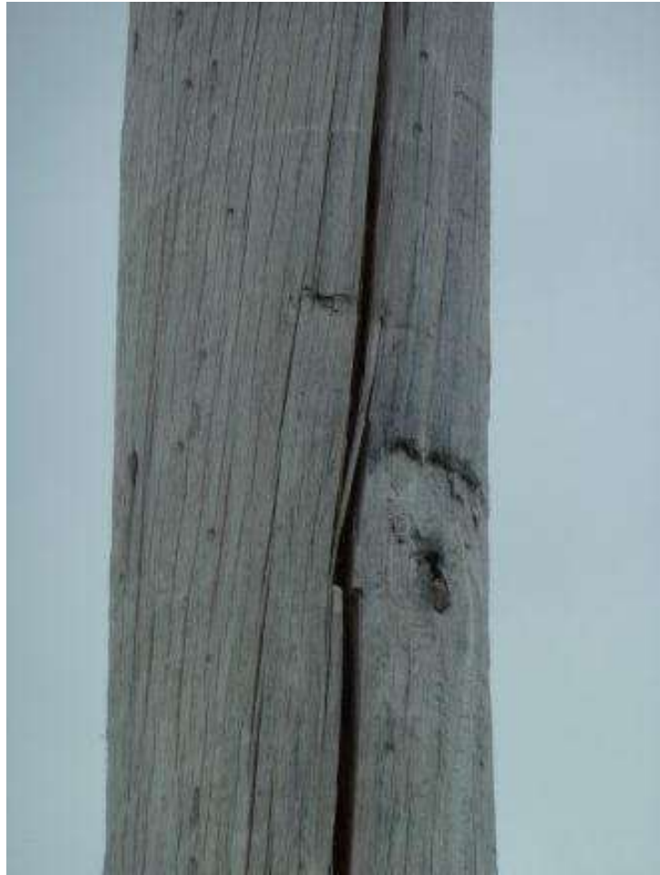
Figure 19 – 68L - Pole showing shell separation
