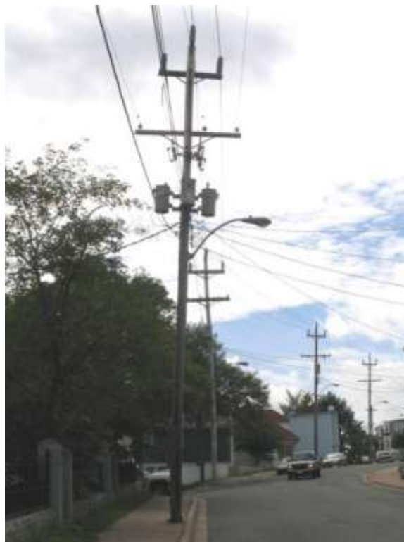
Figure 8 – 13L - Heavily loaded pole leaning
