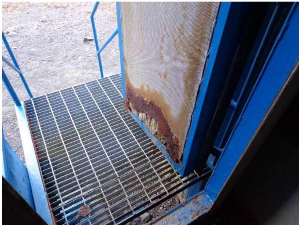
Figure 2 – Corrosion Damage Intake Plenum Door
