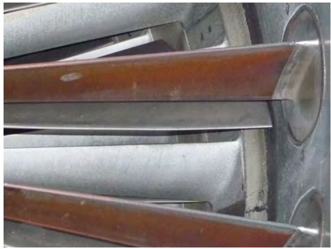
Air intake casing with IGV's
