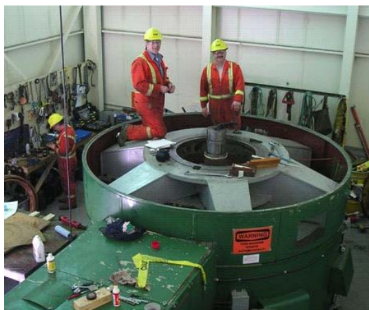
Generation employees work on the Heart's Content Generator to address a machine vibration issue.
