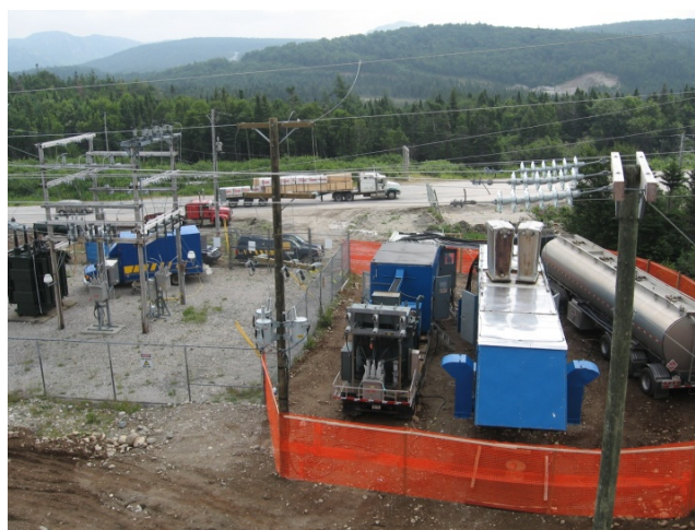
The mobile generation unit was installed at Robinsons substation to facilitate the movement of a transmission line without the need for significant customer outages.
