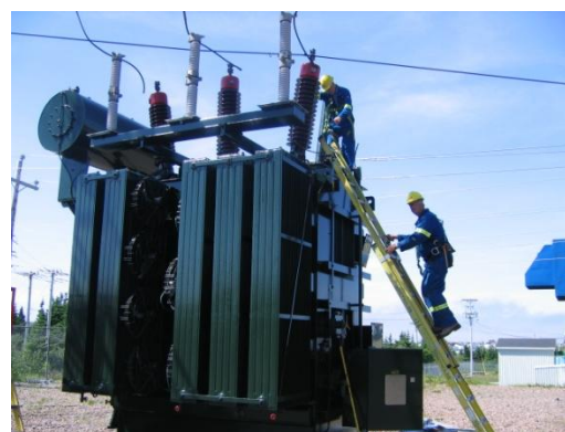
Power Transformer Maintenance
