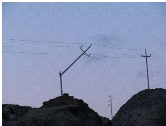
Damage to a structure on radial transmission line 59L during blasting operations by a contractor constructing the Torbay By-Pass Road.
