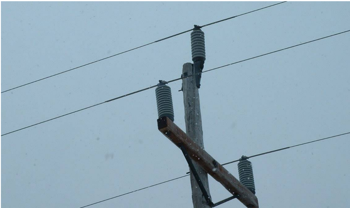
Figure 7 – Deteriorated Pole (Top Split) 111L
