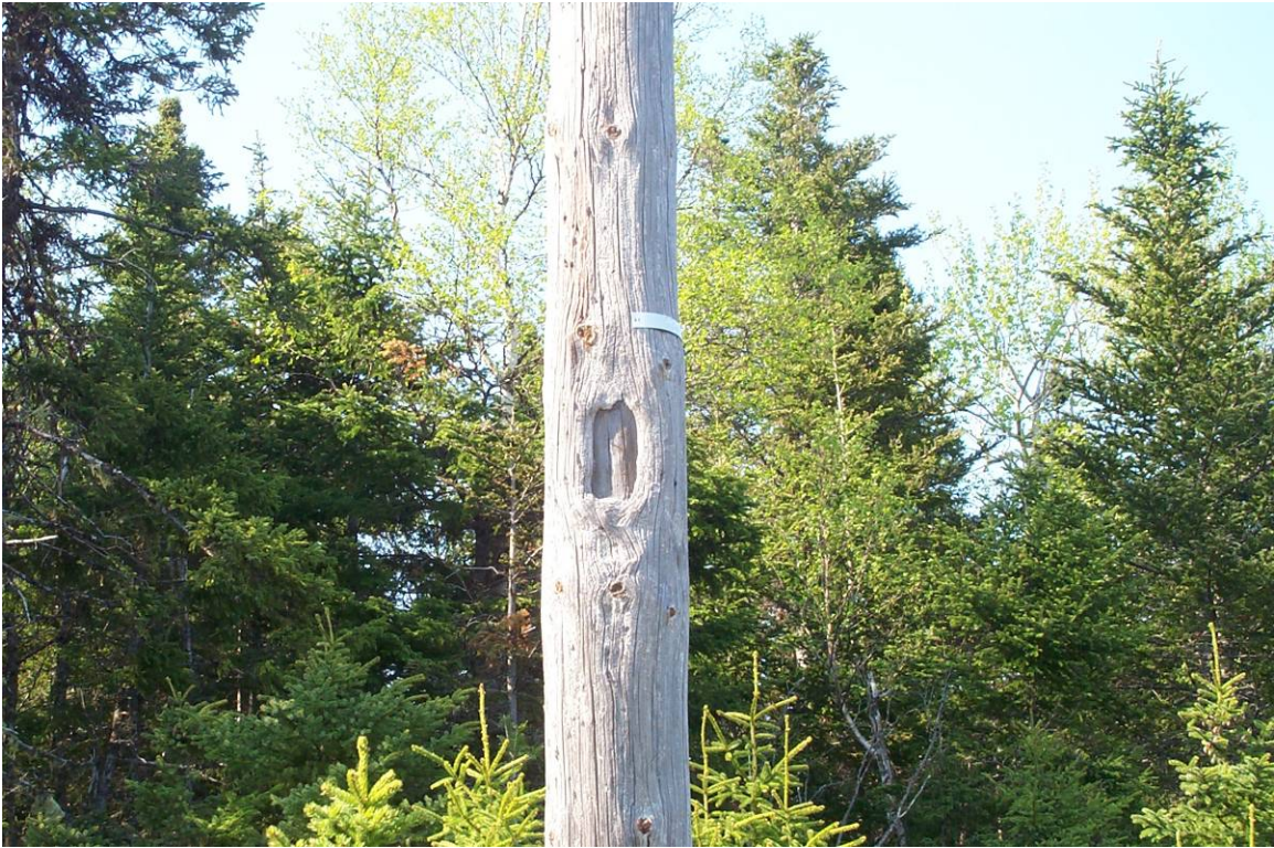
Figure 3 - Deteriorated pole 110L
