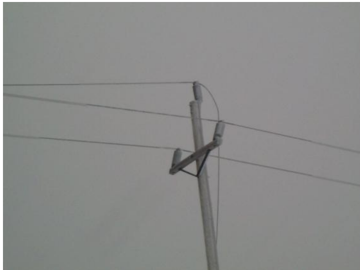
110L Broken Conductor - Ice Build Up December, 2003
