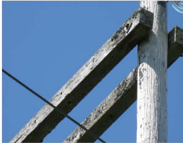
Deteriorated Crossarm
