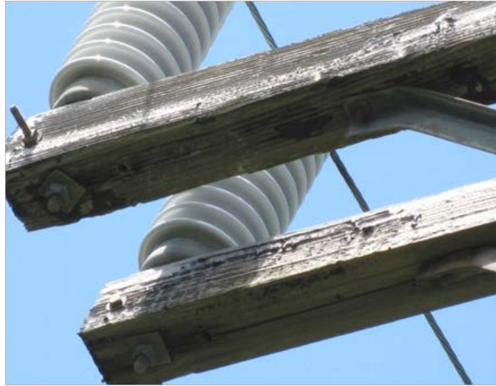
Deteriorated Crossarm
