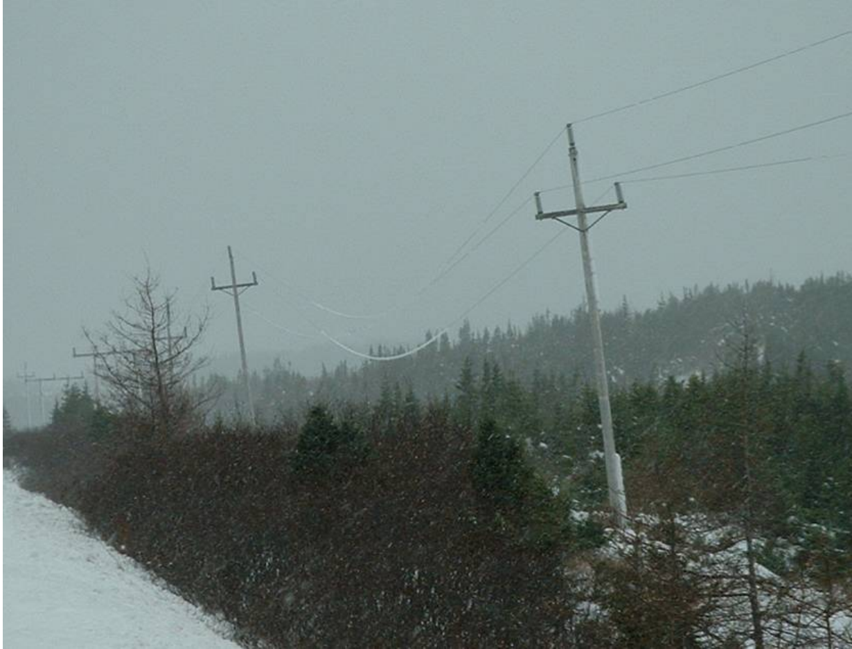
Figure 10 - 111L Ice Storm Damage December 2007
