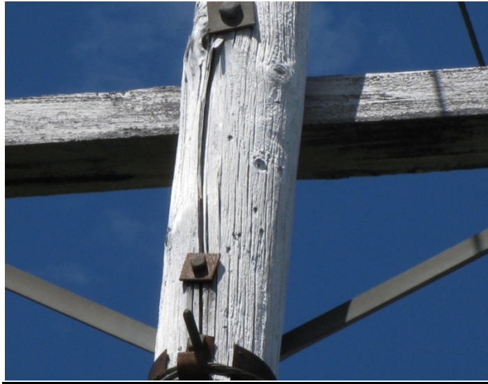
Pole Crack between Bolts
