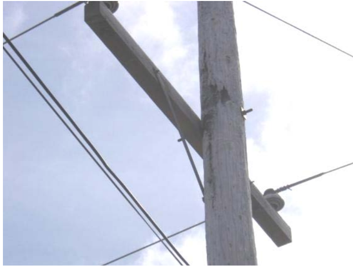
Burn Marks on Pole Caused by Flashover
