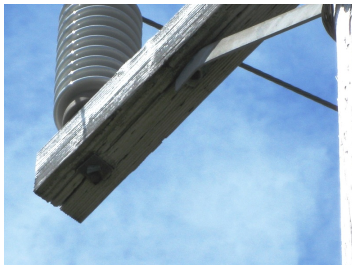
Deteriorated Crossarm
