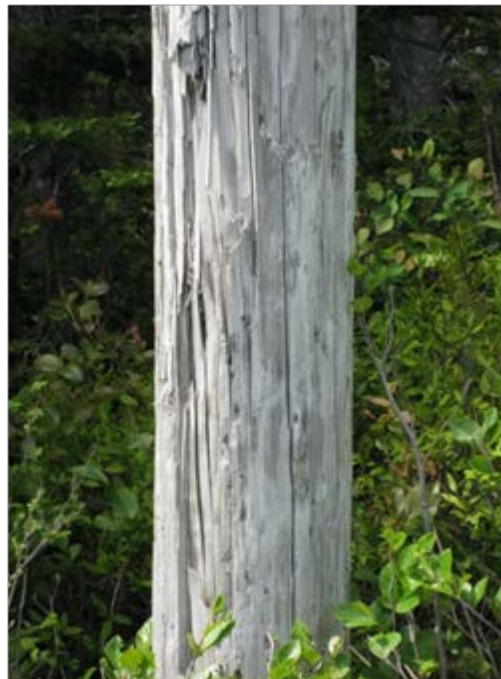
Deteriorated Pole
