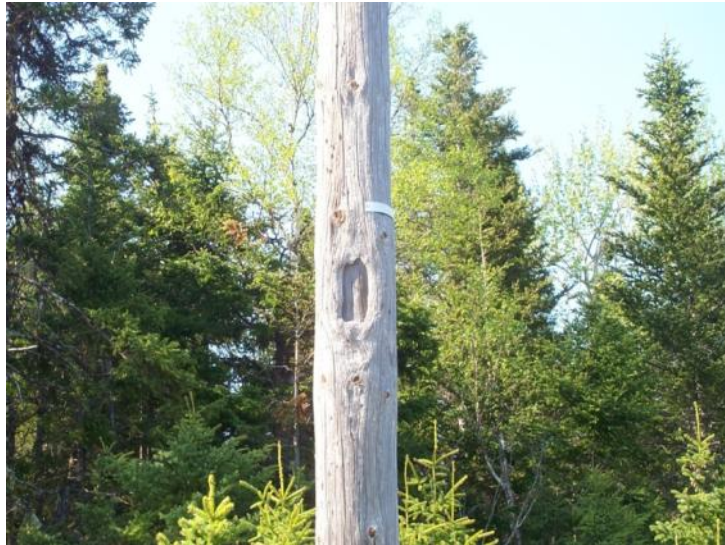
Deteriorated Pole 110L
