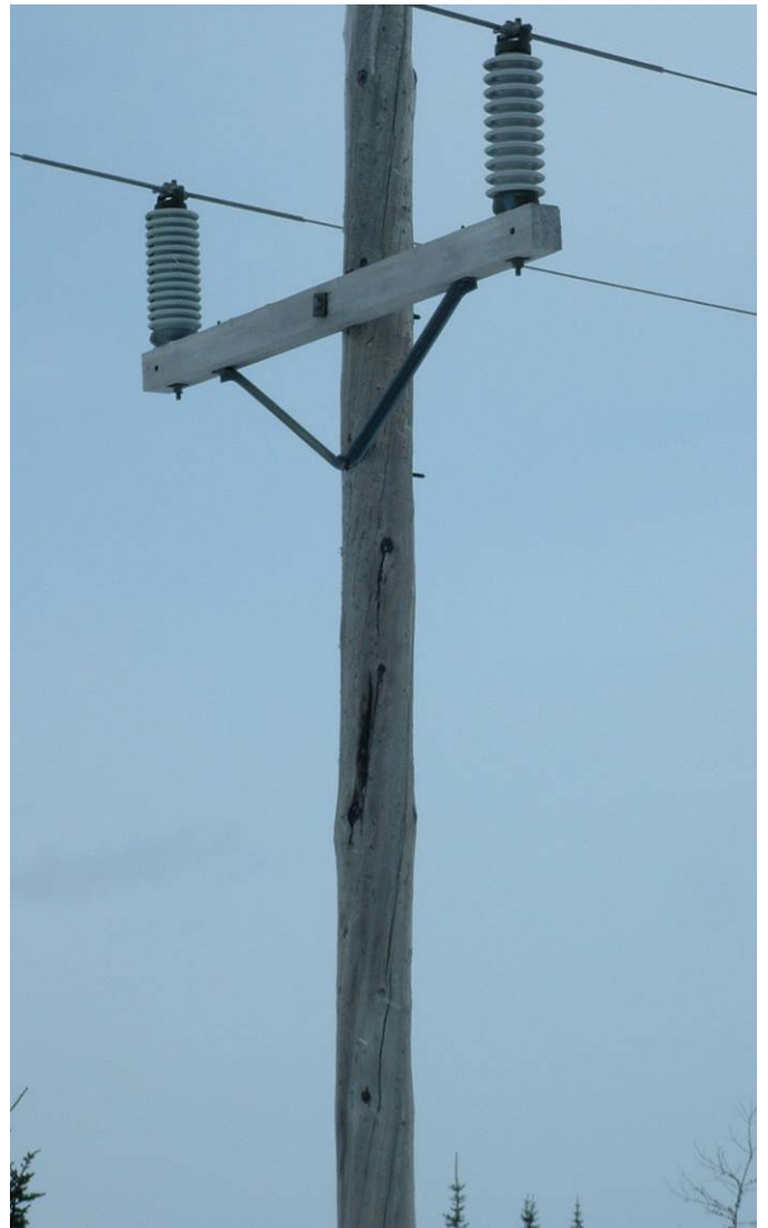
Figure 6 - Deteriorated Pole 111L
