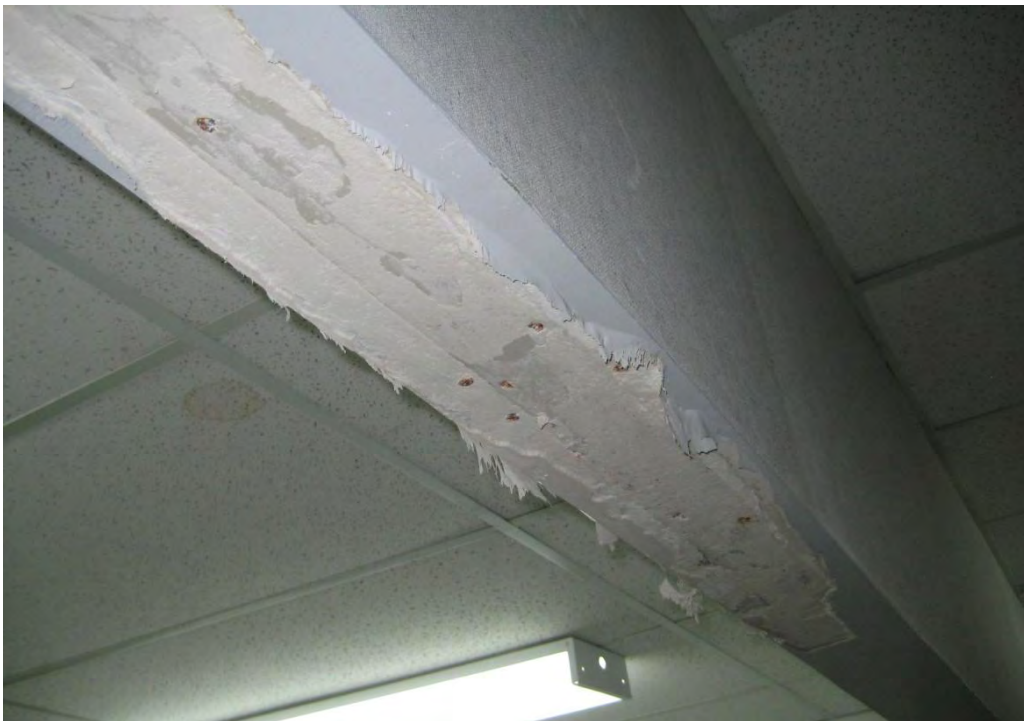
Figure 6 - Water Damage (2009)
