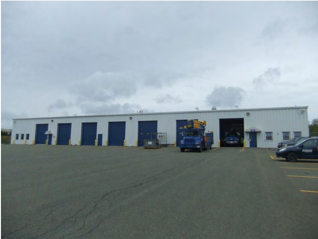
Figure 22 - Vehicle/Mechanical Maintenance, Exterior (2010)
