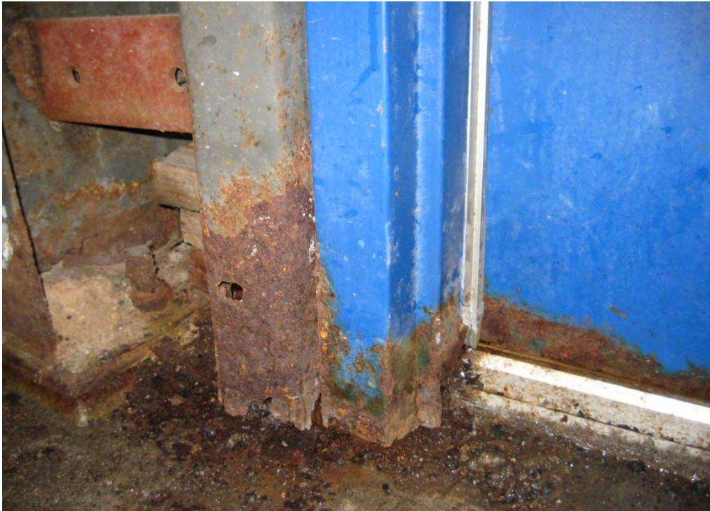
Figure 14 - Door Corrosion (2009)
