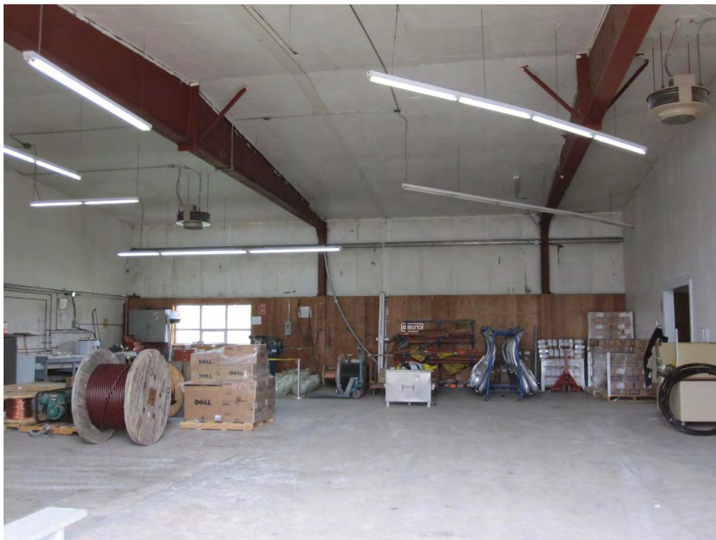
Figure 4 - Service Bay Interior (2010)
