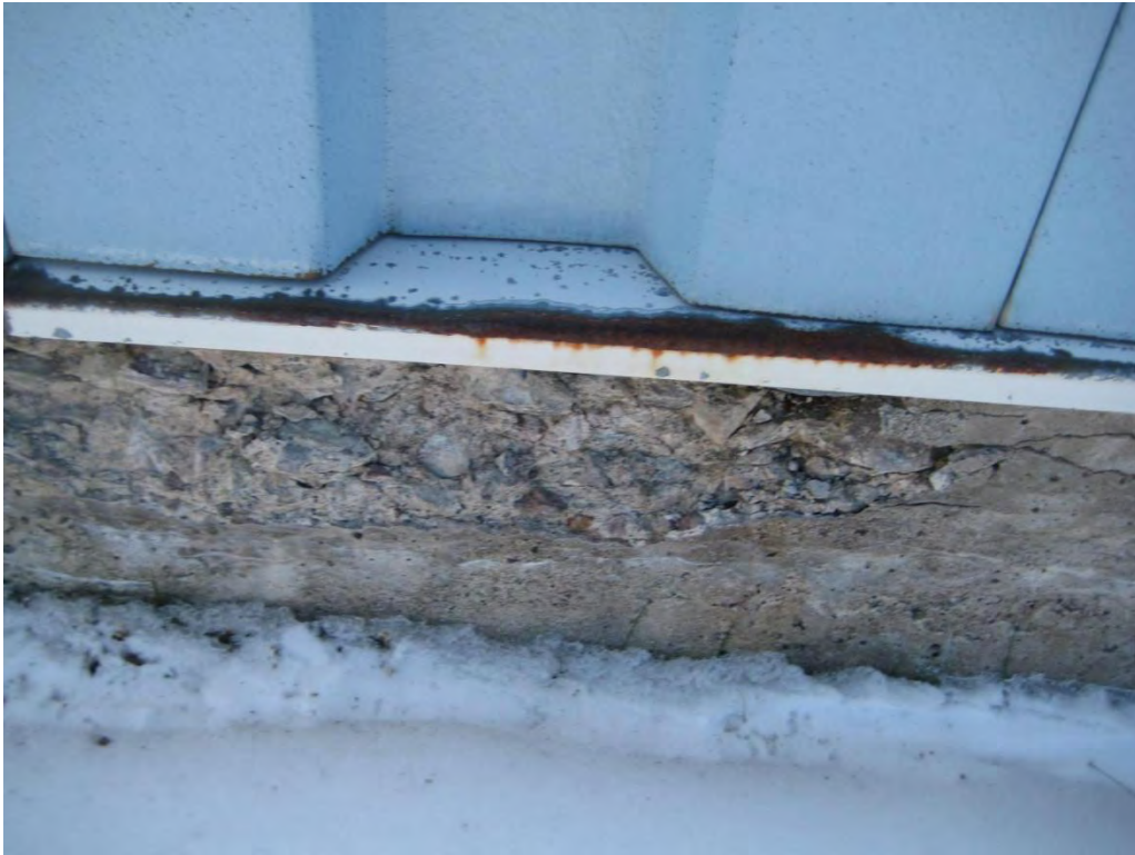
Figure 17 - Damaged Foundation (2009)
