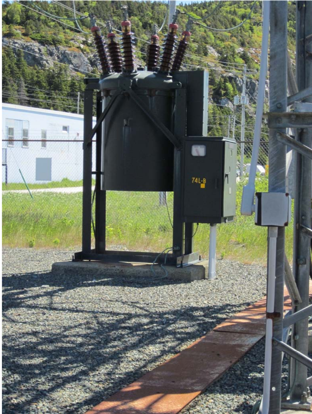
Pepperell Substation Circuit Breaker
