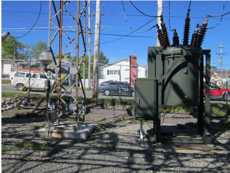
Stamps Lane Substation Oil Circuit Breaker
