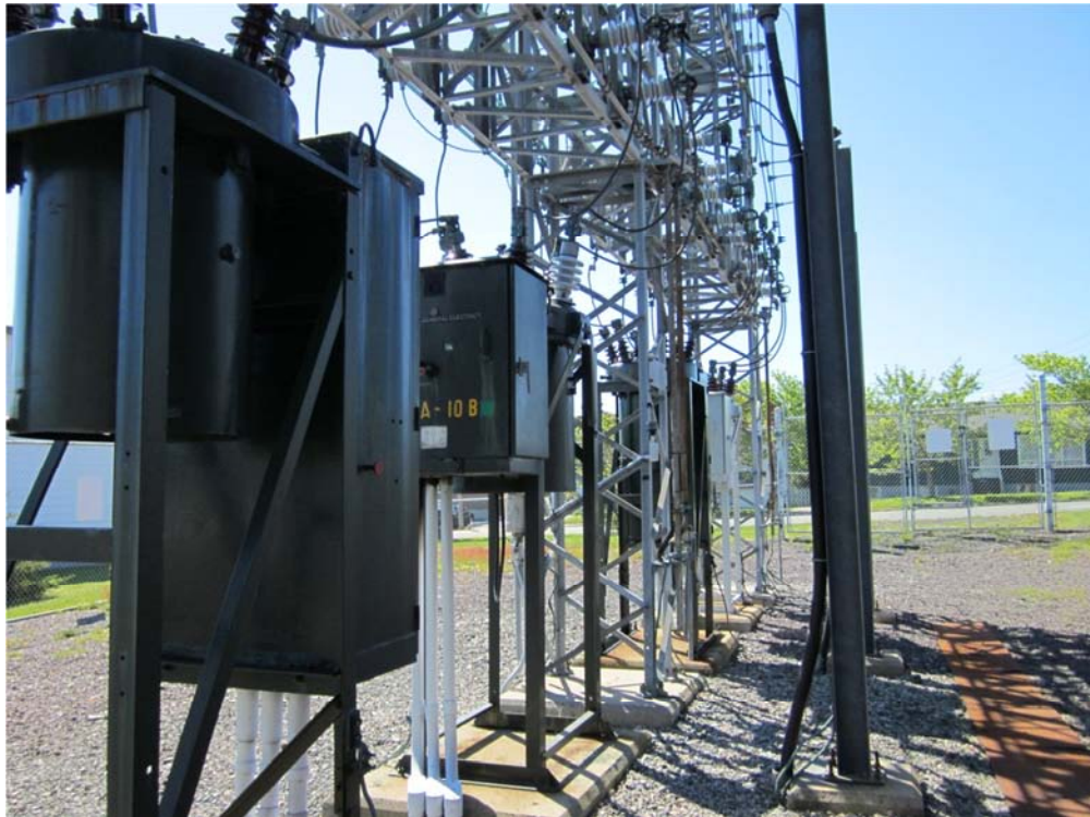
Stamps Lane Substation Circuit Breakers
