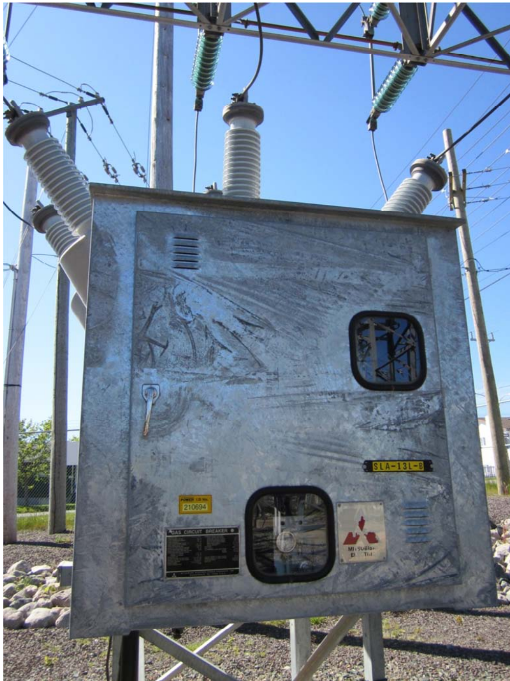
Stamps Lane Substation Circuit Breaker
