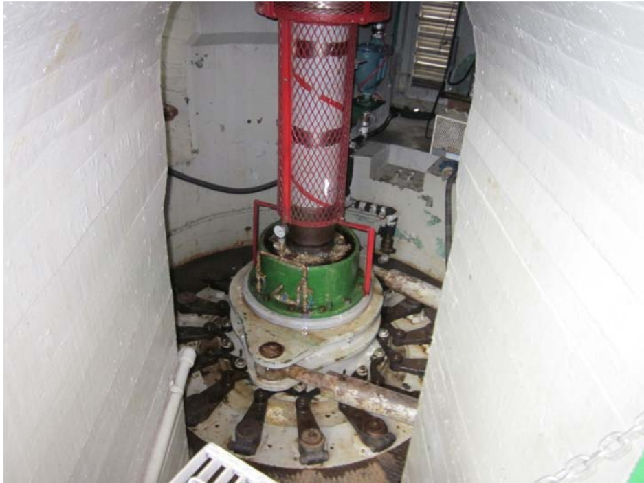
Rocky Pond Hydro Turbine Shaft
