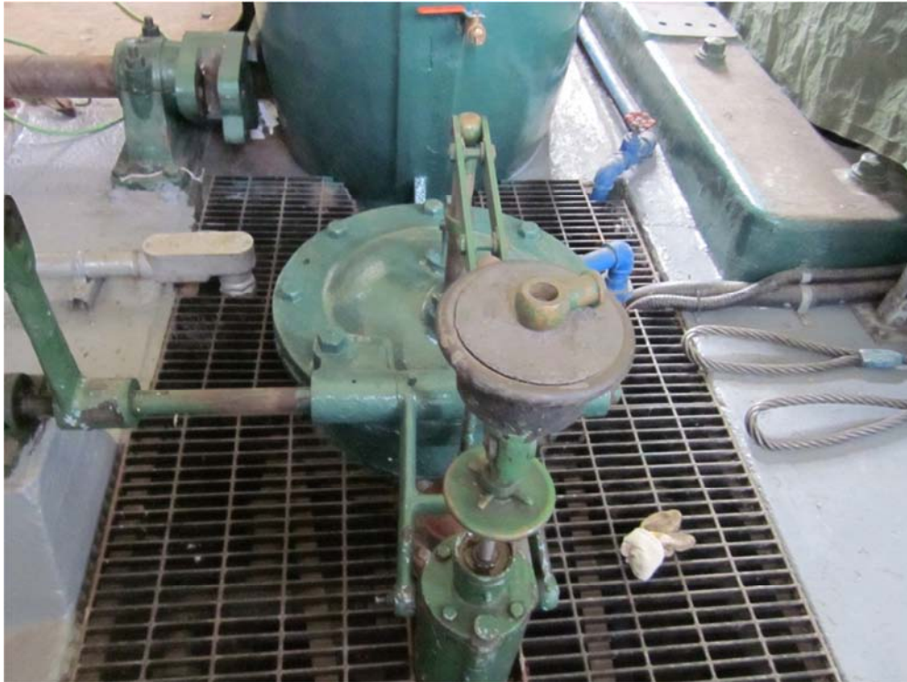
Seal Cove Hydro Plant Pressure Relief Valve
