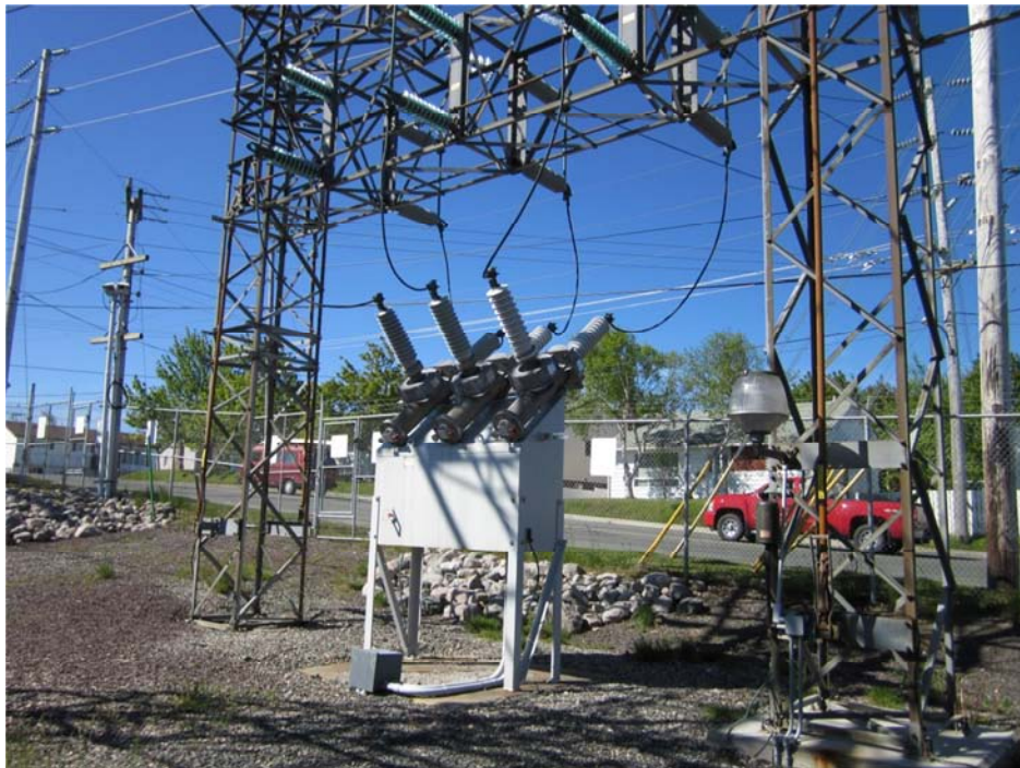
Stamps Lane Substation SF6 Gas Circuit Breaker
