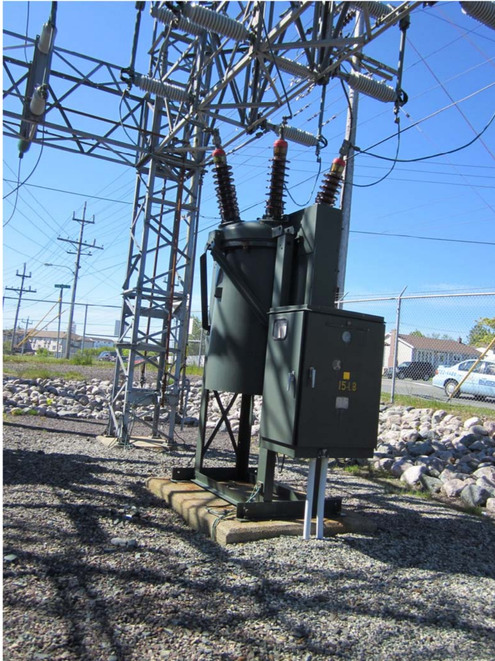
Stamps Lane Substation Circuit Breaker
