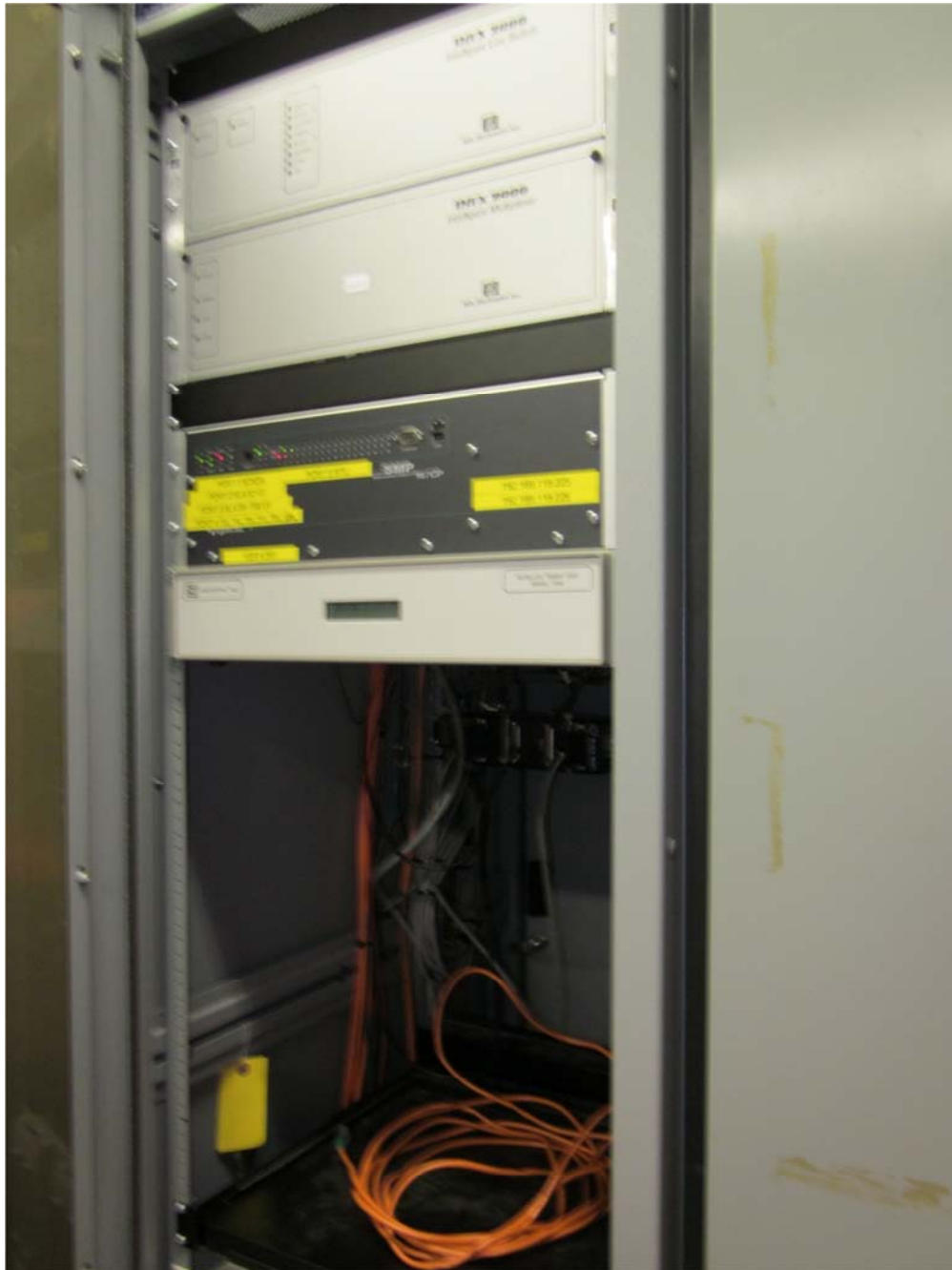
Stamps Lane Substation Fiber Optic Equipment
