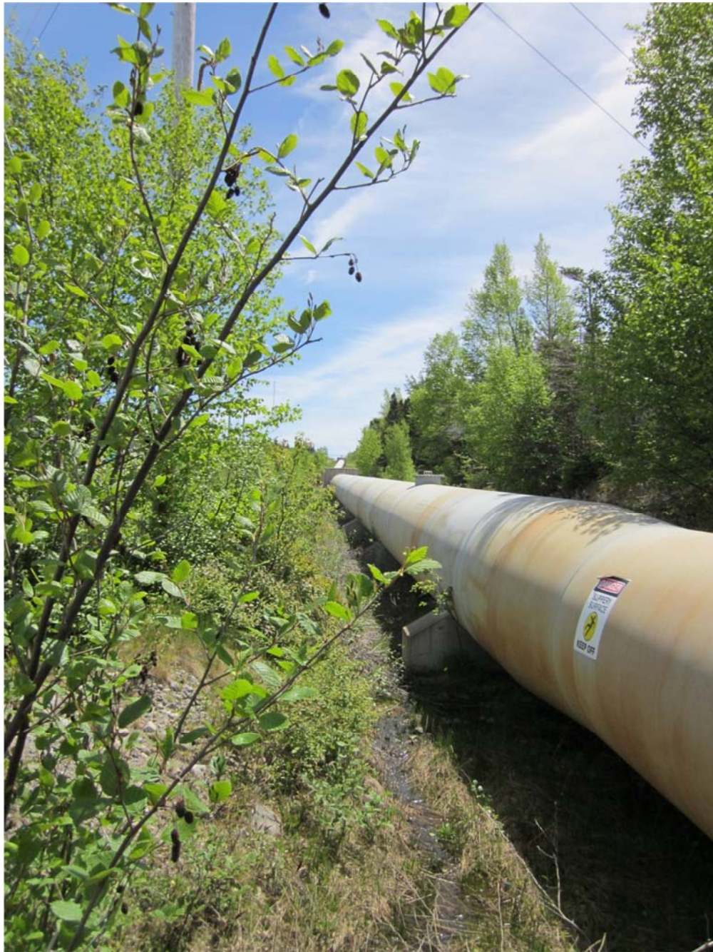
Seal Cove Hydro Plant Penstock
