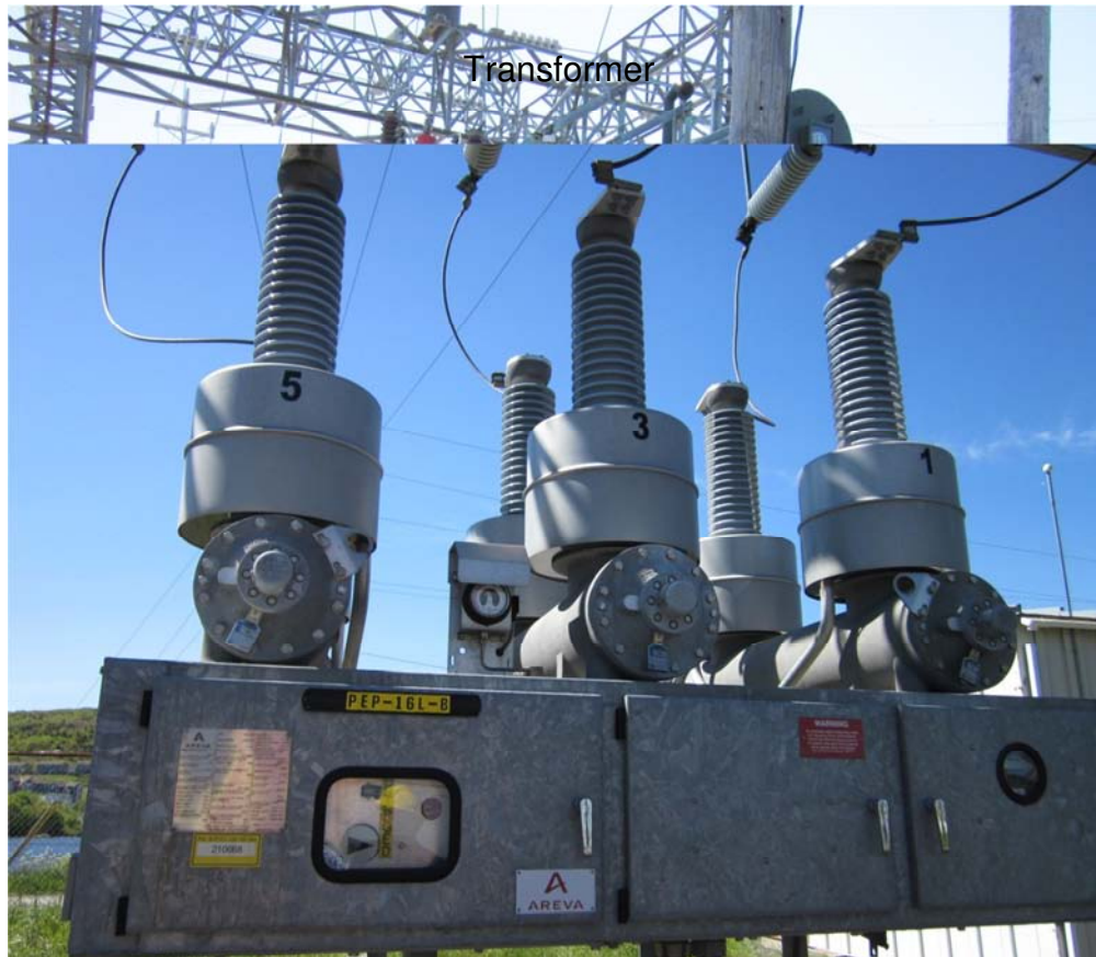
Pepperell Substation Circuit Breaker
