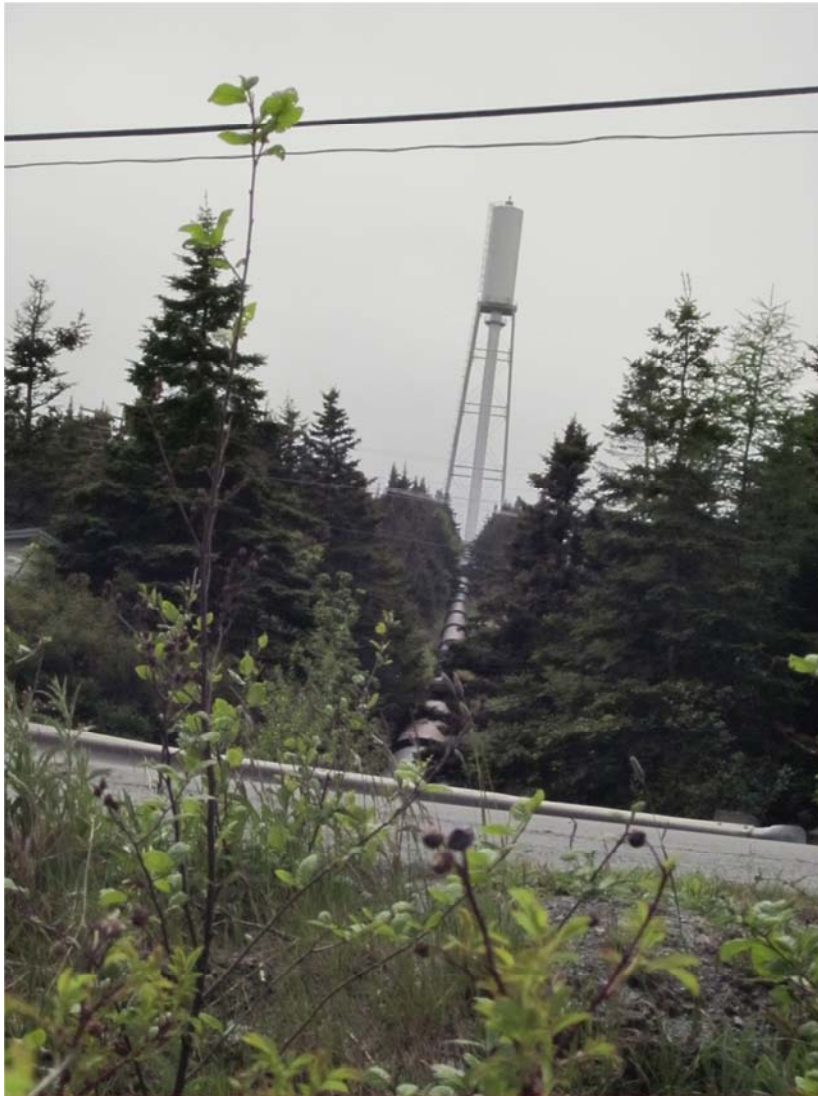
Mobile Hydro Penstock and Surge Tank
