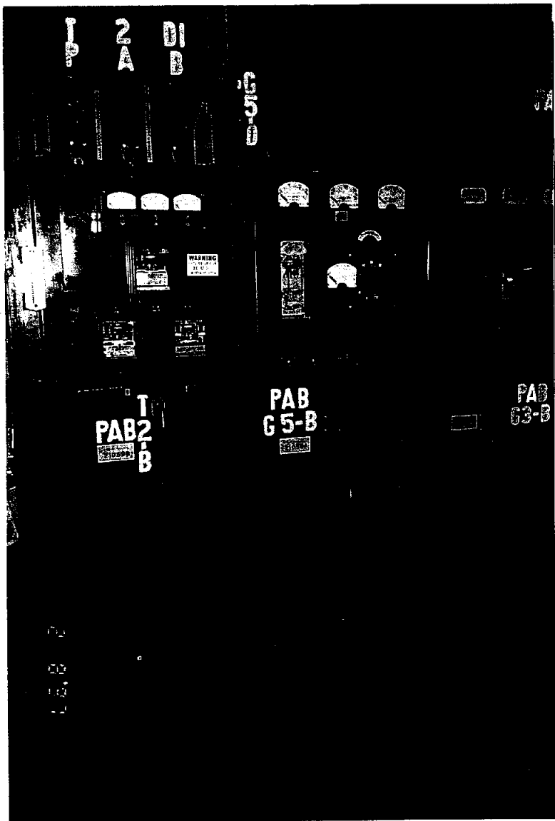
Photo 51 Port-aux-Basques - Outdated switchgear
