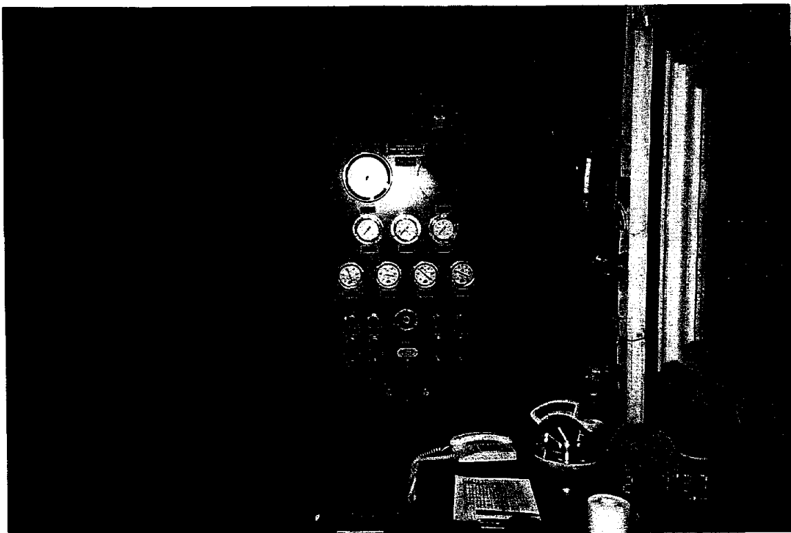
Photo 40 Aguathuna - Engine instrument panel in control room
