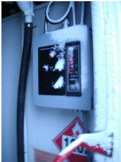
Snow covering electrical equipment in mobile unit
