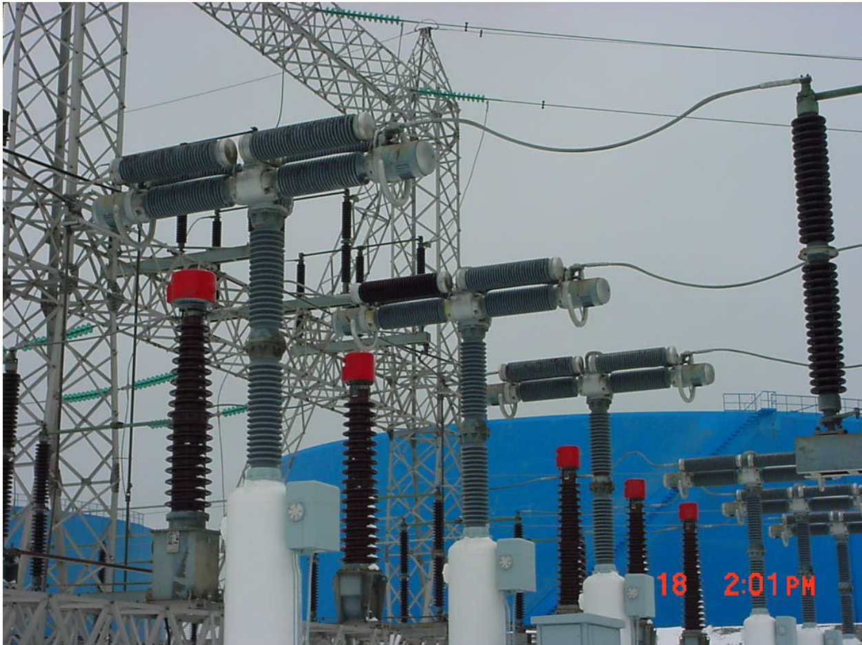
Figure 1: 230 kV Air Blast Circuit Breaker in the HRD TS - DLF Asea Brown Broveri (ABB)
