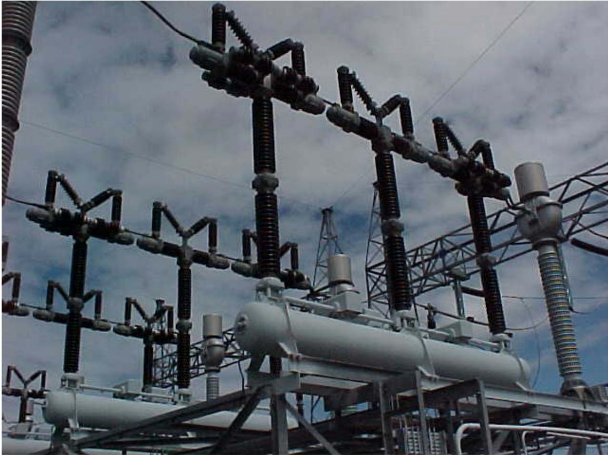
230 kV Breaker – DCVF in terminal station
