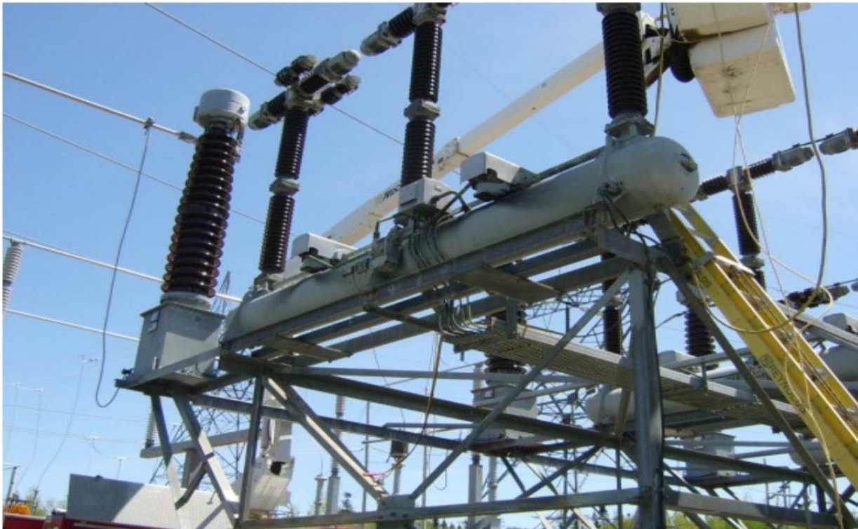
230 kV Breaker – DCVF during overhaul
