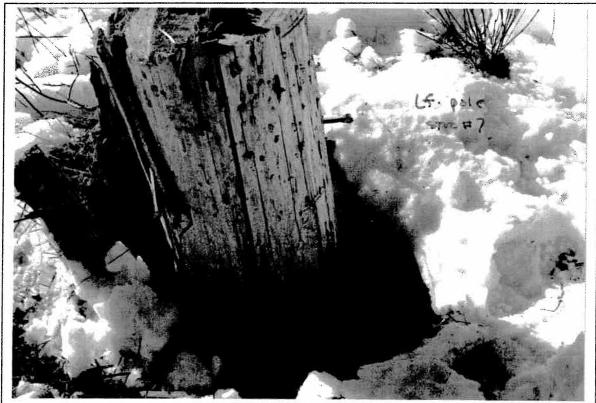
Photo 8: TL201 - Str.#7 - Type A Left pole moved through ground.
