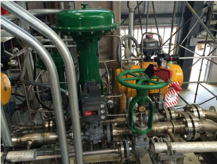
Photo 2: Fuel bypass valve locked and tagged
