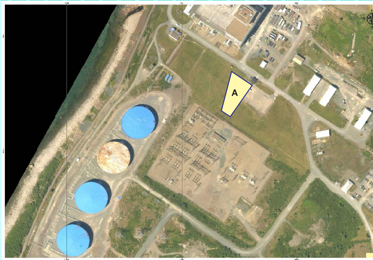
Figure 1. Location of Generator Solution
