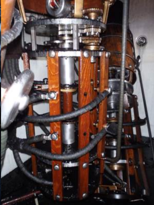
Photo 12 – LTC Compartment (Phases 2 & 1)
