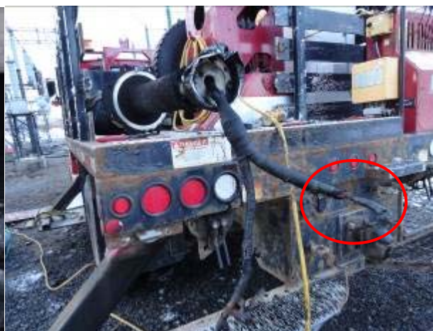
Photo 22 – LV1 Bushing Lead Broken at the Crimp
