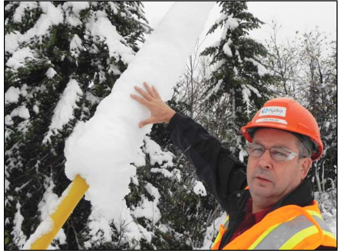
Joe Walsh, Line Superintendent for the Central Region, stands next to a de-energized line on the Baie Verte Peninsula. Up to nine inches of ice stuck to the power lines in the area during a snow and ice storm.
