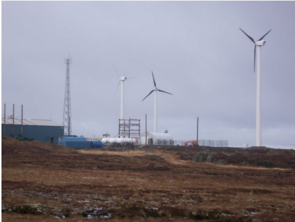
Overall Project Site showing (L-R): diesel plant/storage tanks, meteorological tower, hydrogen electrolyser, three hydrogen storage tanks, distribution box structure, three wind turbines, and Quonset hut housing the hydrogen genset.
