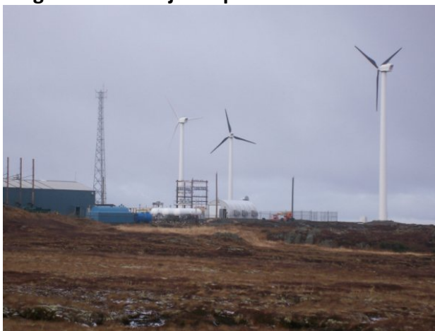
Overall Project Site Showing (l-r) the Diesel Plant/Storage Tanks, Meteorological Tower, Hydrogen Electrolyser, 3 Hydrogen Storage Tanks, Distribution Box Structure, 3 Wind Turbines, and Quonset Hut Housing the Hydrogen Genset.
