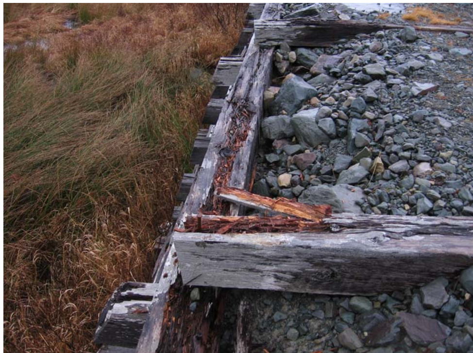
Figure 6 Extensive wood rot evident on timbers (Photo taken prior to 2006 rehabilitation)
