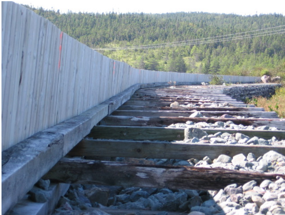
Figure 4 Cribbing prior to 2006 rehabilitation showing extent of deterioration of wood structure
