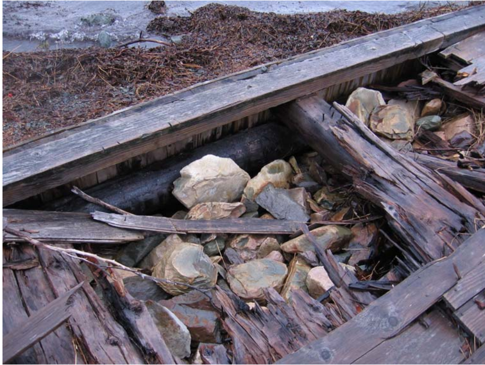
Figure 5 Where dam face meets cribbing (Photo taken prior to 2006 rehabilitation)
