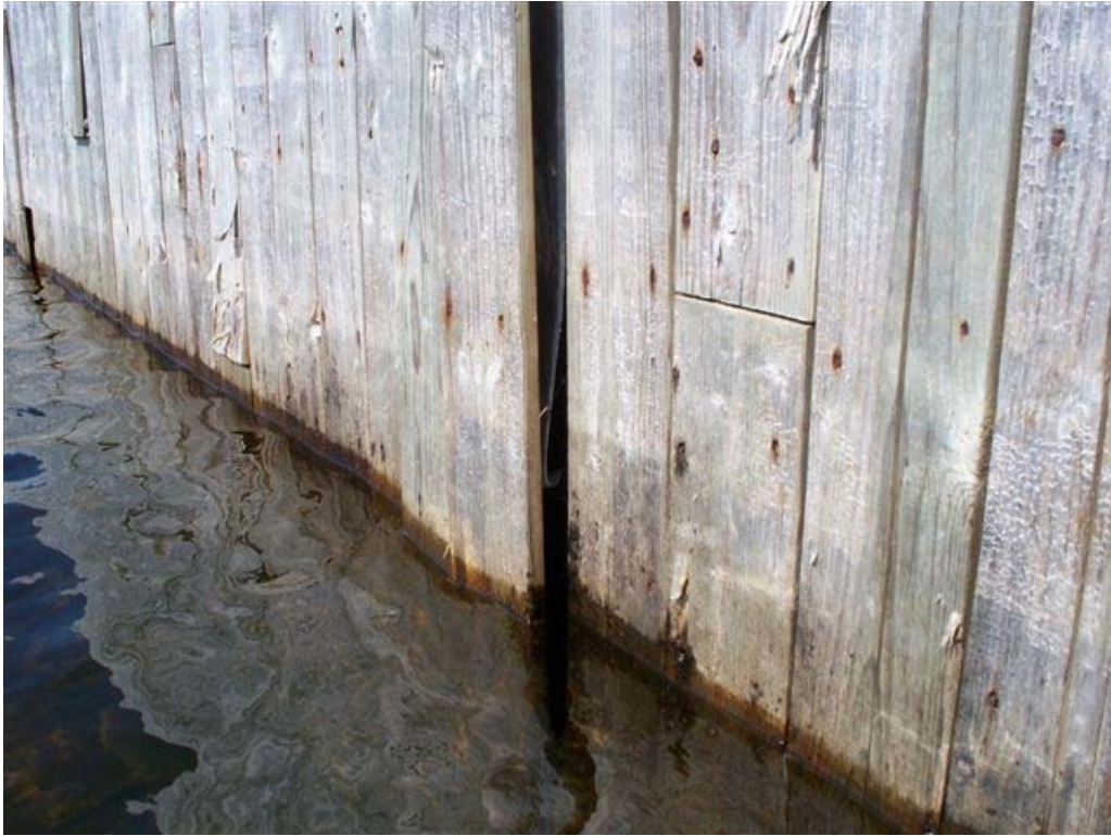
Figure 3 2010 picture showing face board separated from timber cribbing
