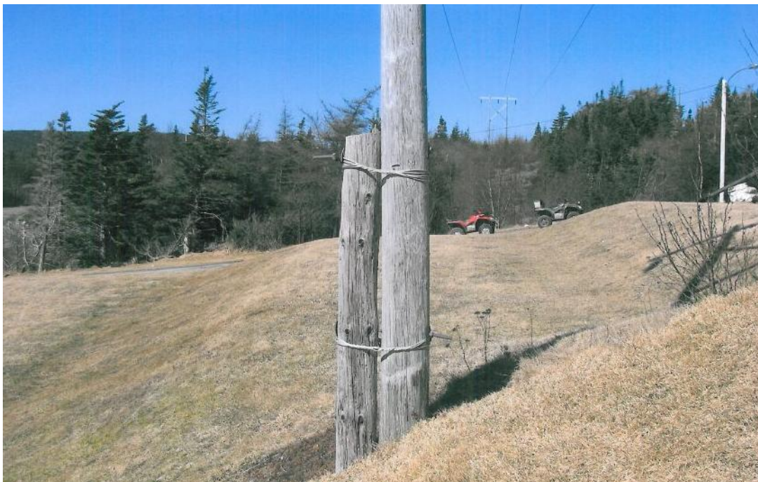
Figure 6 – Pole requiring temporary support 21L
