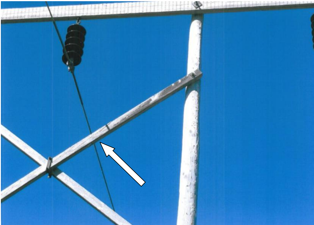
Figure 5 – Split crossbrace 21L
