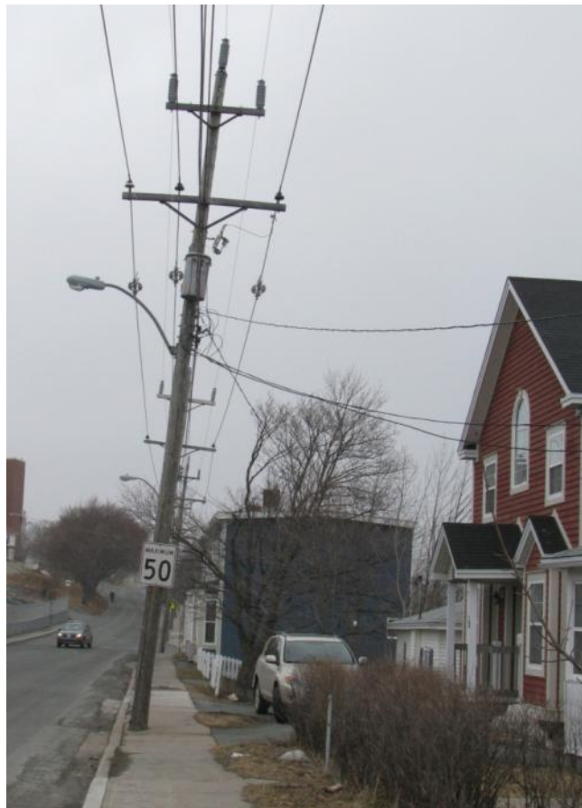
Figure 2 – Poles leaning along the Boulevard 16L
