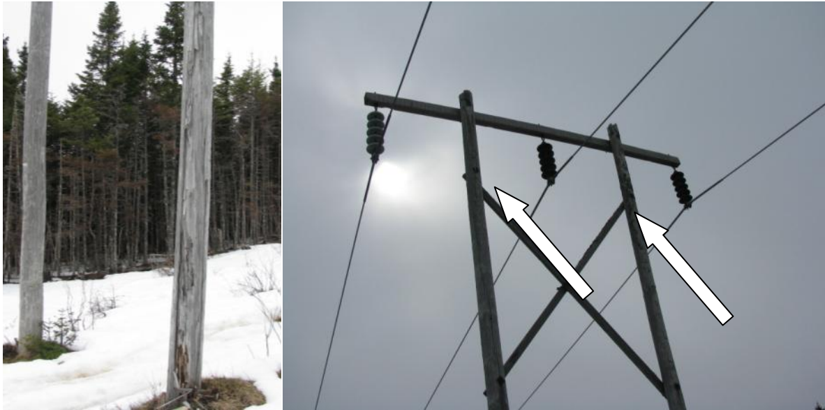
Figure 15 – Rotten poles 25L
