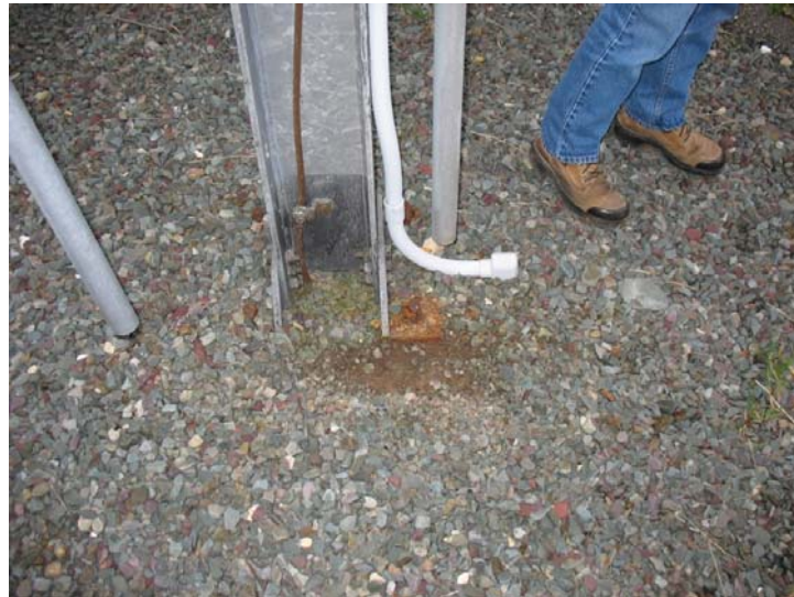
Severe Rusting On Anchor Bolt
