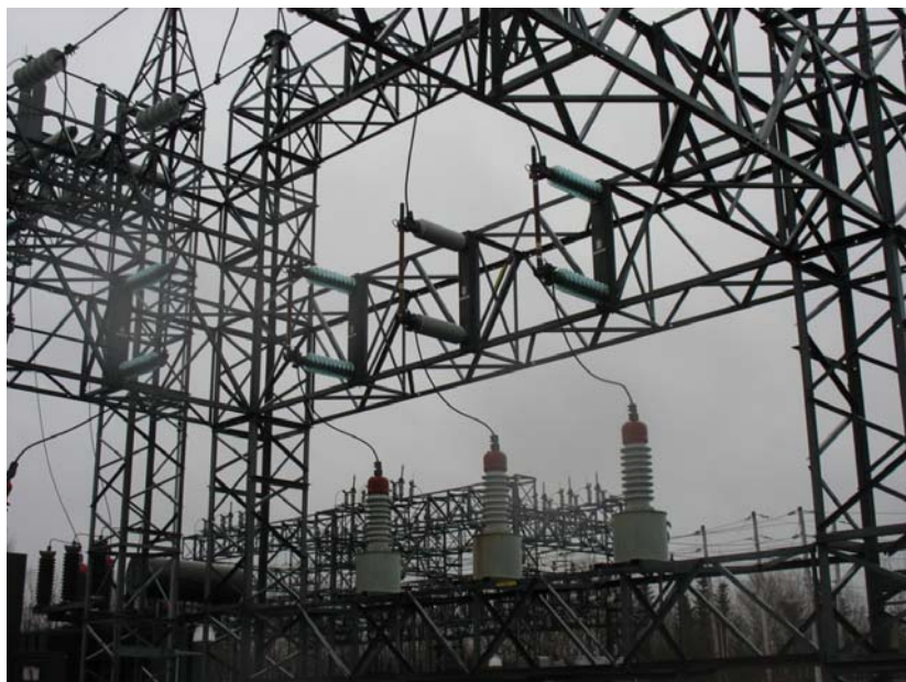
66 kV potential Transformers
