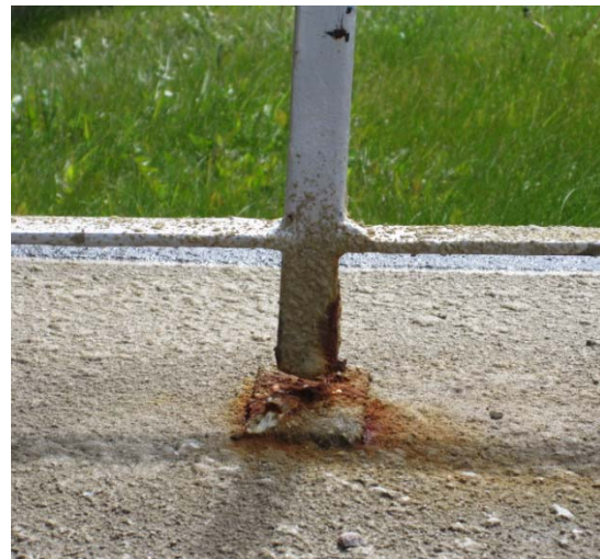
Figure 4 – Completely corroded railing support post.
