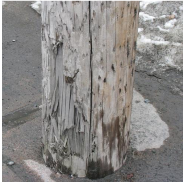
Figure 1 – Pole damaged by vehicle 16L
