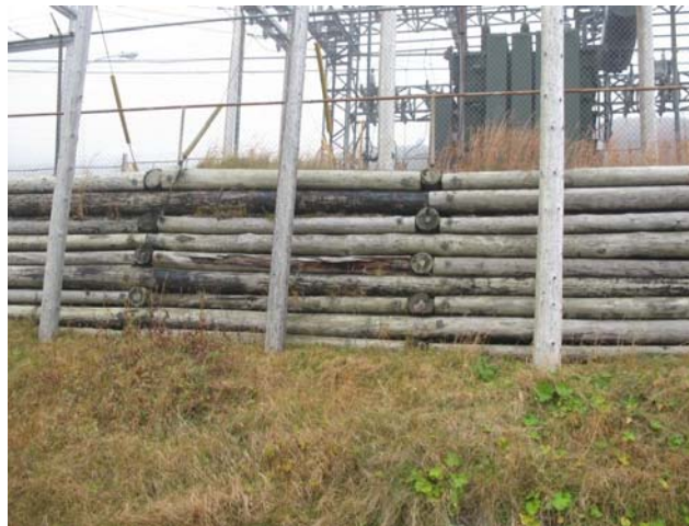
Deteriorated Retaining Wall
