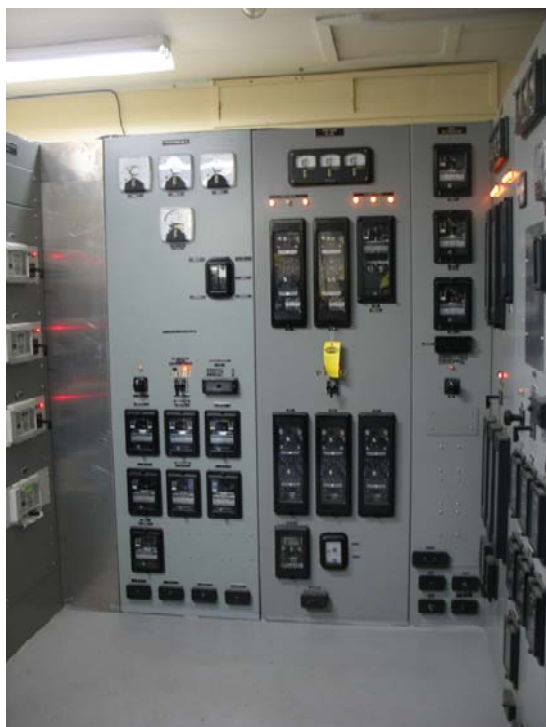
Transmission Line Electro Mechanical Relays
