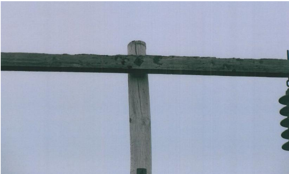
Figure 12 – Deteriorated pole and crossarm 21L
