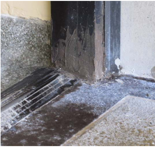
Figure 1 – Repairs to corroded door frame.
