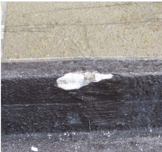
Figure 3 – Annual chipping and cracks from deteriorated underlying concrete.
