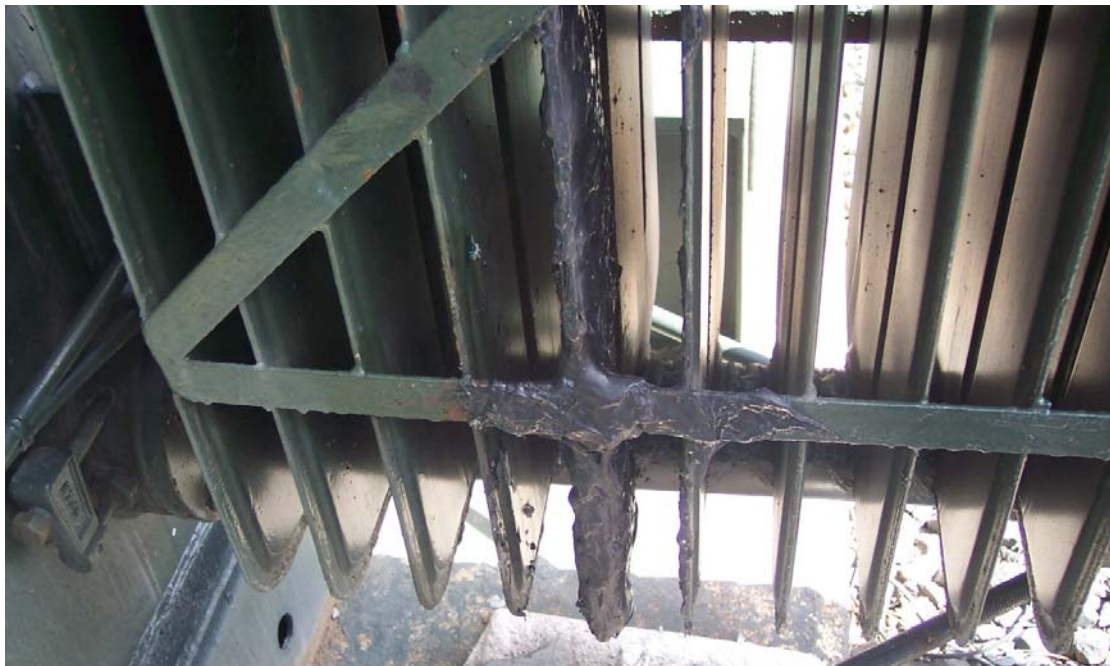
Patched Radiator on SLA-T2
