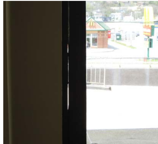
Figure 2 – Air gap between door and frame.
