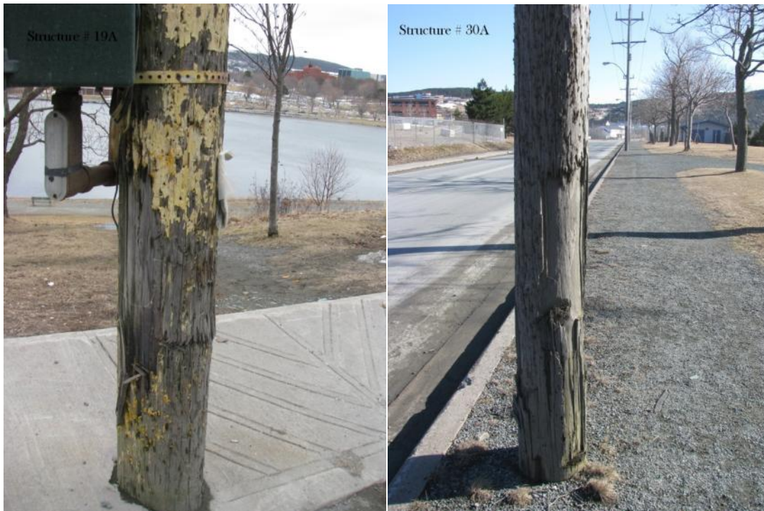
Figure 3 – Deteriorated poles 16L
