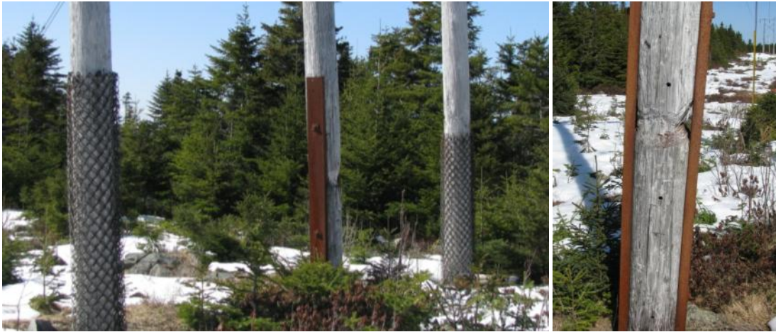
Figure 13 – Damaged pole requiring external support 25L
