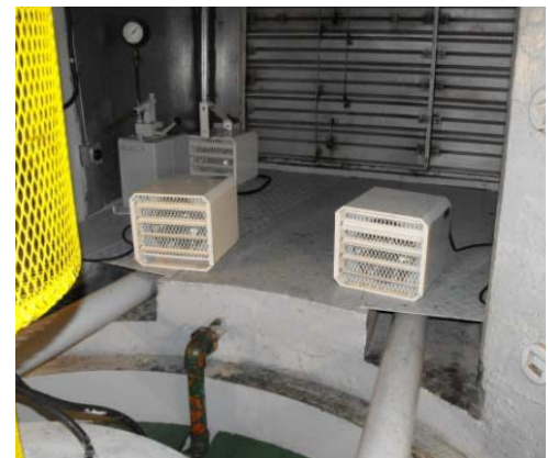
Figure 7 - Anti-condensation Heaters
