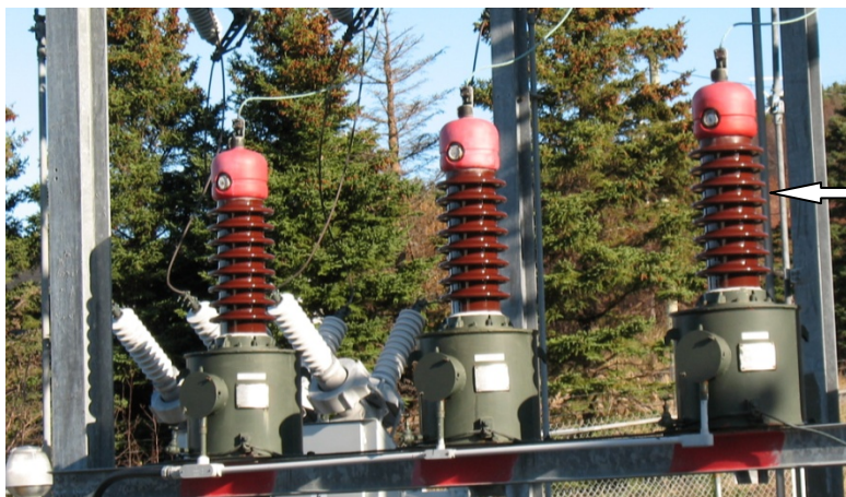
Figure 3 - 66 kV Potential Transformers
