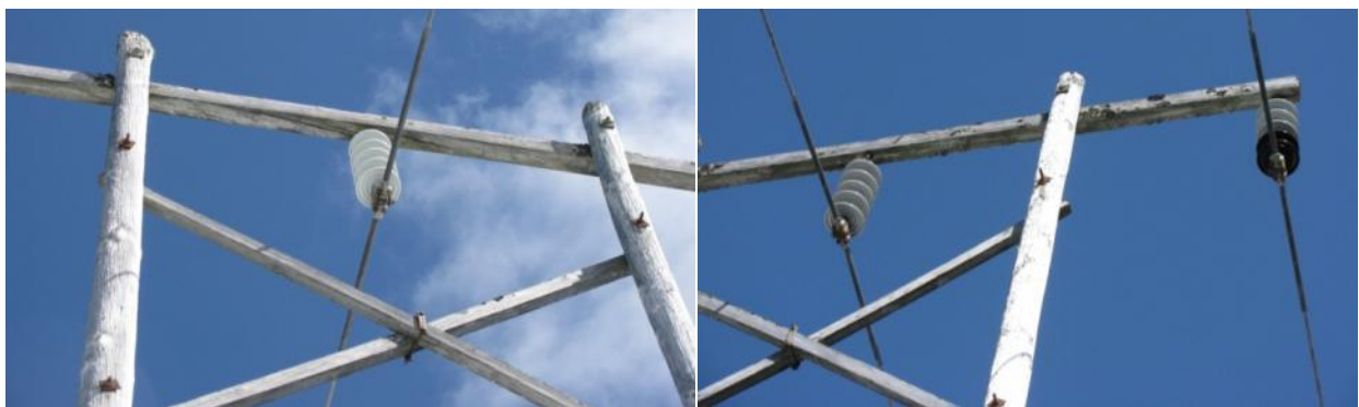
Figure 18 – Deteriorated poles, crossarms and hardware 25L
