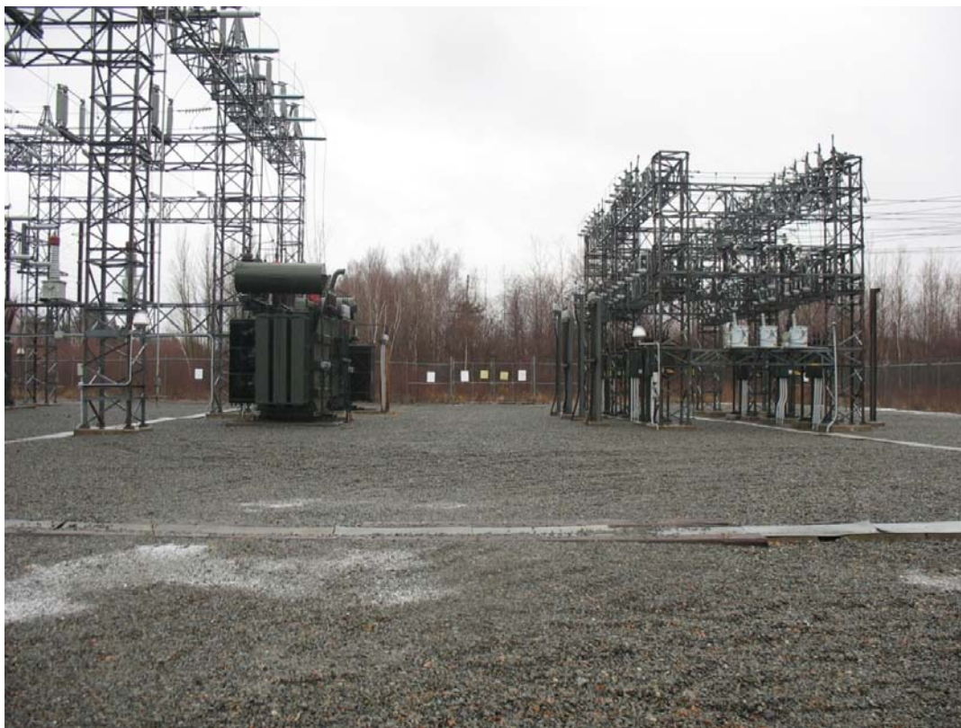
138kV & 25 kV Steel Structures & Bus
