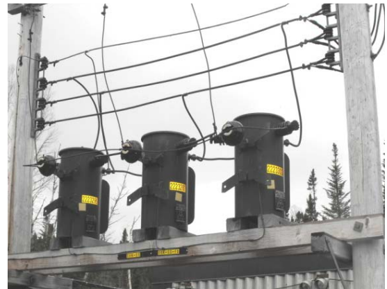
Figure 4 - Station Service Transformers
