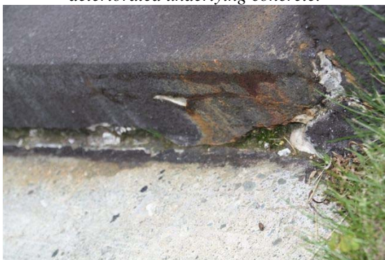
Figure 5 – Deteriorated concrete step.
