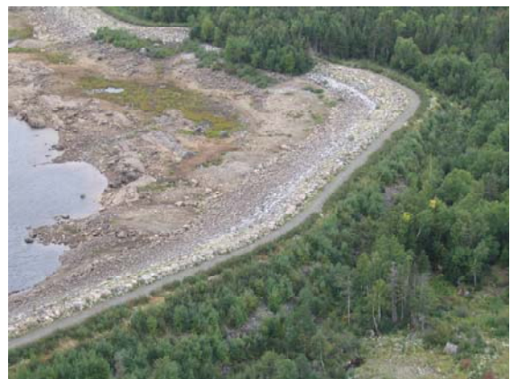
Figure 3 - Rattling Lake Dam (Note excessive vegetation on downstream face)
