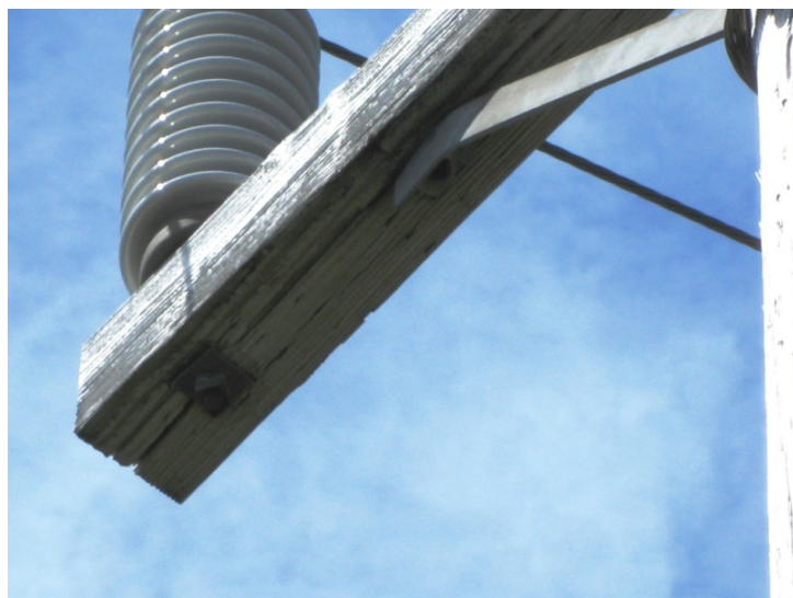
Deteriorated Crossarm
