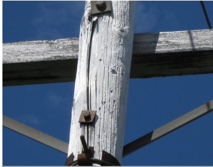
Pole Crack between Bolts
