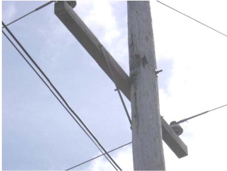
Burn Marks on Pole Caused by Flashover
