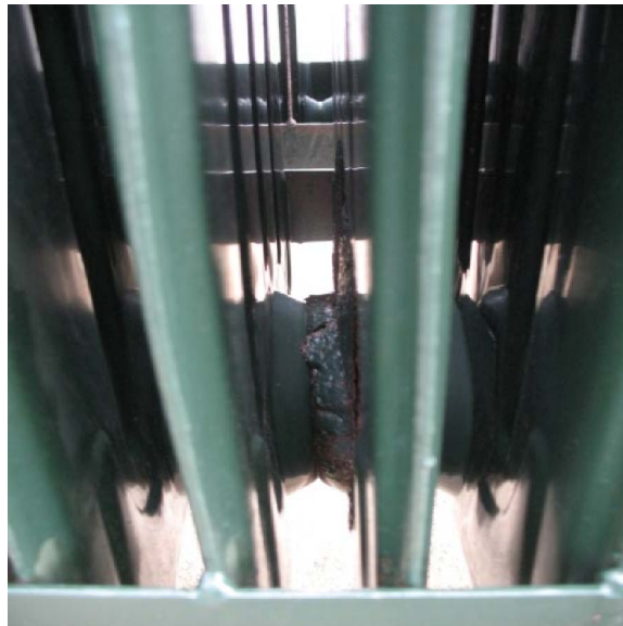
Gillams Transformer Radiator Deterioration
