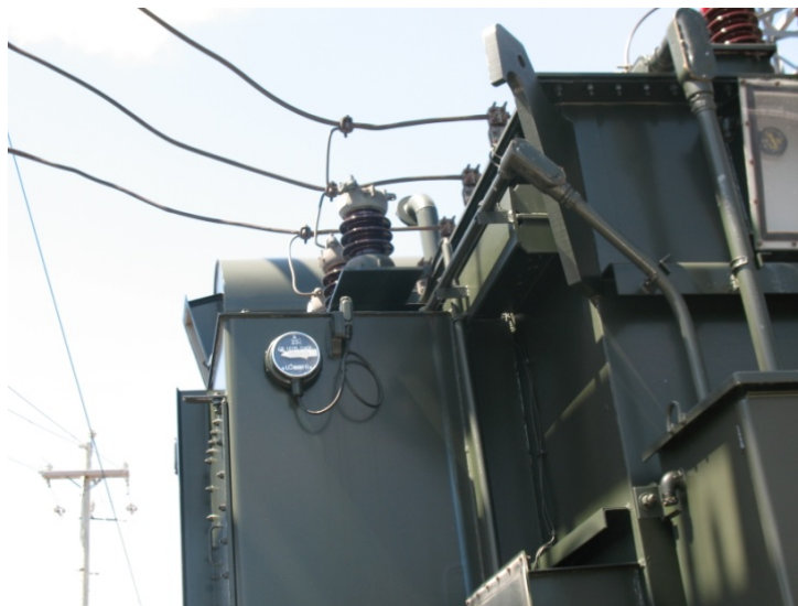
WES-T1 Low Voltage Lightning Arrestors
