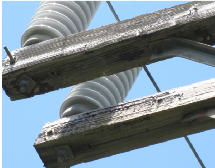
Deteriorated Crossarm
