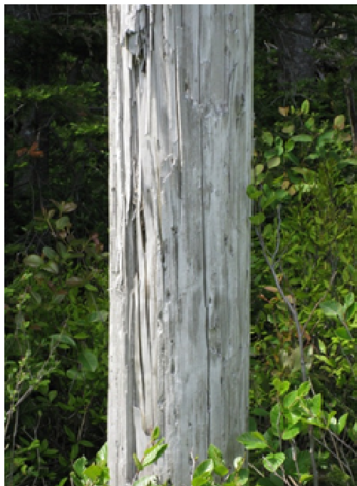
Deteriorated Pole
