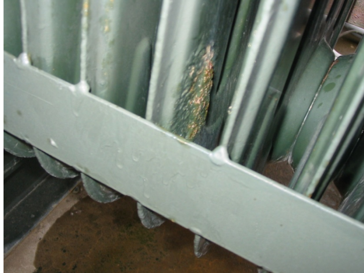
Deteriorated Radiator
