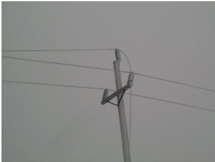
110L Broken Conductor - Ice Build Up December, 2003
