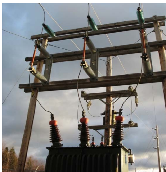
Station Service Transformer Structure
