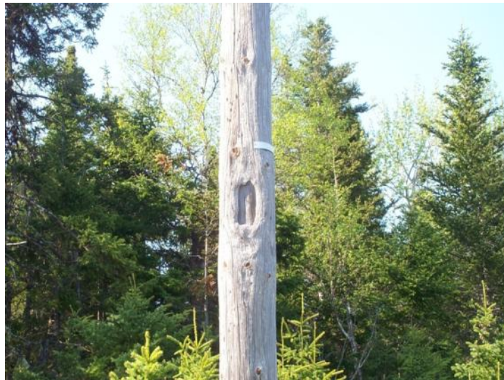
Deteriorated Pole 110L
