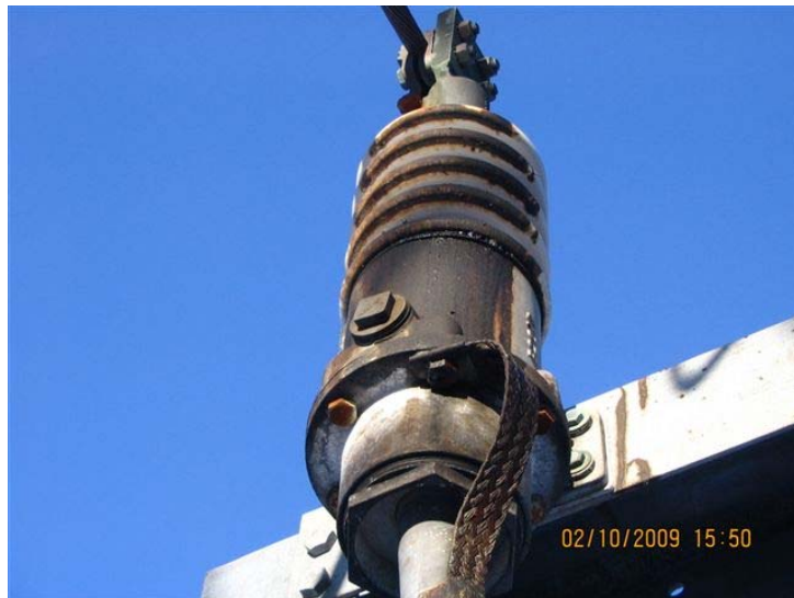
Leaking 12.5 kV Potheads
