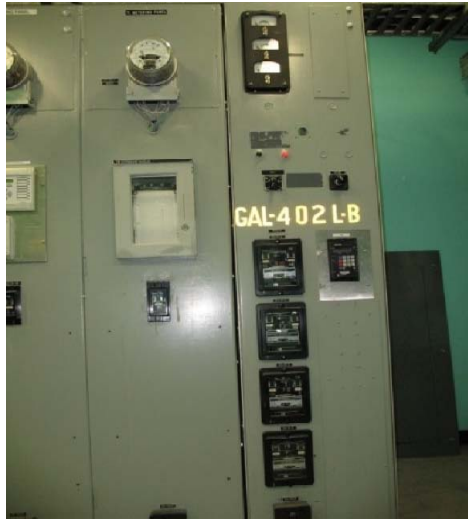
Transmission Line Protection Relays
