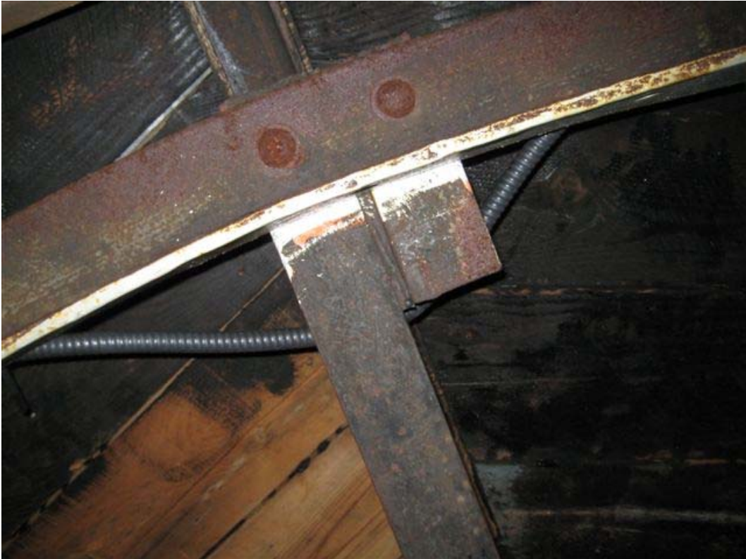
Roof Beam Connection to Outer Ring
