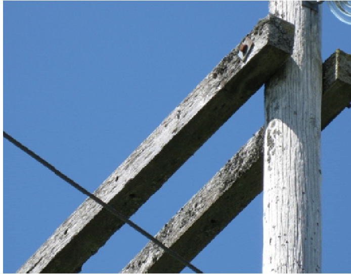
Deteriorated Crossarm
