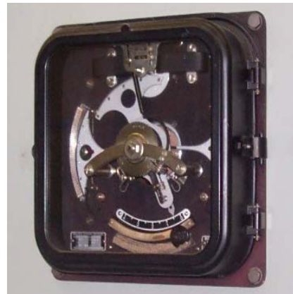
Figure 1 - BB Voltage Regulator
