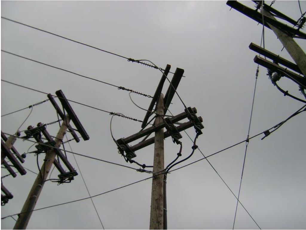
Figure 2: Inadequate structure clearance for increased voltage levels.
