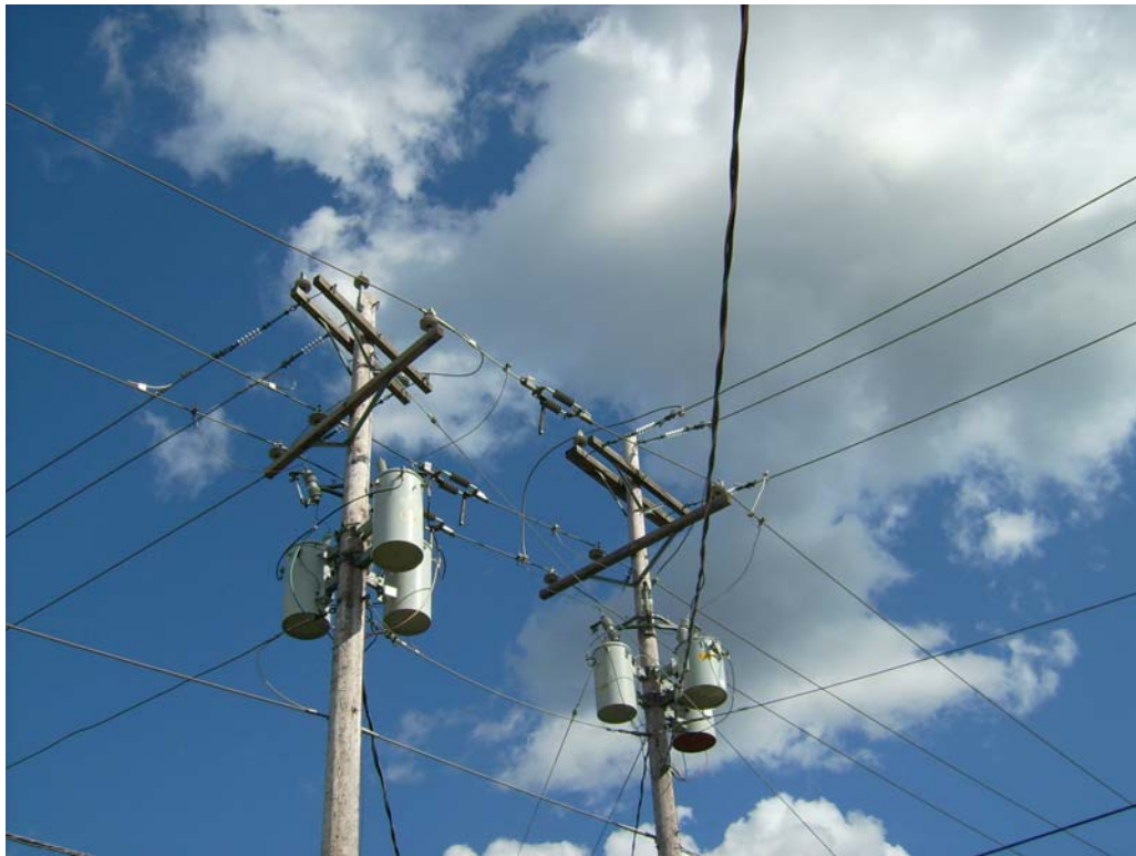
Figure 1: Existing poles are congested and overloaded.
