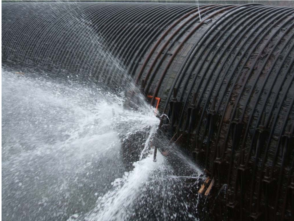
Figure 2 – Metal Patch Covering Area of March 8 Major Leak (Photo: August 12 th , 2008)
