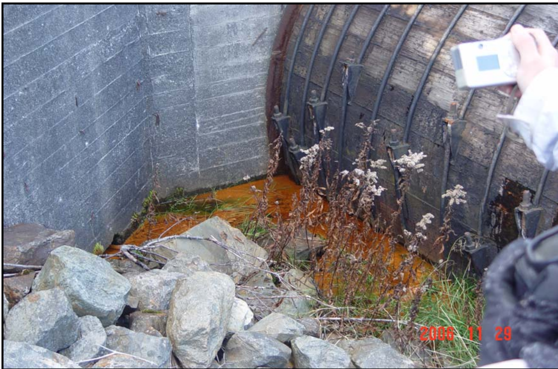
Photograph #14 – Poor drainage and ventilation near the intake conduit.
