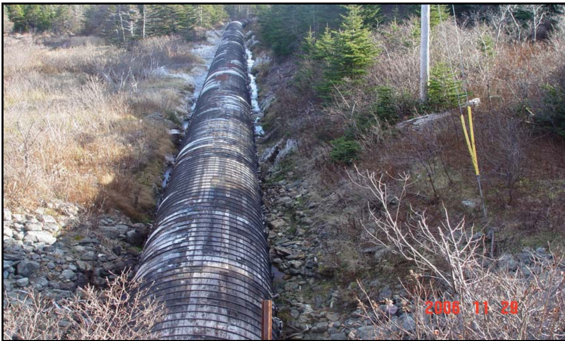
Photograph #15 – Looking downstream at the intake. Note creosote leached out by the sun.
