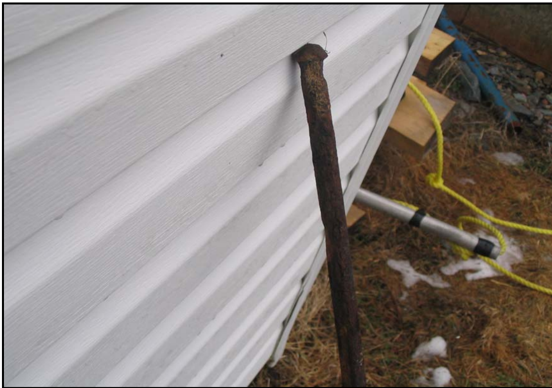
Photograph #27 – Typical corroded steel band button head.
