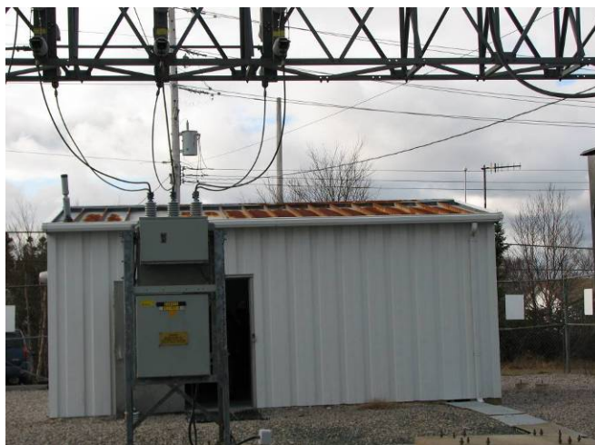
Control Building Roof Deterioration
