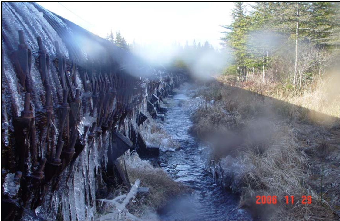
Photograph #19 – Extensive flows along the pipeline.
