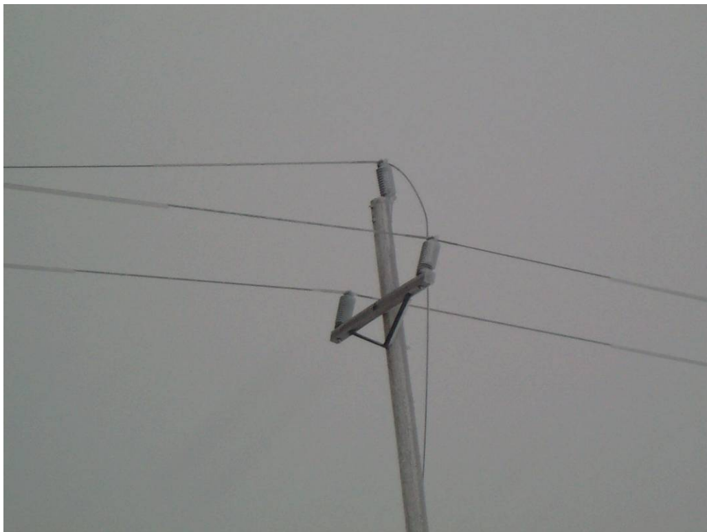
Figure 2 - 110L Broken conductor - ice build up December, 2003
