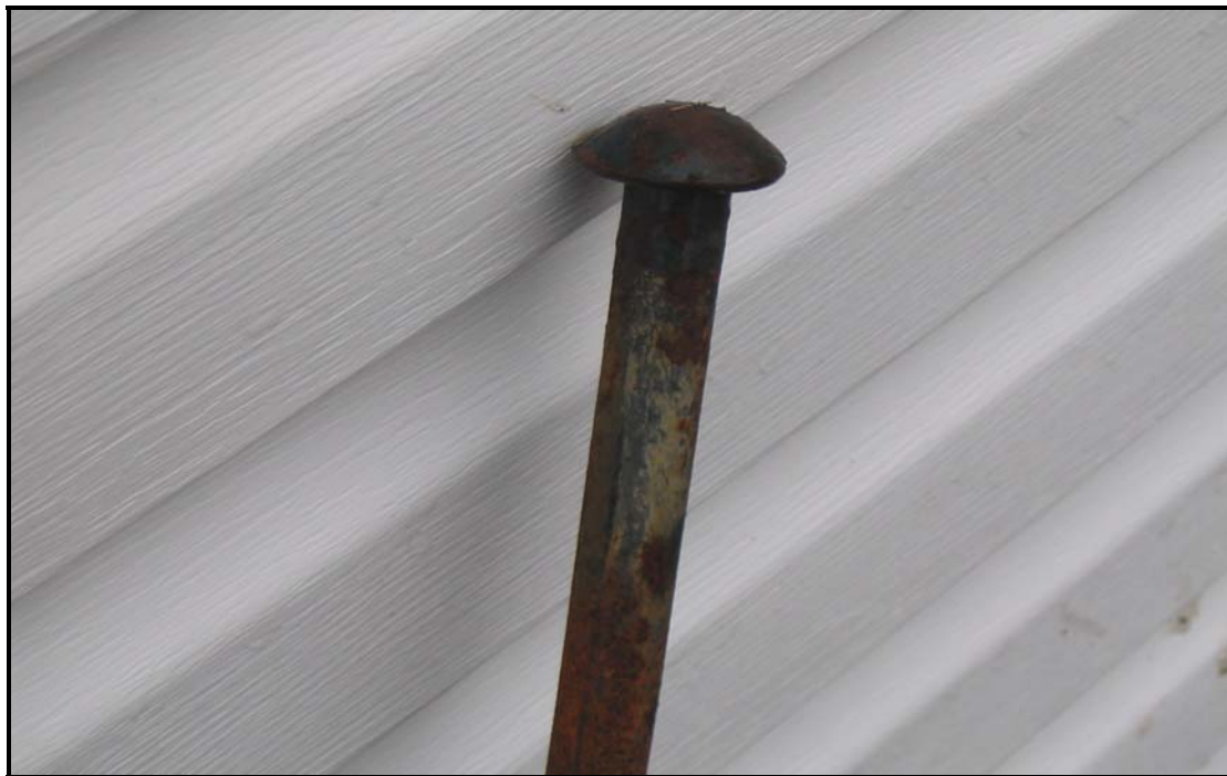
Photograph #28 – Typical un-corroded steel band button head.
