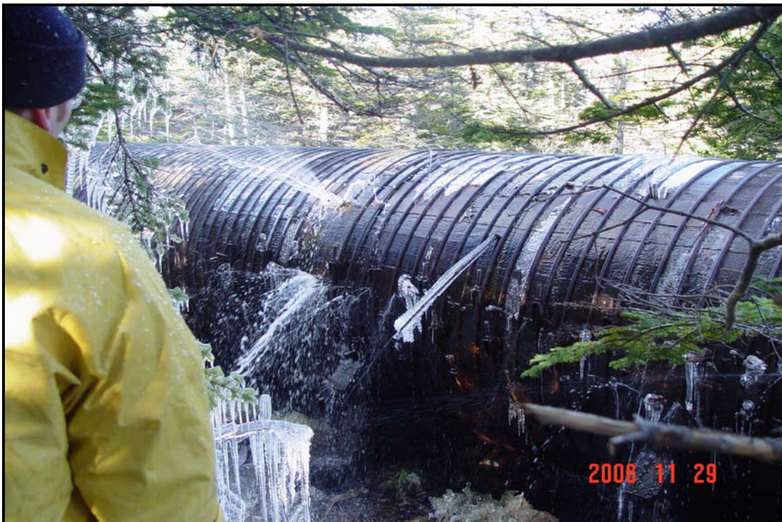
Photograph #10 – Several missing bands at one location near the intake end.
