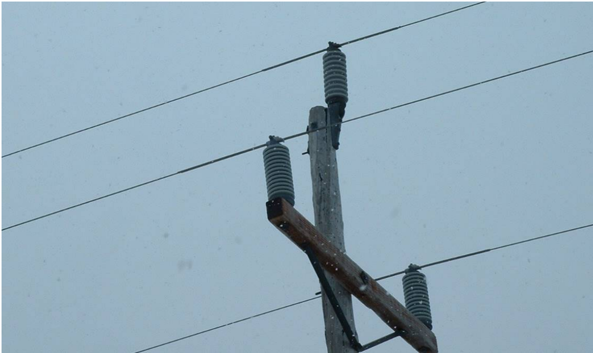
Figure 7 – Deteriorated Pole (Top Split) 111L
