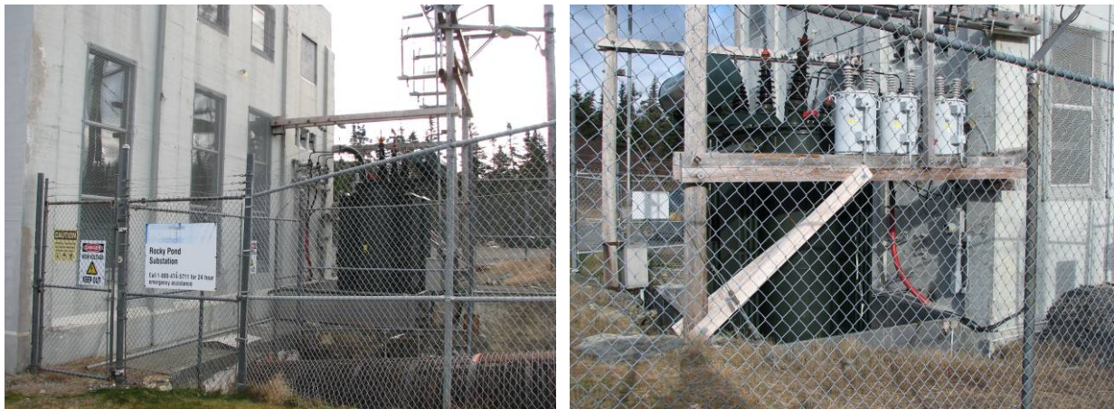
Existing Substation – Penstock Inside Yard - Inadequate Clearances
