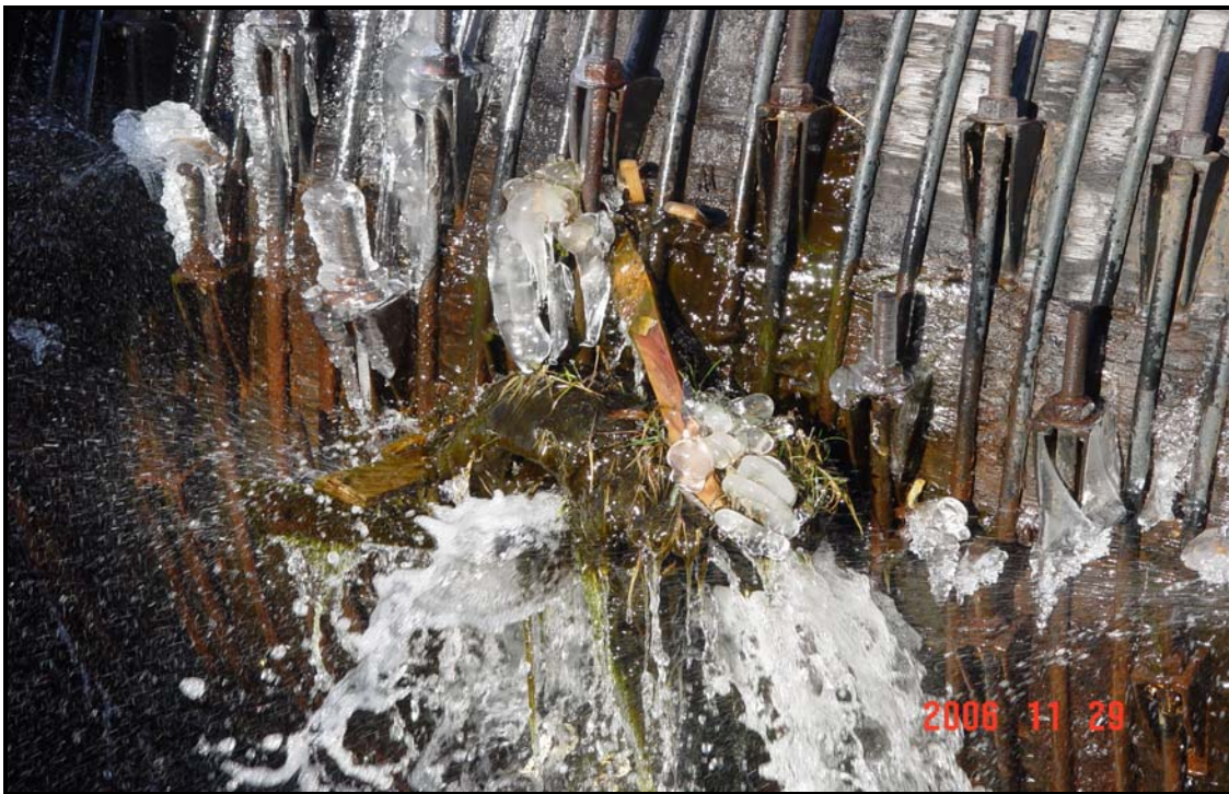
Photograph #5 – Use of sod in repair. Note steel band corrosion.
