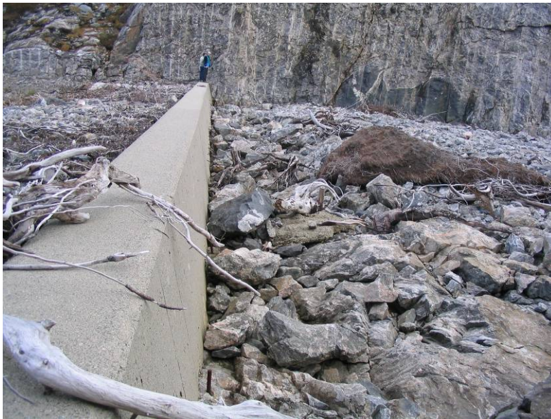
Picture 2: Existing Concrete Overflow Spillway
