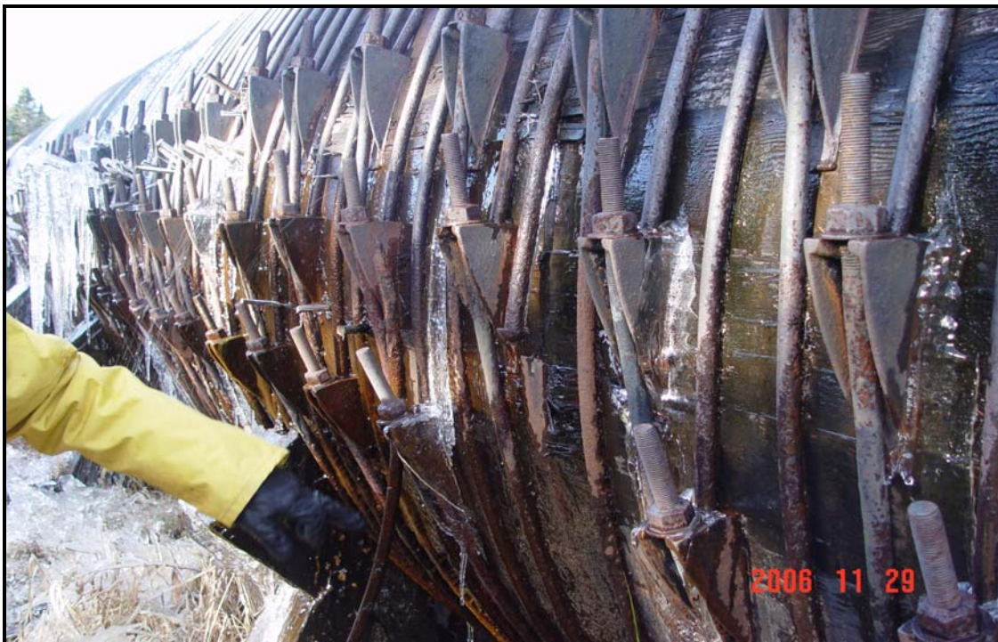
Photographs #8 – Band failed due to corrosion.
