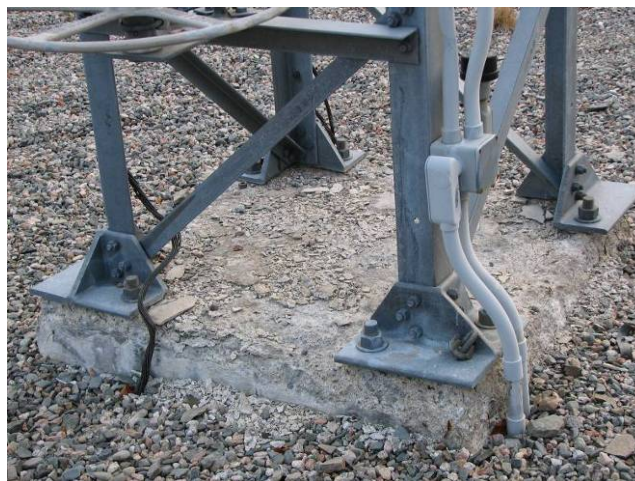
138 kV Structure Foundation
