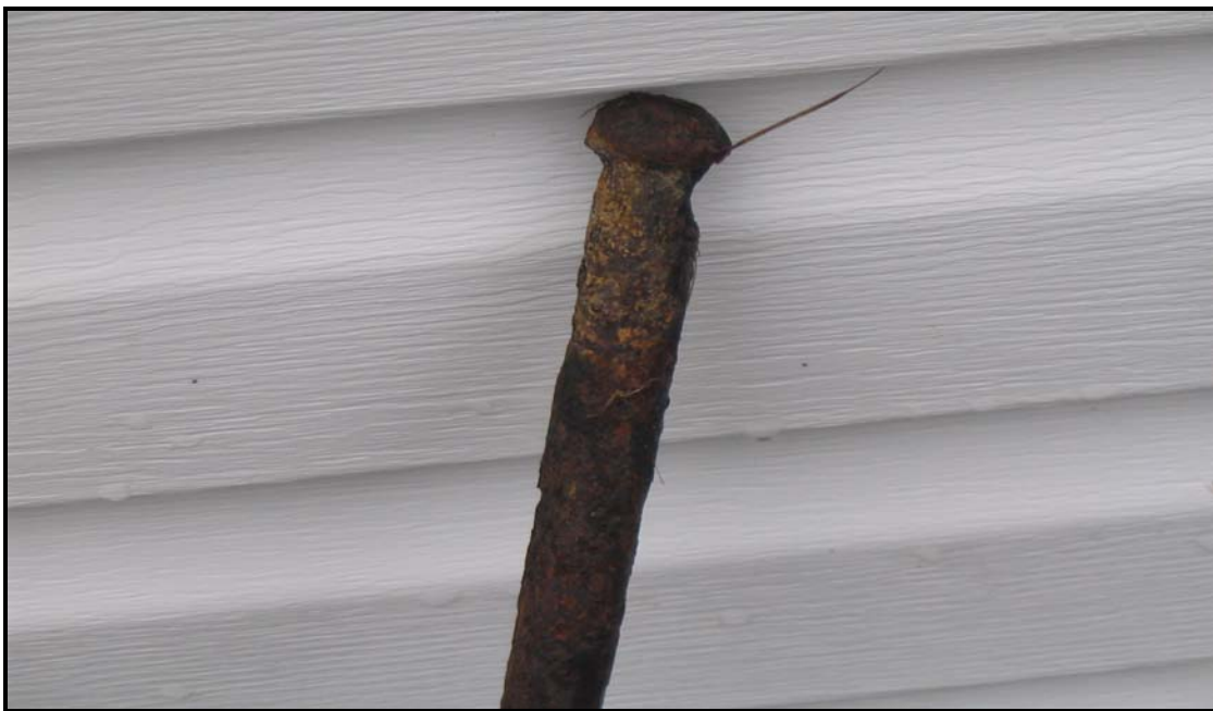
Photograph #26 – Typical corroded steel band button head.
