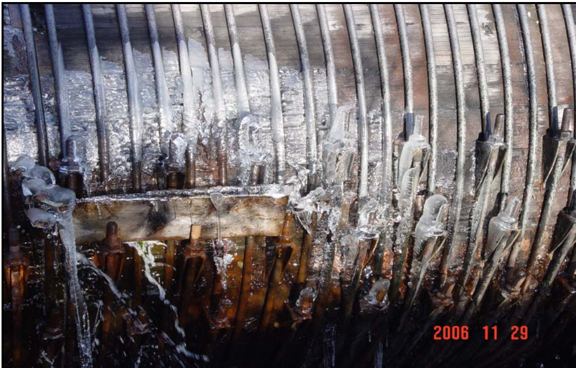
Photograph #4 – Typical repair – wooden board or slat.
