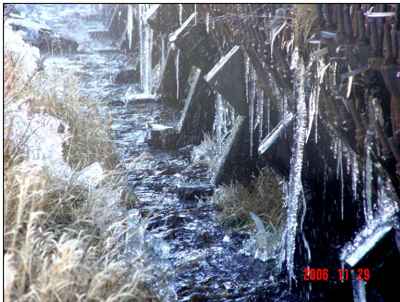
Picture 6: Poor drainage along Penstock
