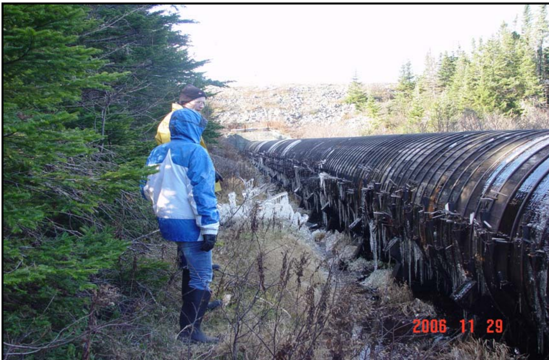
Photograph #11 – Near the intake conduit. Note the wedges near the top steel band connecting hardware.
