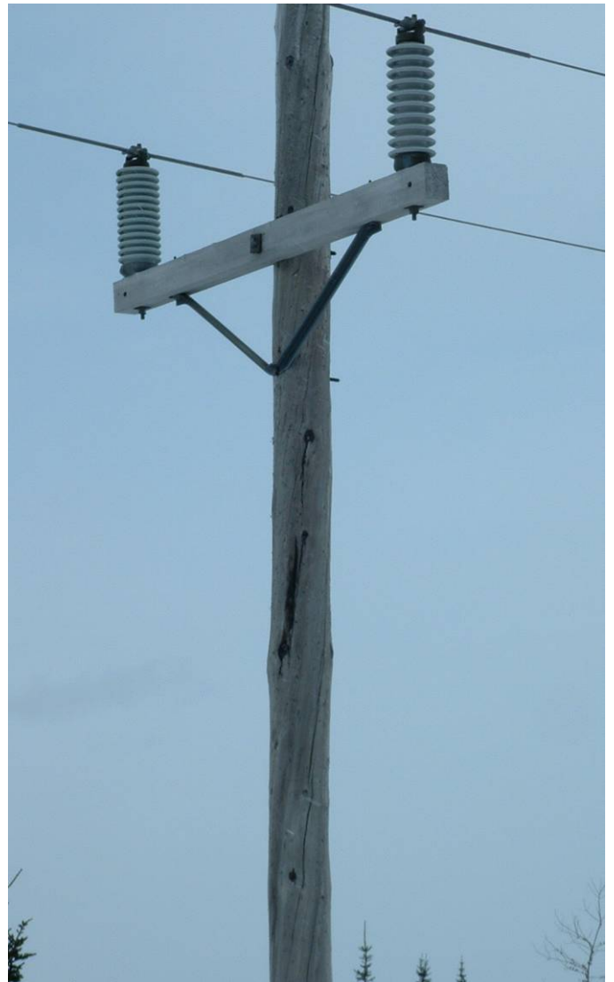
Figure 6 - Deteriorated Pole 111L
