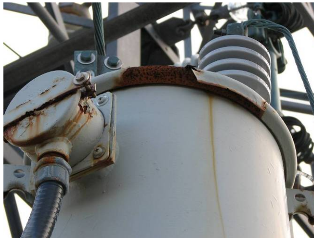
25 kV Potential Transformer
