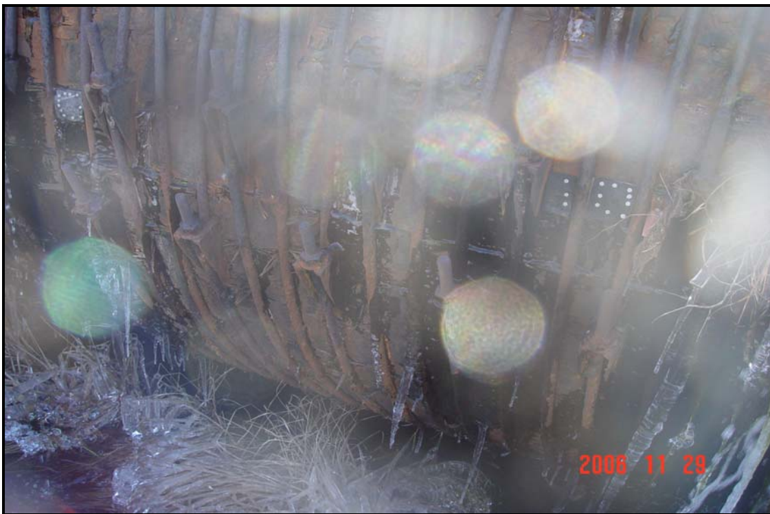
Photograph #20 – Close view of corrosion and vegetation at the foundation soil bed.
