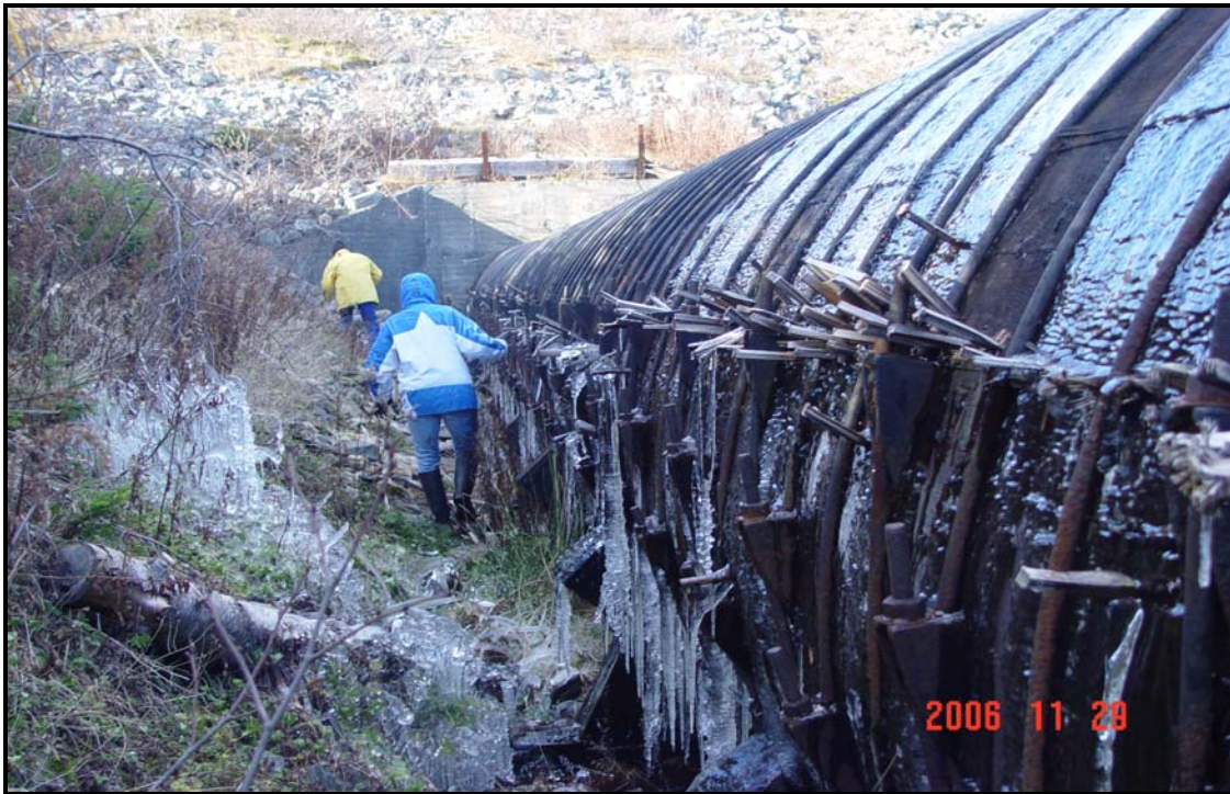
Photograph #13 – Extensive use of wedges to plug leaks near the intake.
