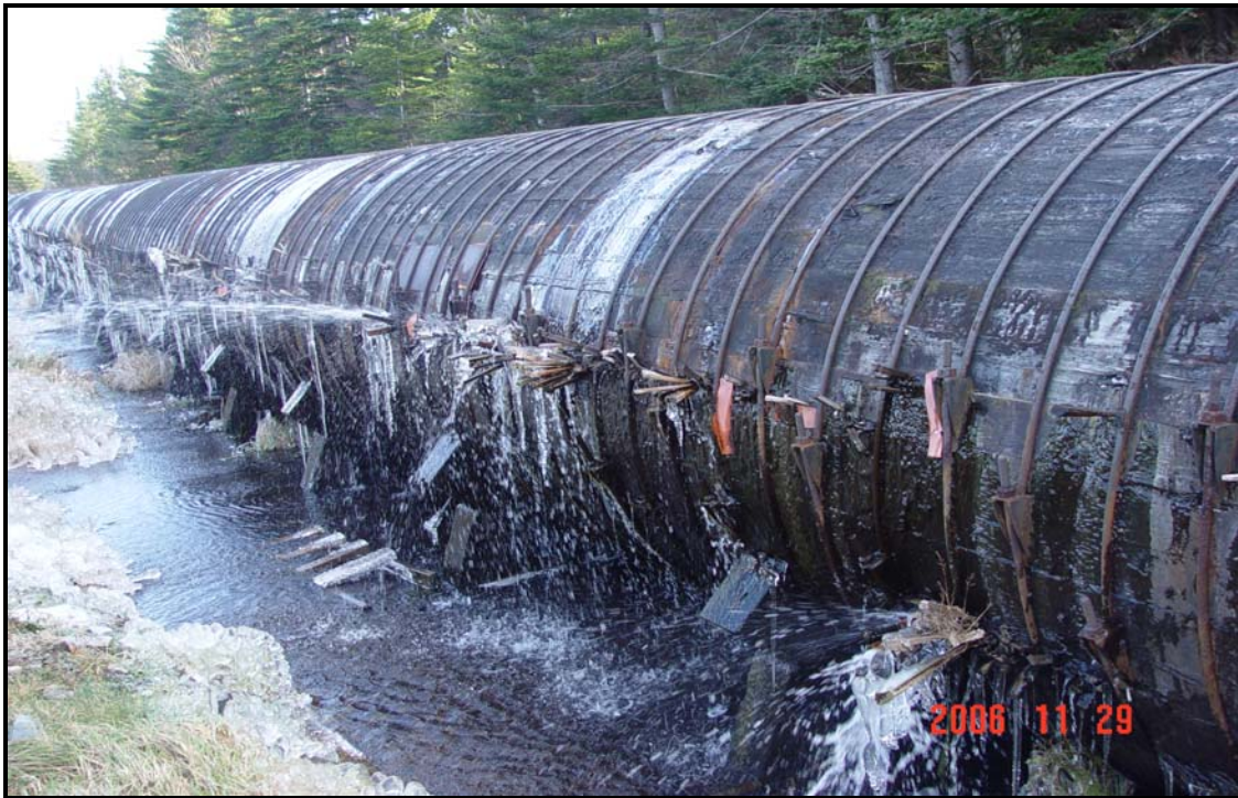
Photograph #17 – Several repairs and poor drainage and ventilation.
