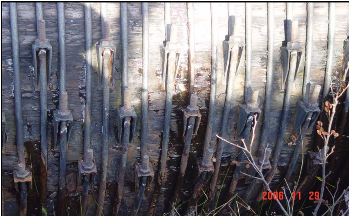
Photograph #2 – Wood stave crushing and corroded steel bands near the road bridge. Note there are no nut/washer keepers built into the band hardware.
