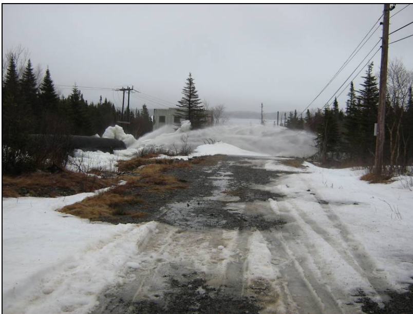
Picture 8: Major Leak Upstream of Powerhouse (March 8 th , 2008)
