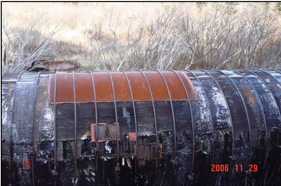
Photograph #12 – Typical large area repairs with steel plate and rubber gasket.
