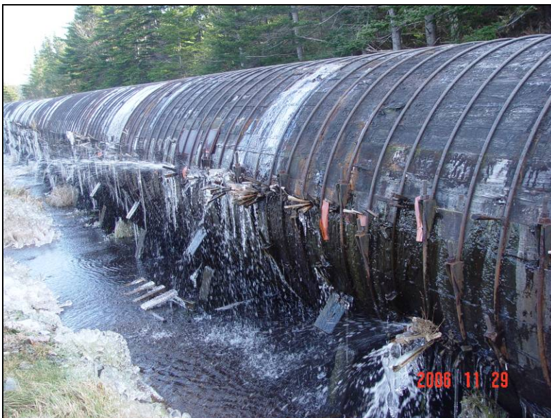
Picture 4: Poor drainage along Penstock
