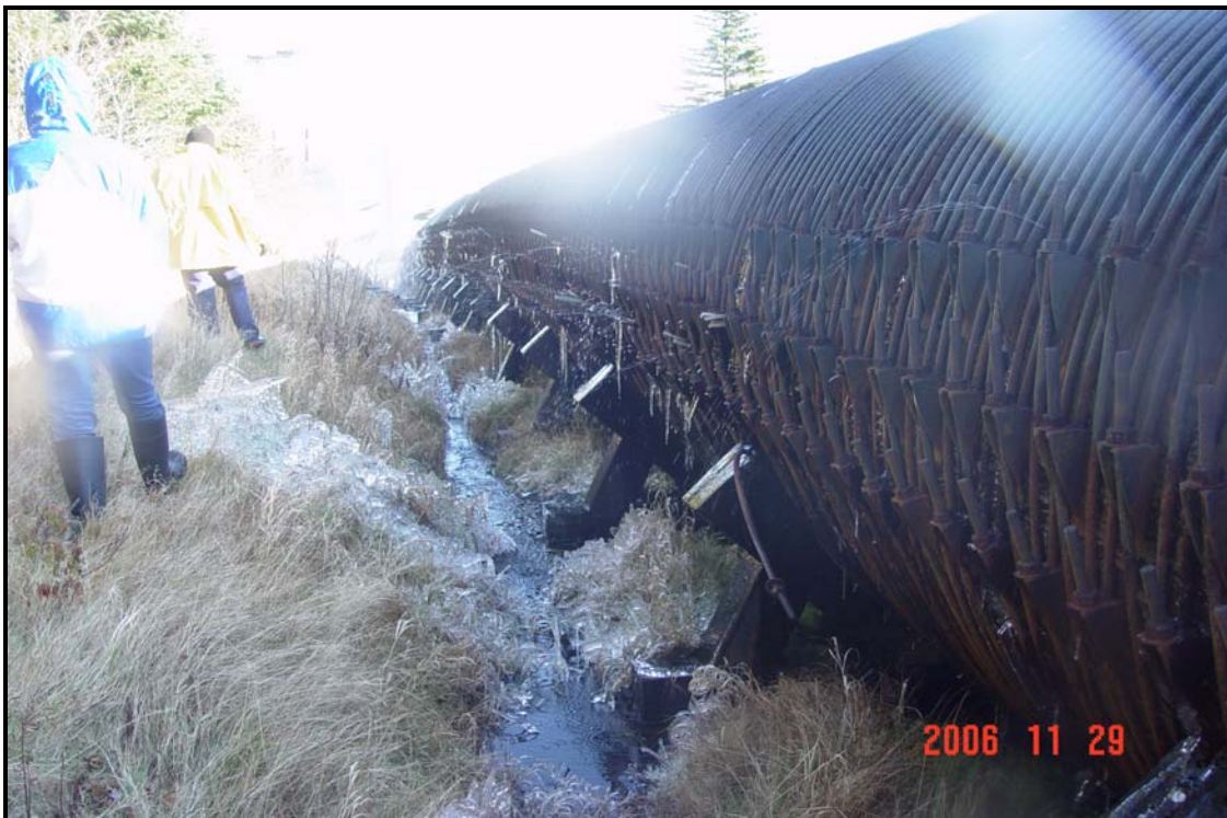
Photograph #23 – Missing steel band near the powerhouse.
