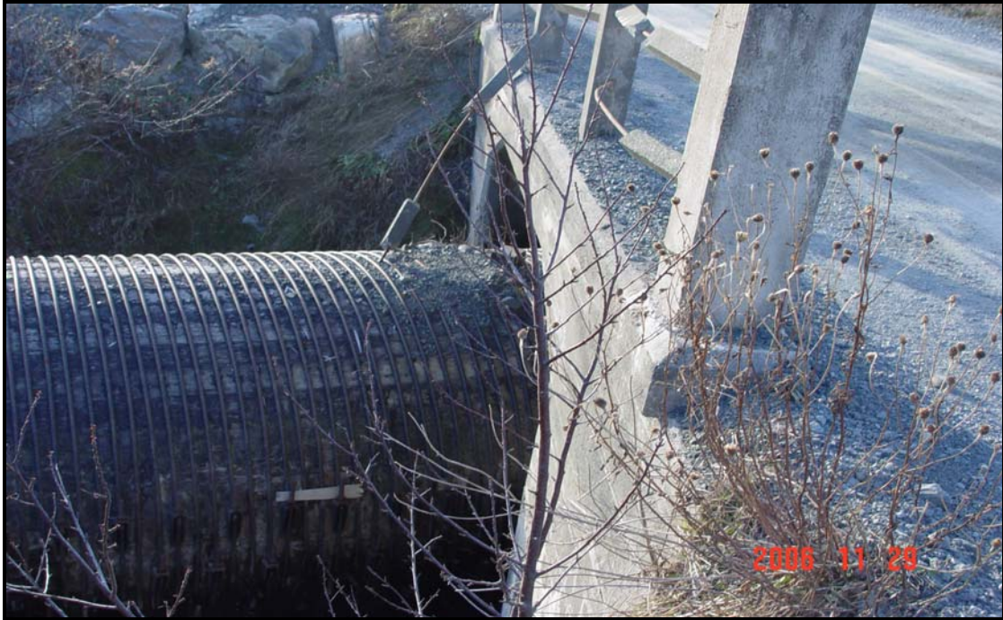
Photograph #1 – Soil and concrete on pipe at the road bridge.
