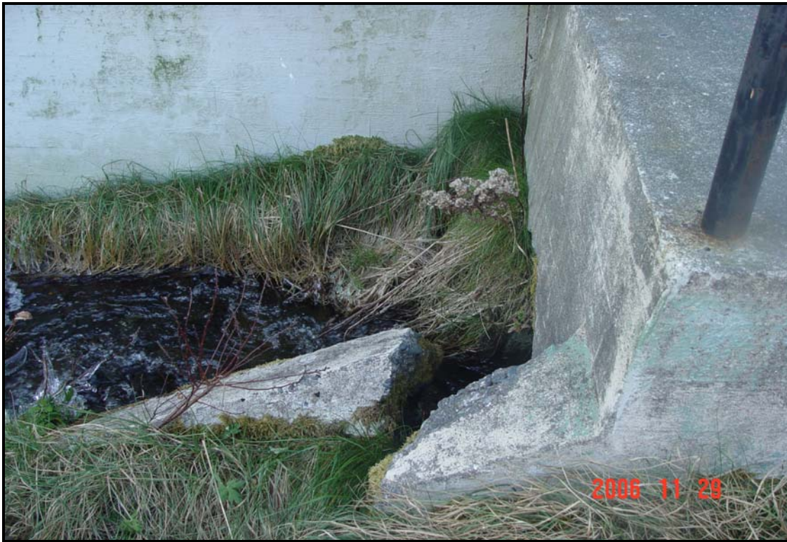
Photograph #25 – Significant penstock drainage under the repair bay. View is at the downstream of the powerhouse.
