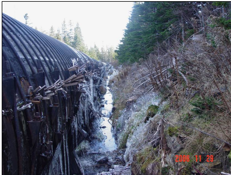
Picture 11: Leakage Repair near Intake
