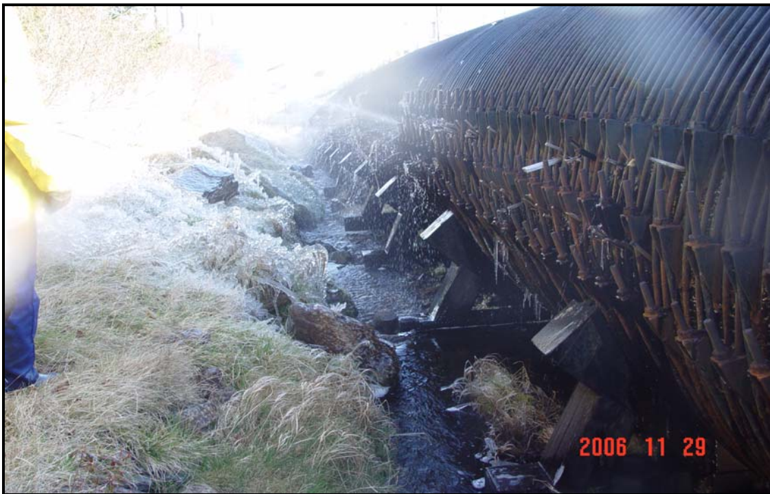
Photograph #24 – Poor drainage and ventilation near the powerhouse. Note the undercut cradle sleeper near centre photograph.
