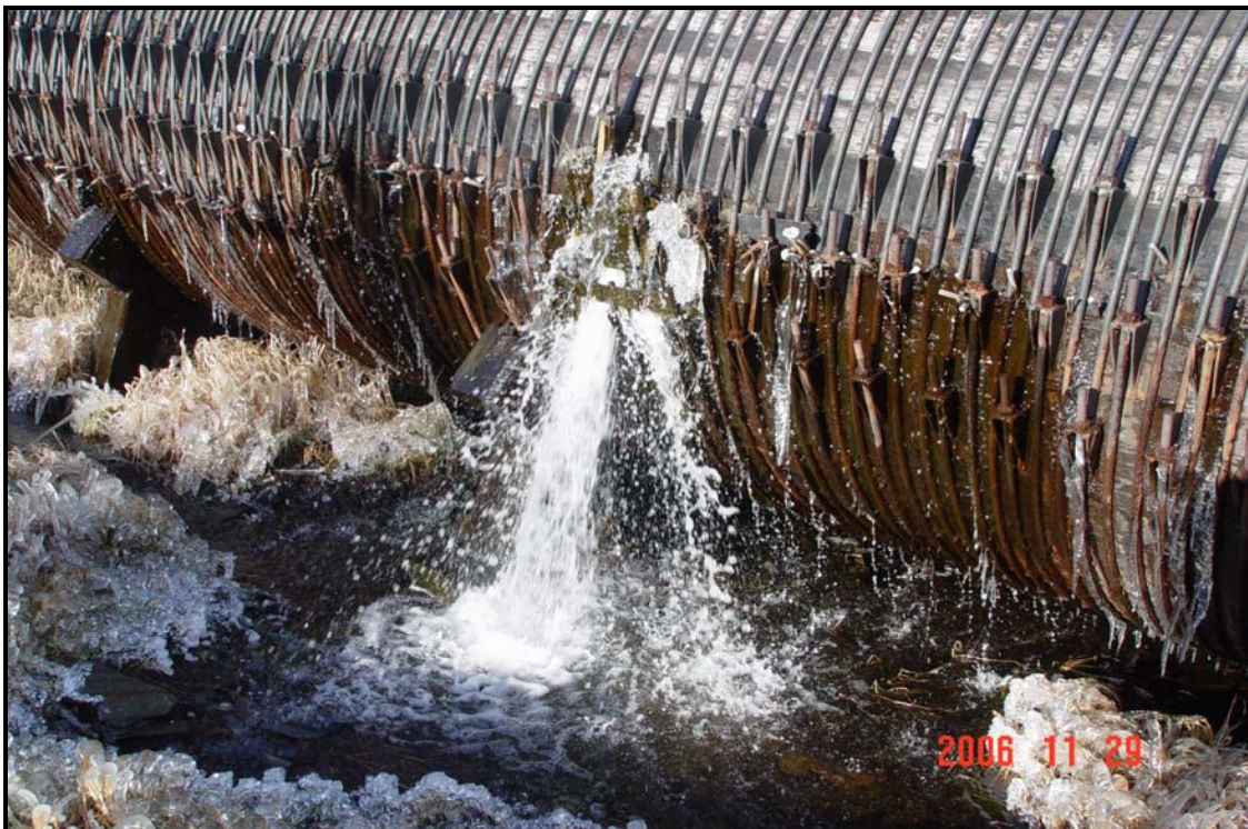
Photograph #6 – Extensive leakage at a repair area.
