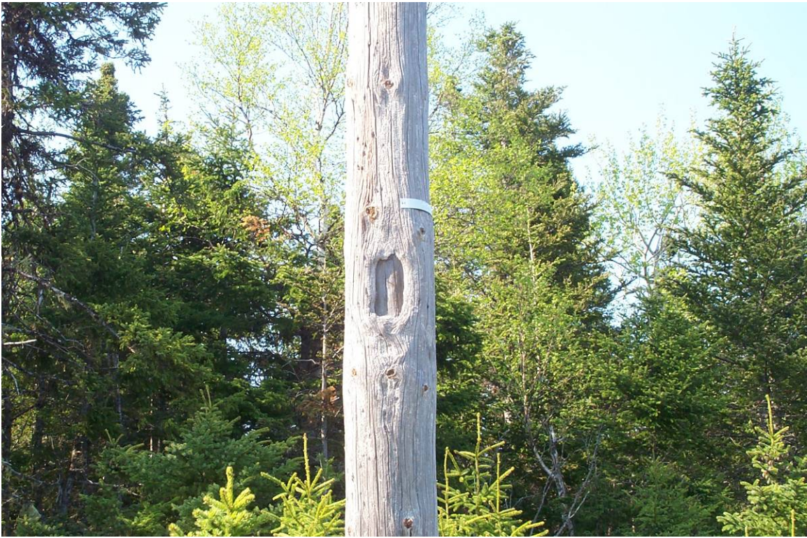
Figure 3 - Deteriorated pole 110L
