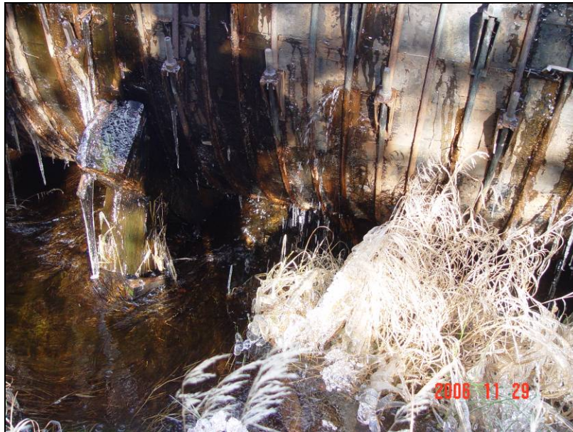
Picture 9: Undermining and Support Settlement into Penstock Bedding
