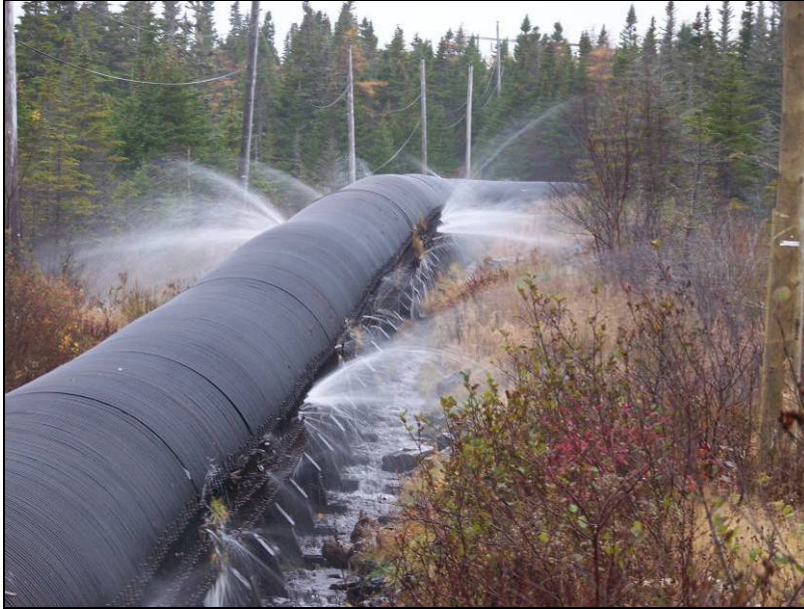
Picture 1: Water Leakage from Penstock
