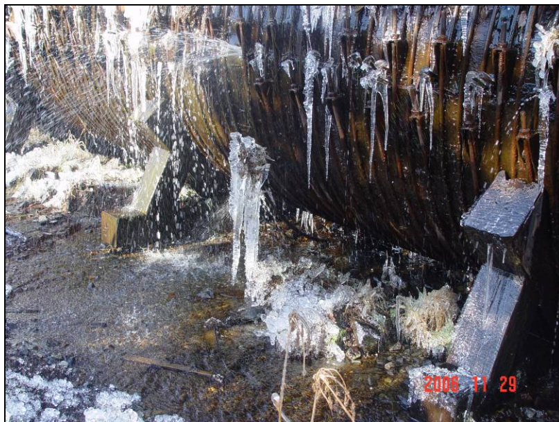
Picture 10: Settlement of Penstock Supports into Bedding
