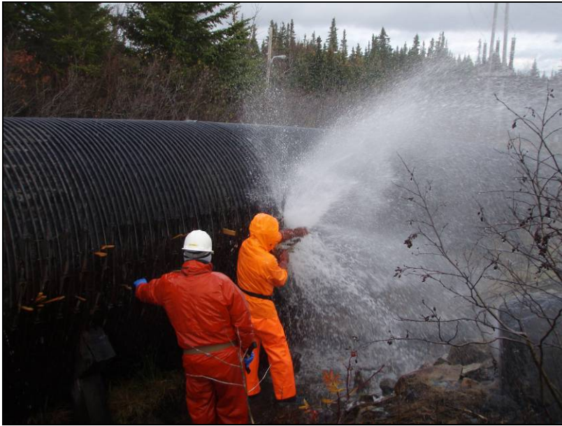
Picture 3: Maintenance Personnel attempting to plug leaks in Penstock
