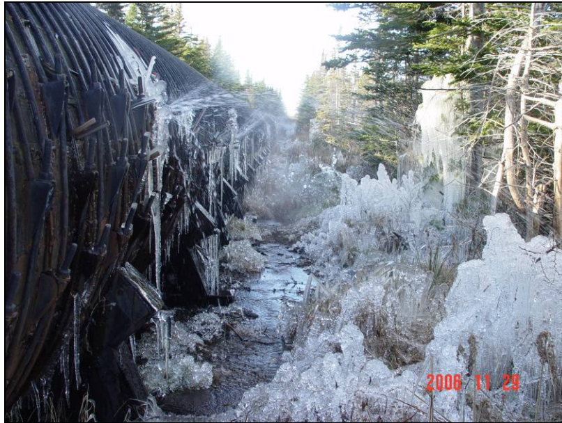
Picture 5: Poor drainage along Penstock
