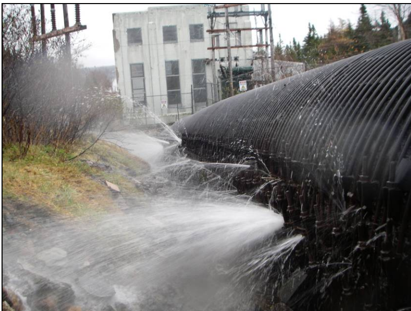
Picture 2: Water Leakage from Penstock
