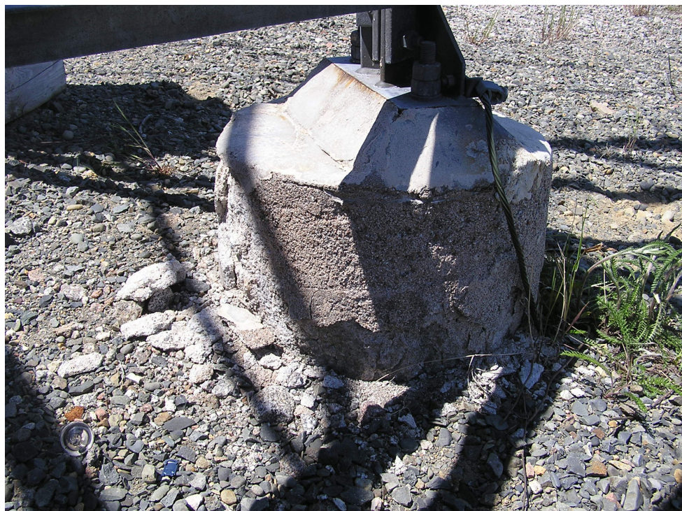
Photo #4: Deteriorated Foundation
