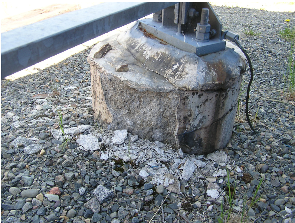
Photo #3: Deteriorated Foundation
