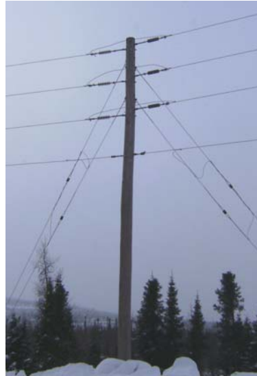
Figure 2. Substandard Guying of E Type Structure
