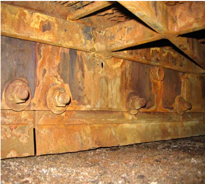
Figure 1 – Air Preheater Cold End: Extensive Corrosion
