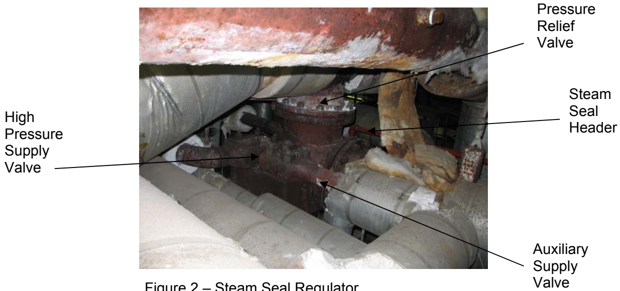
Figure 2 – Steam Seal Regulator
