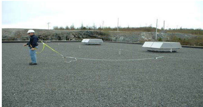
Figure 1. Roof Fall Arrest Protection System
