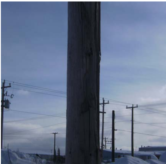
Figure 3. Damaged Pole Requiring Replacement
