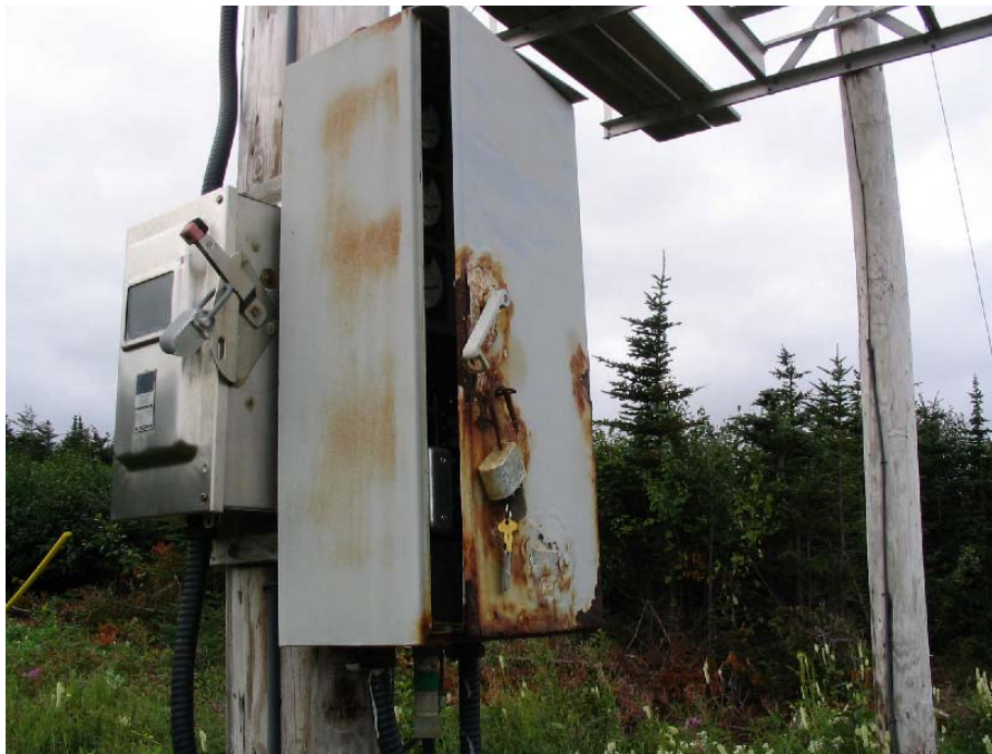
Figure 2. Outside of Recloser Control Panel
