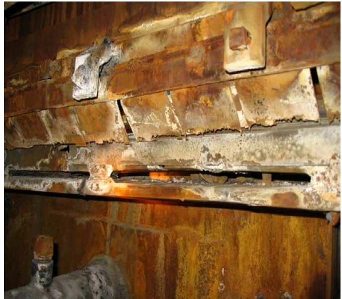
Figure 2 – Air Preheater Cold End: Extensive Corrosion
