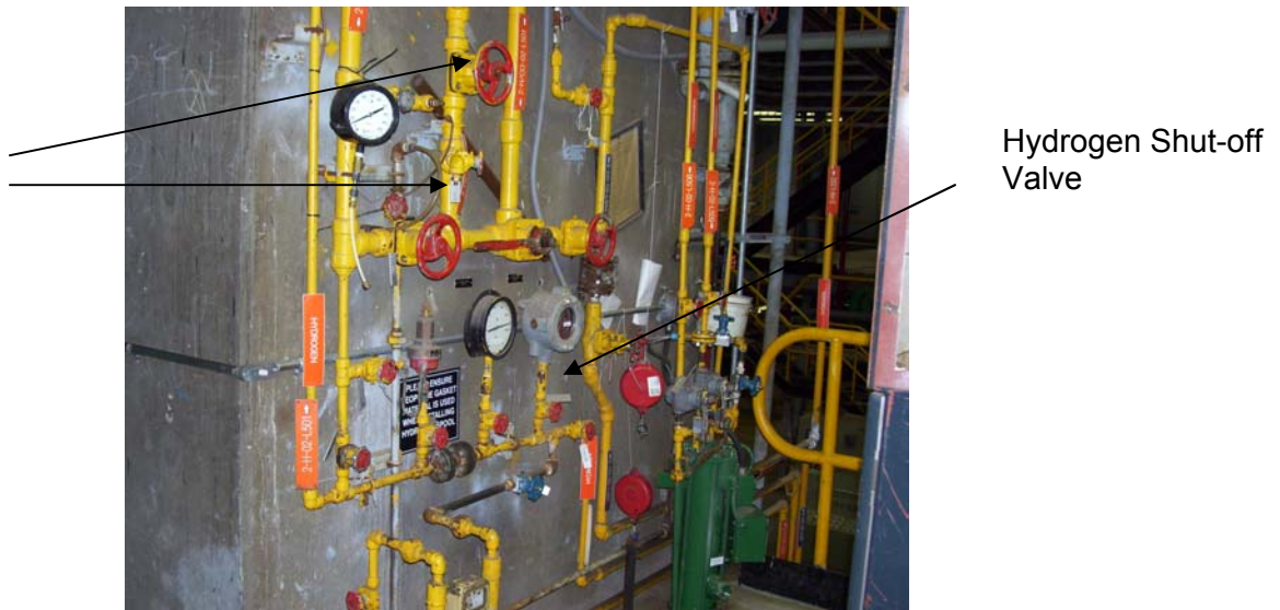
Figure 1. Unit 1 Hydrogen Valve Station
