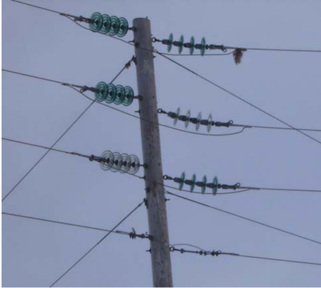
Figure 1. Substandard 46 kV E Type Structure
