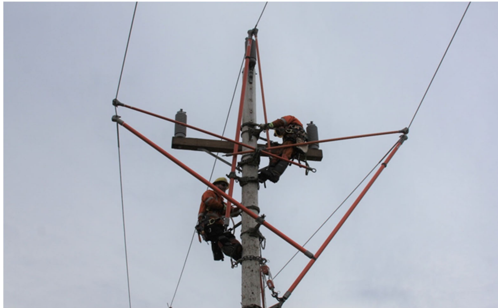
Figure 2 - Typical Hotline Setup on Single Pole Structure
