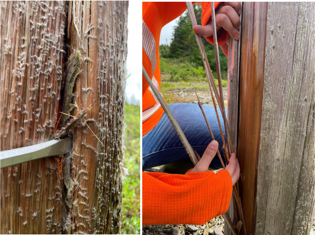
Figure 1 - Shell Separation
