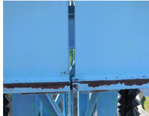
Figure 10: Alignment Gaps in Monorail Beam
