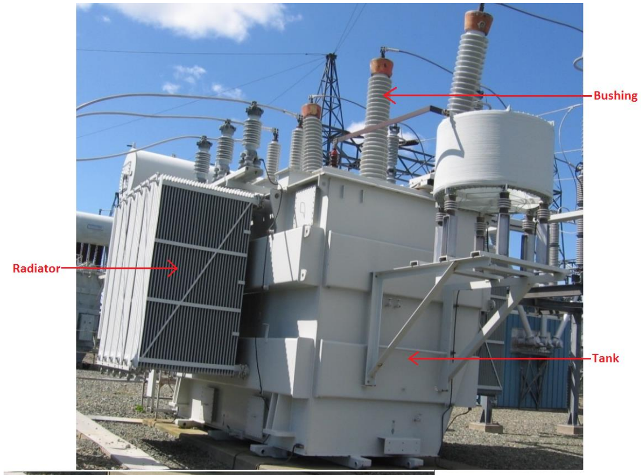
Figure 8: Power Transformer
