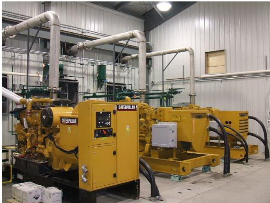
Figure 3: St. Lewis Diesel Generators in Power House
