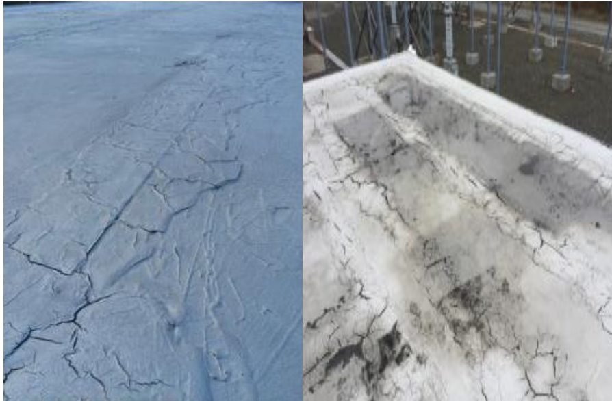
Figure 16: Terminal Station Control Buildings (Come by Chance and Sunnyside) Showing Cracking and Deterioration of the Roof Membrane System
