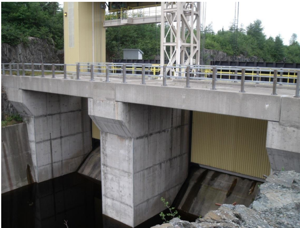
Figure 5: West Salmon Spillway Control Structure
