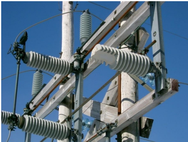
Figure 4: Broken Insulator on 69 kV Disconnect Switch
