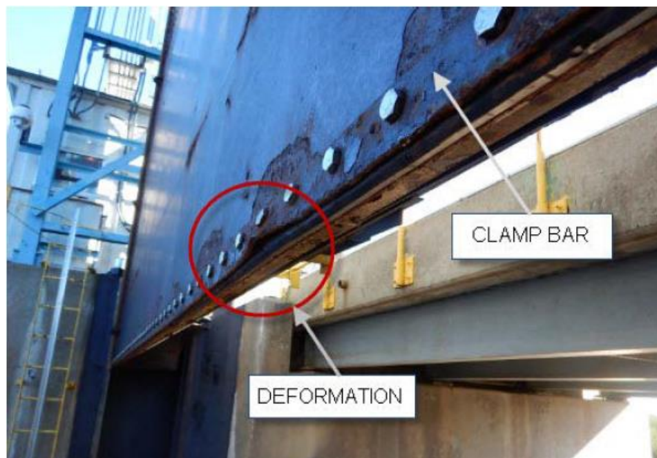
Figure 15: Deformed Gate Knife – Burnt Dam
