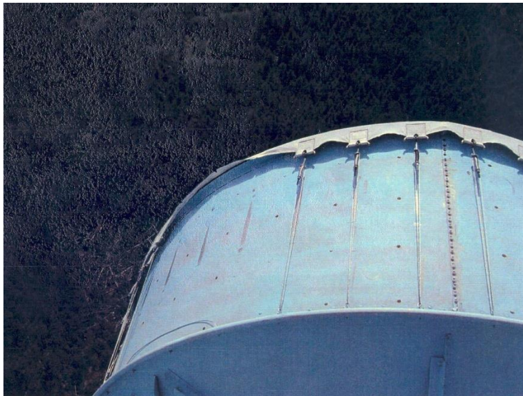
Figure 4: Missing Radome Mounts
