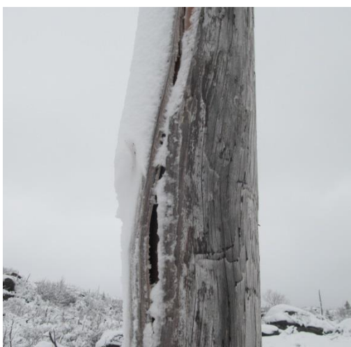
Figure 3: Deteriorated Pole
