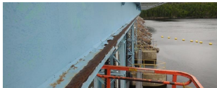
Figure 13: Corrosion along the Monorail Beam Roller Plates
