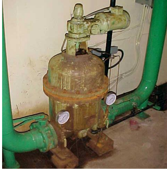
Figure 19: Upper Salmon Rotary Strainer
