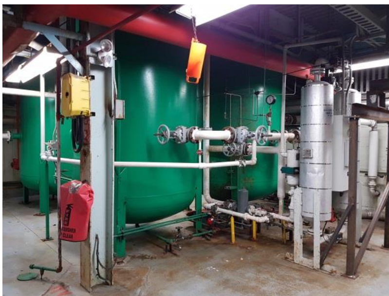
Figure 1: Compressed Air Receiver Tanks in Powerhouse
