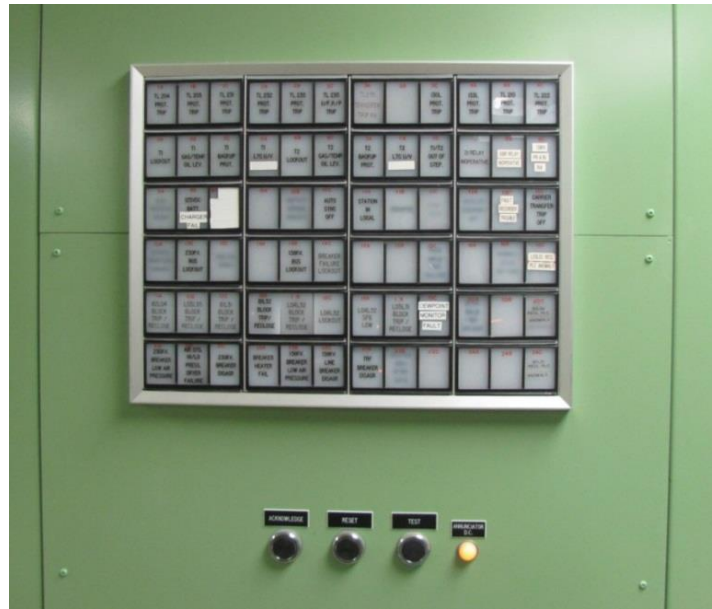
Figure 19: Annunciator Commonly Found in Hydro Terminal Stations
