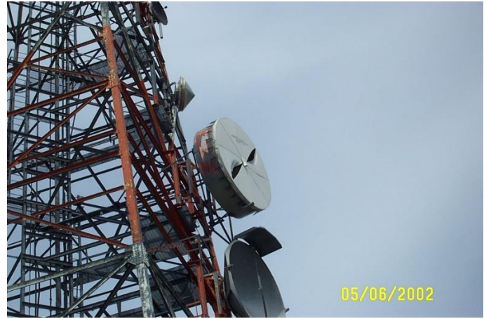
Figure 3: Heavily Damaged Radome
