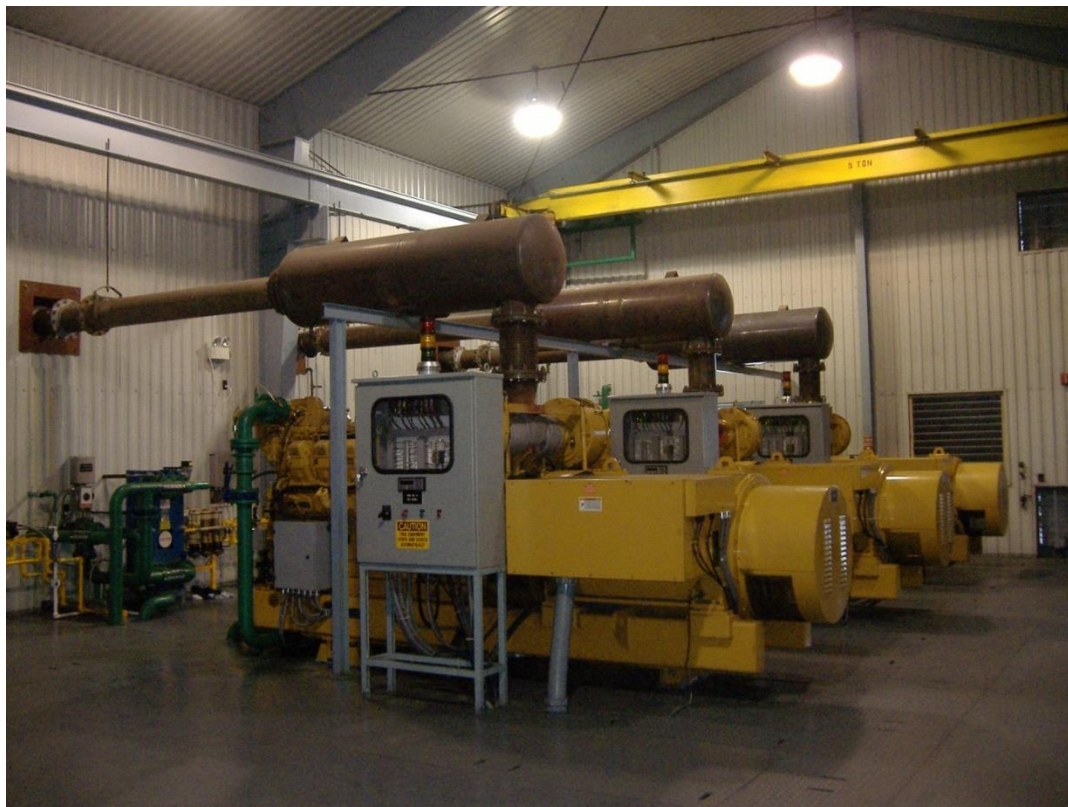
Figure 2: Ramea Diesel Generating Units
