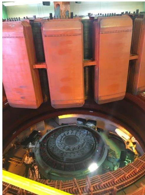
Figure 3: Dismantled Generator
