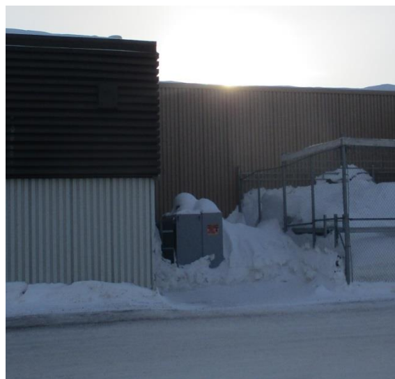
Figure 4: Existing Pad-Mounted Transformer
