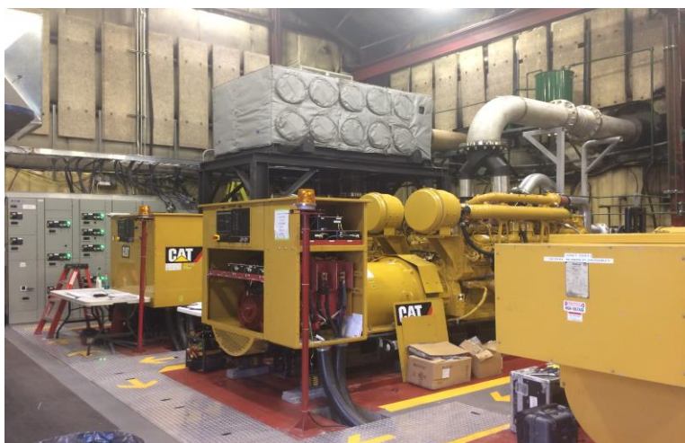
Figure 3: L’Anse-au-Loup Diesel Generators in Power House
