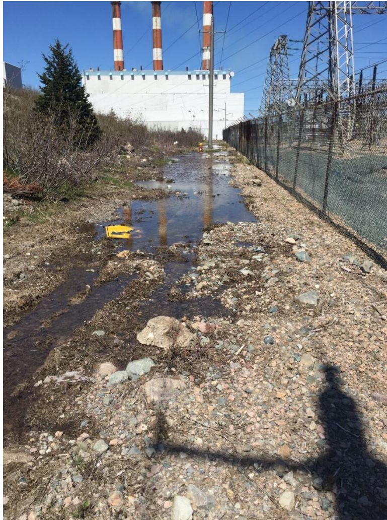
Figure 2: Fire Distribution Line Leakage near the Terminal Station.
