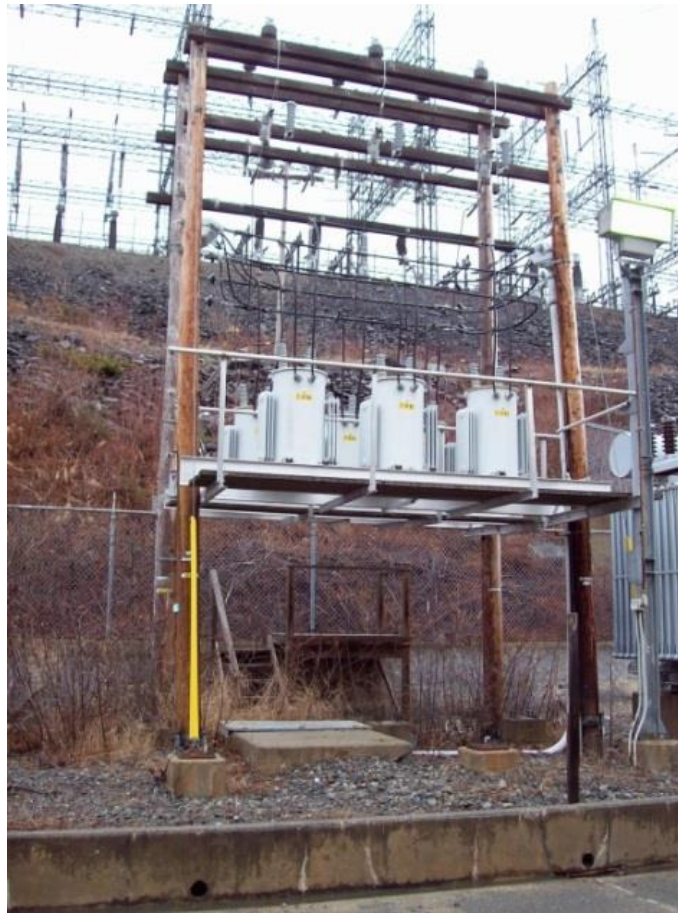
Figure 11: Bay D'Espoir– Station Service Transformers
