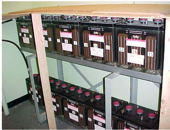
Figure 10: 125 Vdc Terminal Station Battery Bank
