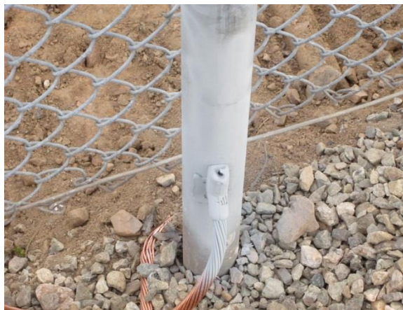
Figure 7: Typical Grounding Connection on Terminal Station Fence
