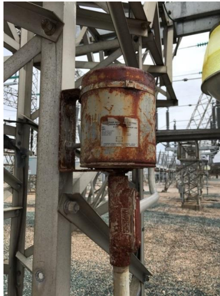
Figure 12: Corroded Ballast Requiring Replacement
