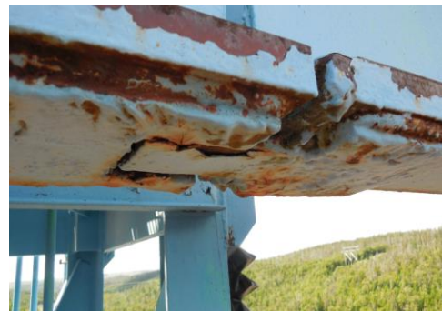
Figure 12: Monorail Beam Scaling
