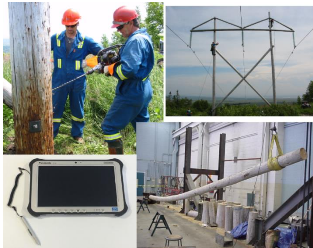
Figure 1: Wood Pole Line Management Inspection Techniques. Clockwise from Bottom Left: (1) Field Data Collector, (2) Installing Boron Treatment, (3) Climbing Inspection, (4) Destructive Testing at Memorial University of Newfoundland
