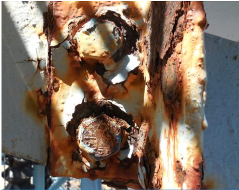
Figure 9: Structure Bolt Scaling
