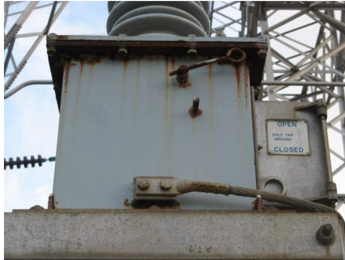
Figure 2: Rusting Potential Transformer
