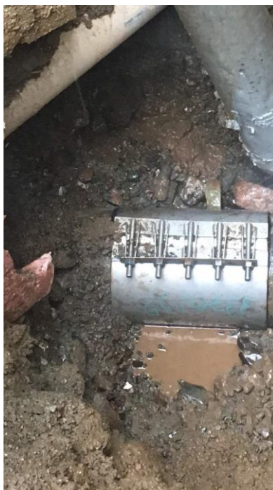
Figure 1: Fire Distribution Line Break behind the Stack of Unit 2
