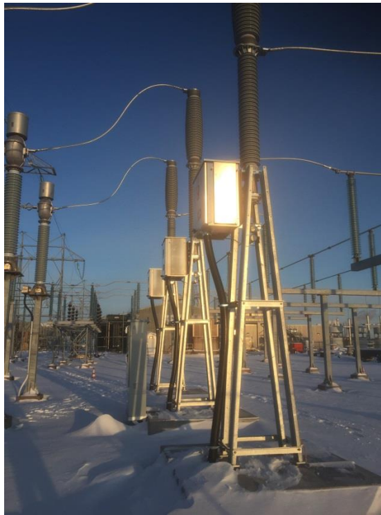
Figure 2: Live Tank Circuit Breaker Wabush Terminal Station 230-2
