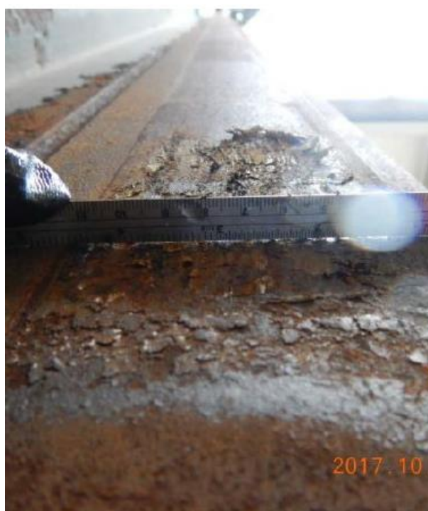
Figure 16: Rubbing Marks on Embedded Parts – Burnt Dam
