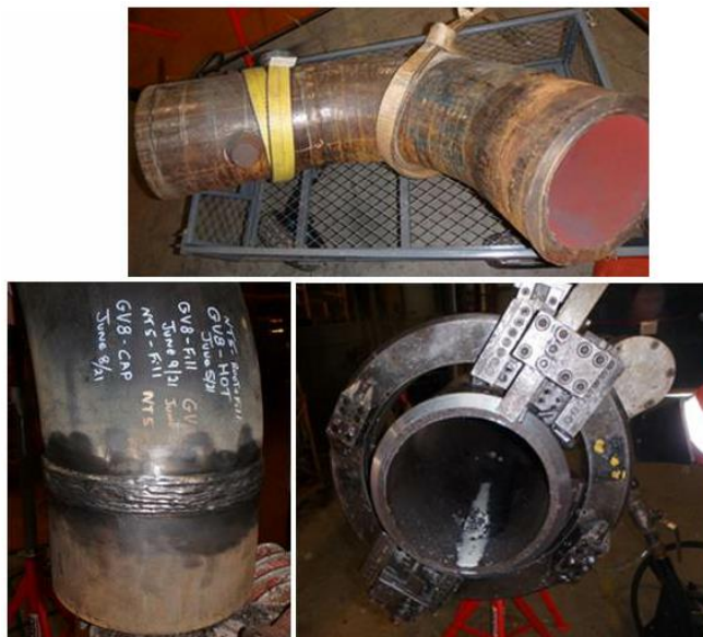
Figure 2: Unit 3 Feedwater Piping Replacement in Progress
