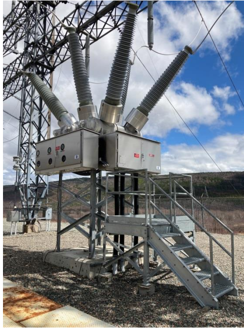
Figure 1: Dead Tank Circuit Breaker BDE B2T4
