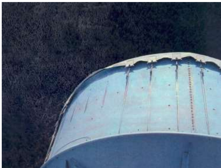
Figure 4: Missing Radome Mounts
