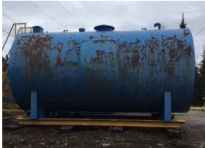
Figure 1: Failed Epoxy Coating and Rust on Tank (Side View)
