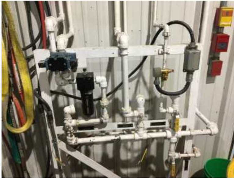
Figure 3: Snow Door Air Header at the Happy Valley Gas Turbine
