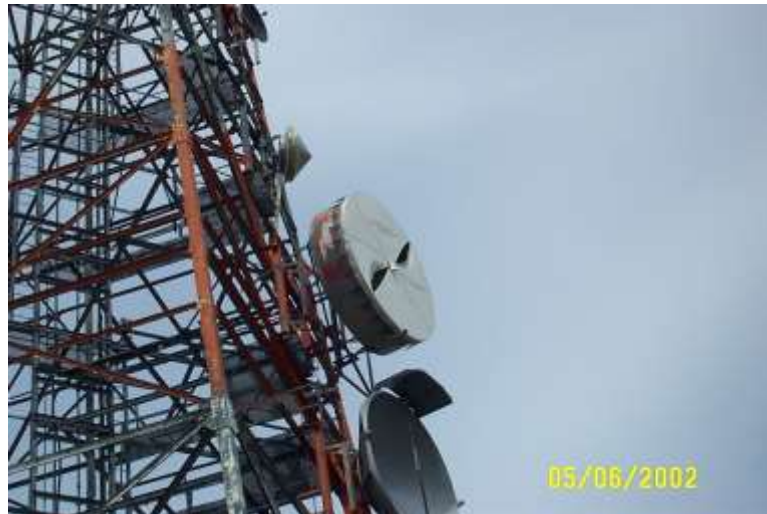
Figure 3: Heavily Damaged Radome
