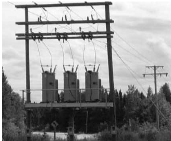
Figure 1: Typical Hydro 200 A Voltage Regulator Bank
