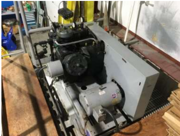
Figure 2: Air Compressors at the Happy Valley Gas Turbine
