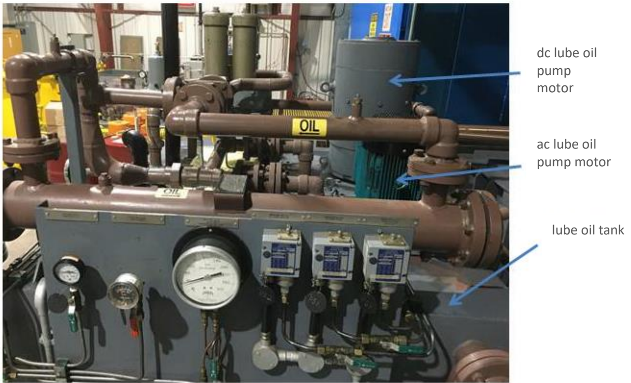
Figure 3: Lube Oil Pumps – Happy Valley Gas Turbine
