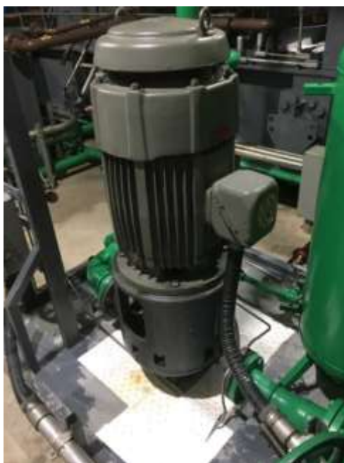
Figure 4: Glycol Pump - Happy Valley Gas Turbine
