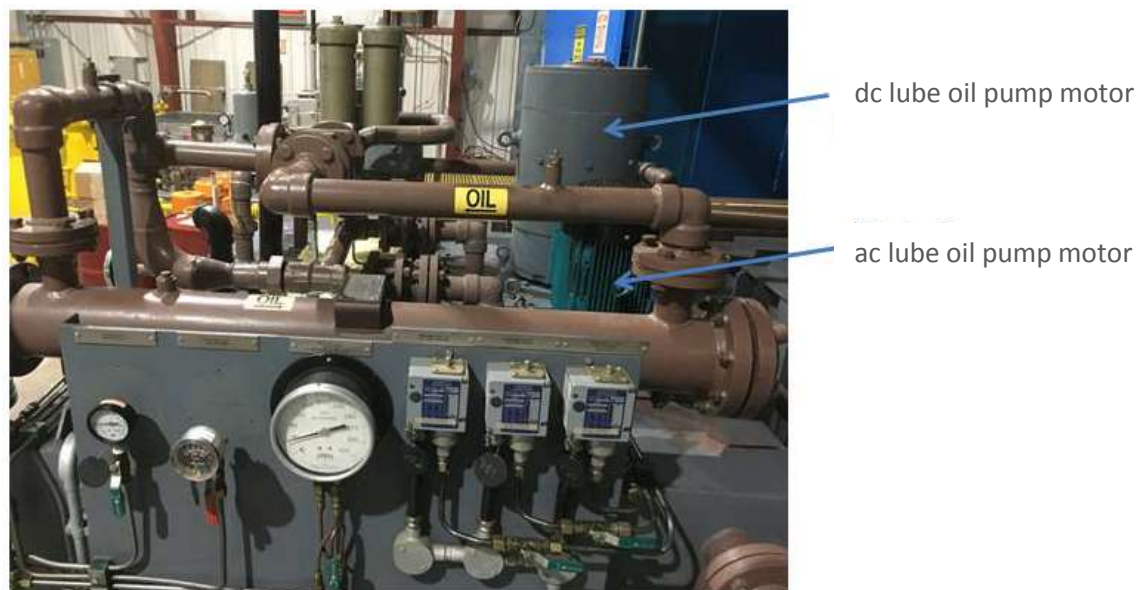
Figure 3: Lube Oil Pumps - Happy Valley Gas Turbine
