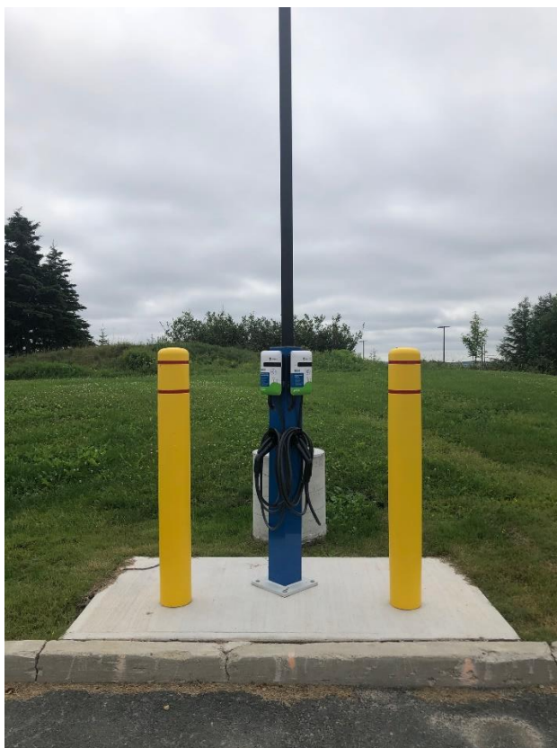
Figure 1: Duel Port Single Bollard Installation
