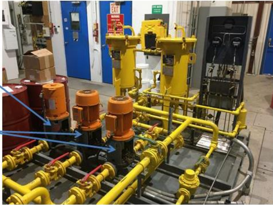
Figure 2: Fuel Oil Pumps – Happy Valley Gas Turbine
