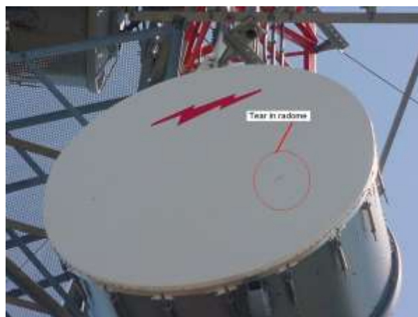
Figure 2: Tear in Radome
