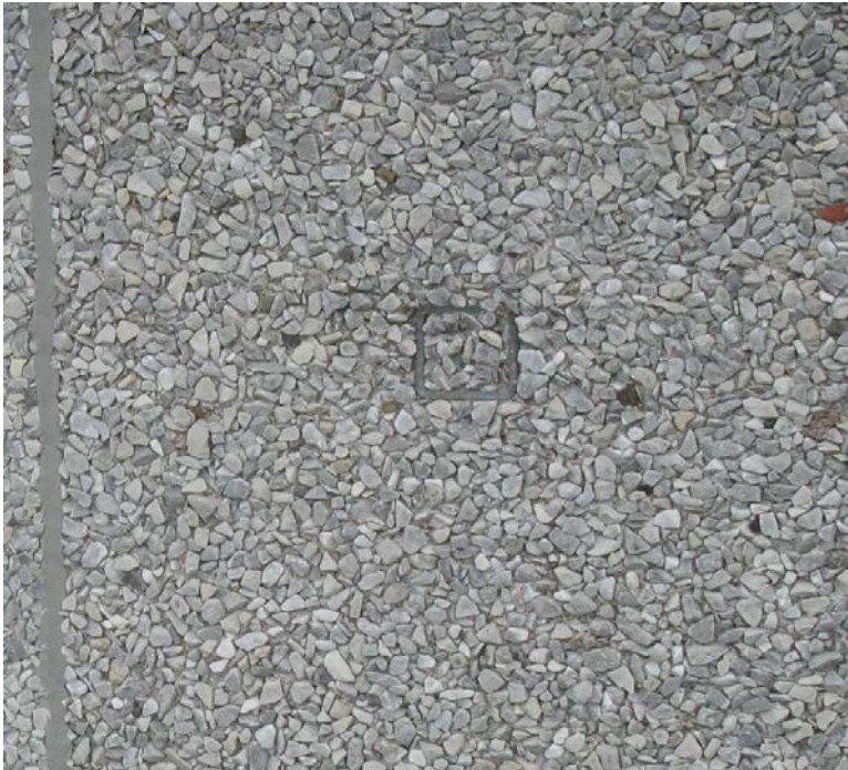
Photo 25: Visible panel support at exterior.
