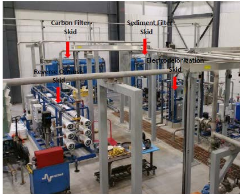
Figure 3: Demineralized Water System
