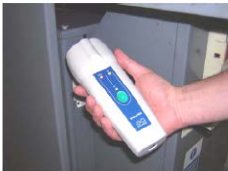
Red Indication Pointing Towards Switchgear
