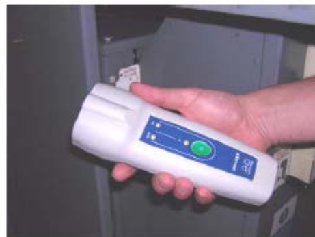
Green Indication Pointing Away From Switchgear
