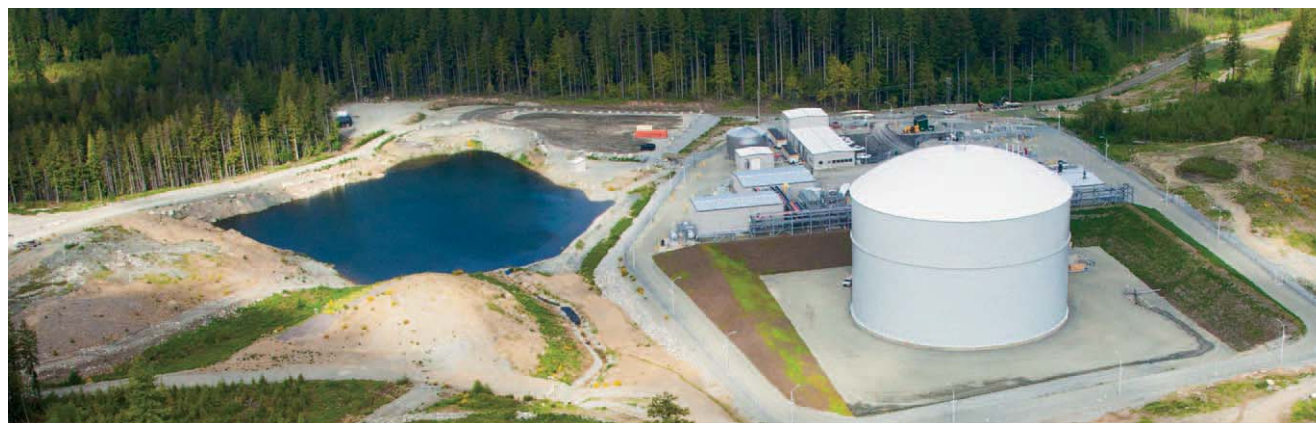
Construction of the $212 million 1.5 billion-cubic foot liquefied natural gas storage facility on Vancouver Island was completed in 2011.
