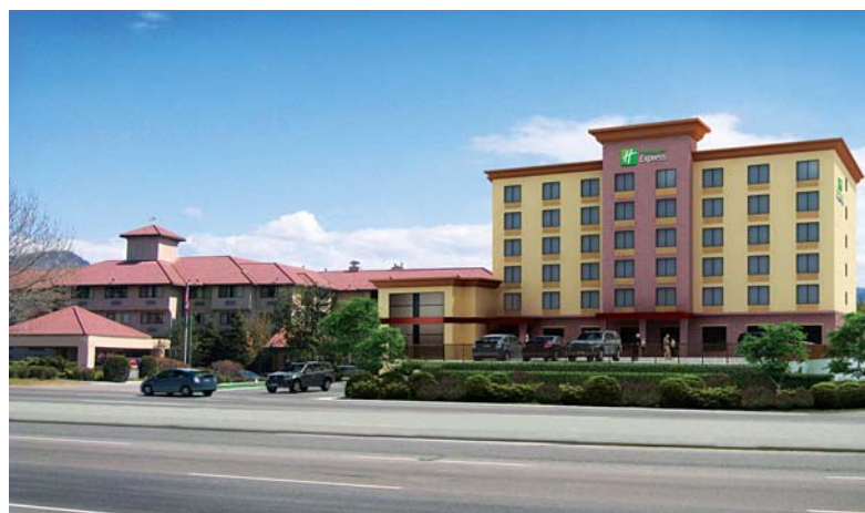
The 70-room expansion of the Holiday Inn Express Kelowna opened in February 2010.
