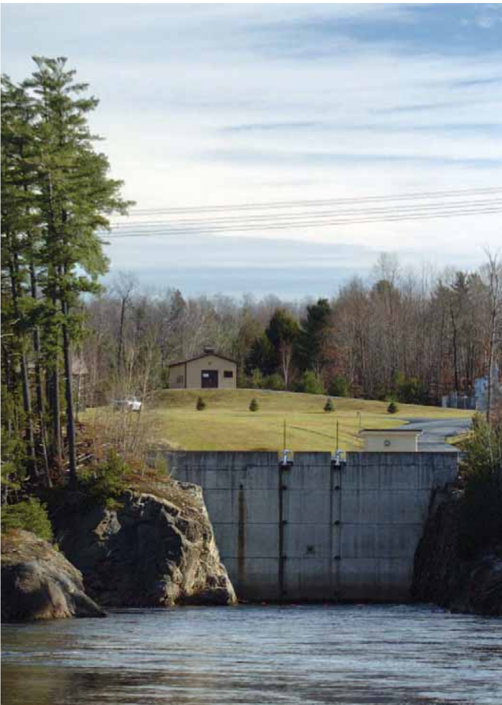
In Upper New York State, the non-regulated generating assets are 4 hydroelectric generating stations located in Moose River, Philadelphia, Dolgeville and Diana. The plants have a combined capacity of approximately 23 MW.
