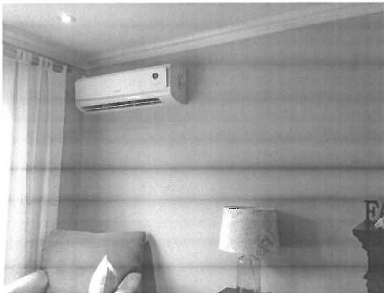
Figure 1 Indoor Air Handling Unit
