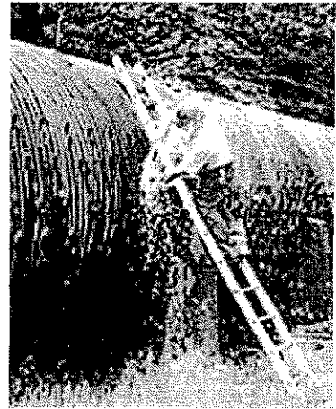
Figure No. 2: Maintenance of Wood Stave Penstock (Built in 1959)
