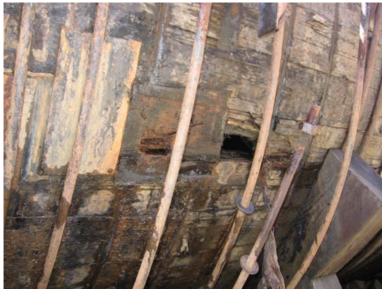
22 23 24 Figure 1 – Major Leak Downstream of TCH Bridge
