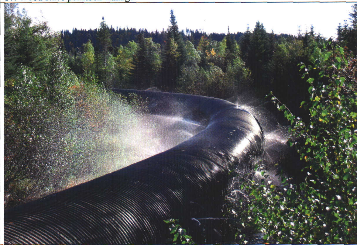
18. Wood stave penstock leakage.
