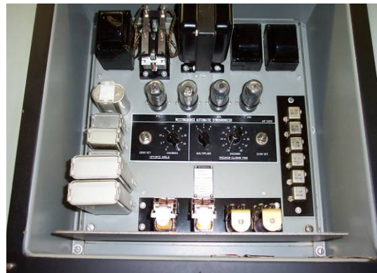
Figure 9 - Existing Synchronizer
