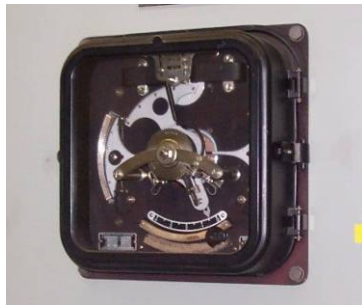
Figure 5 - Voltage Regulator
