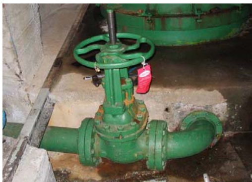
Figure 2 - Drain Valve
