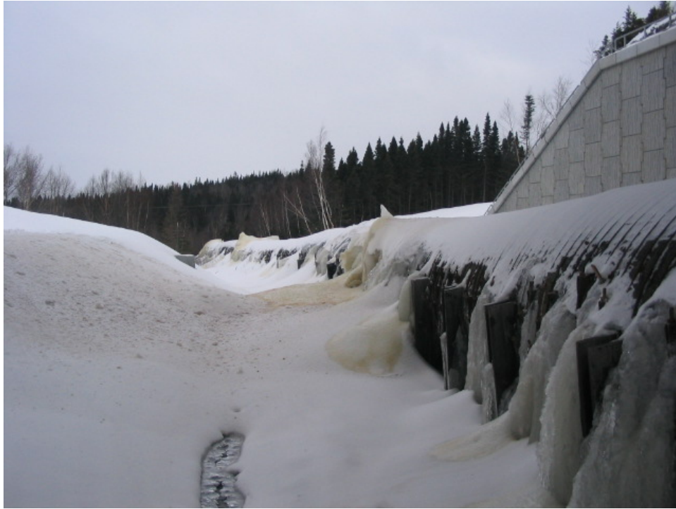
Figure 10: Ice Forming on Penstock during Winter
