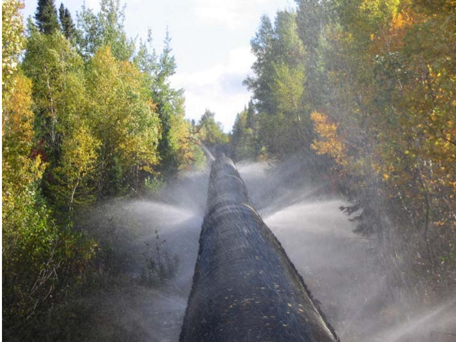
Figure 3: Water Leakage from Penstock
