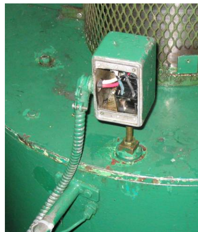
Figure 12 – Bearing Oil Level Switch
