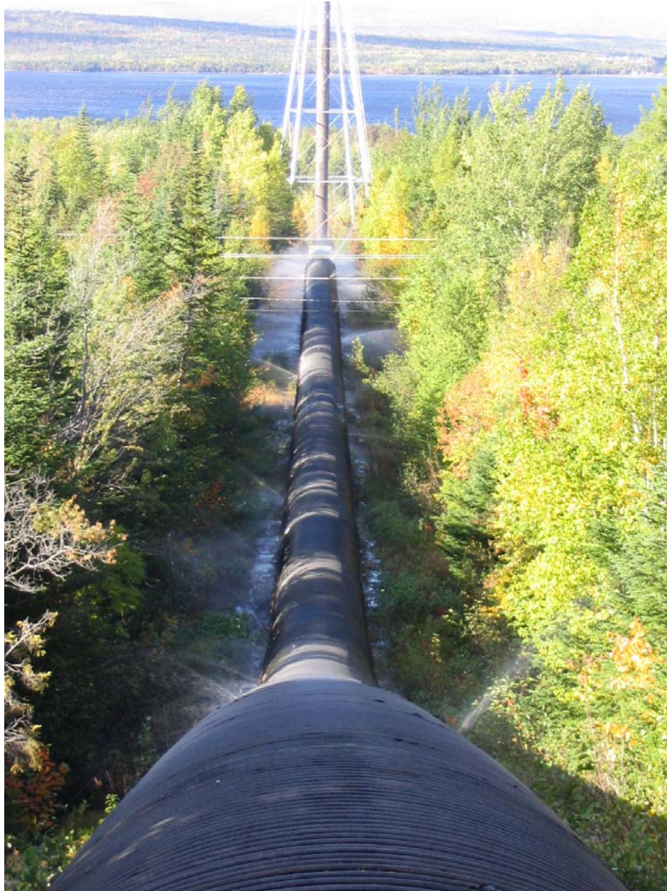
Figure 7: Lower Section of Woodstave Penstock
