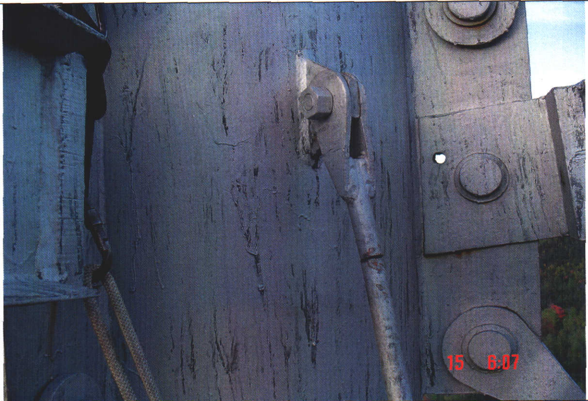
5. External riser stabilizer rod connection to leg #4 at EL.140'. Weld failure on connection to riser.
