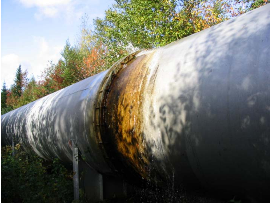
Figure 18: Leakage at Expansion Joint
