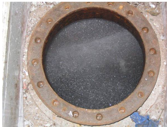
Figure 7 – Scroll Case Access Hatch
