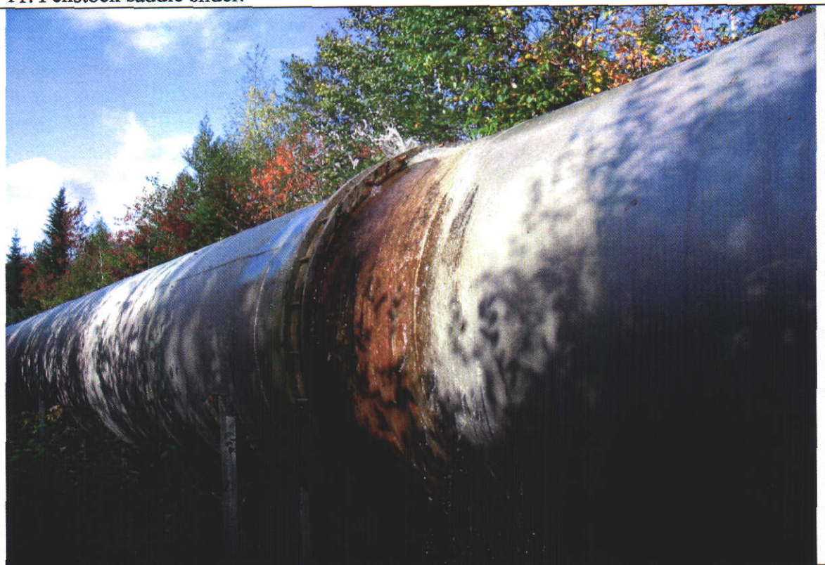
12. Expansion joint #2 leaking at top.
