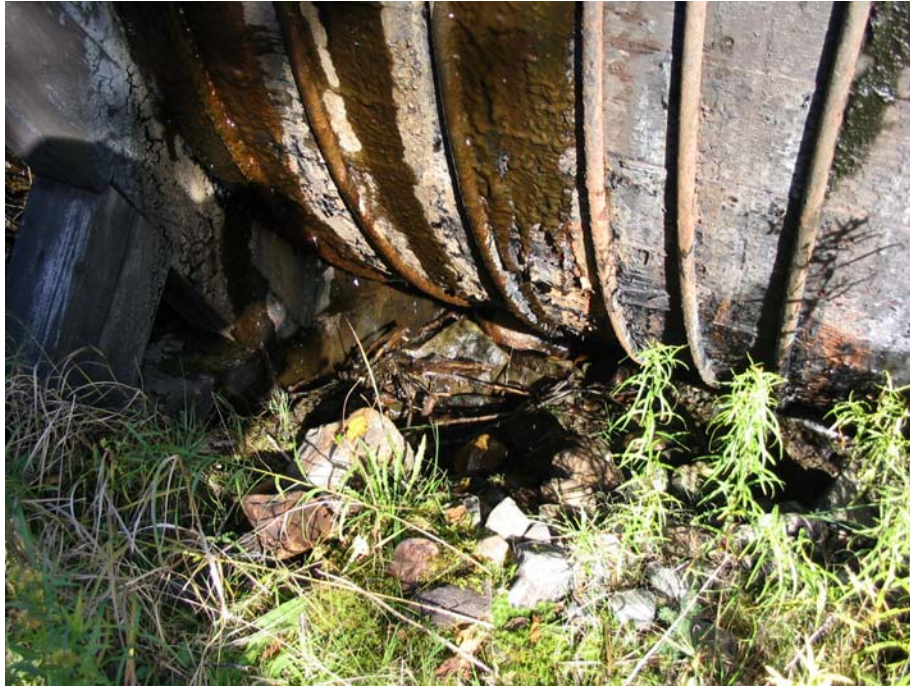
Figure 14: Settlement of Penstock into Bedding
