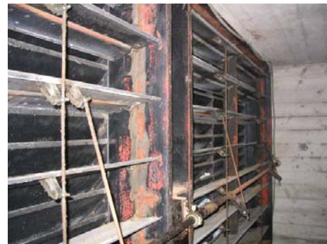
Figure 18– Air Inlet Dampers
