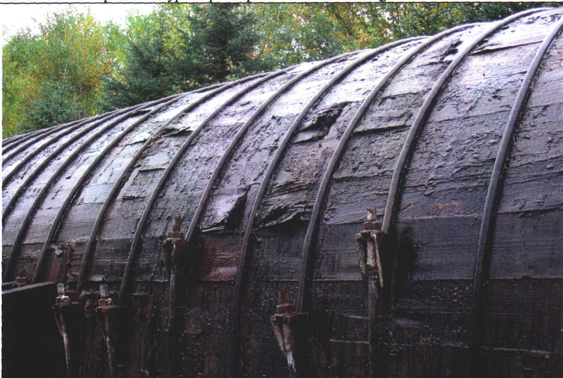
16. Wood stave penstock surface condition.
