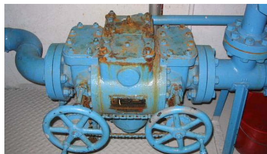
Figure 14 – Twin Strainer
