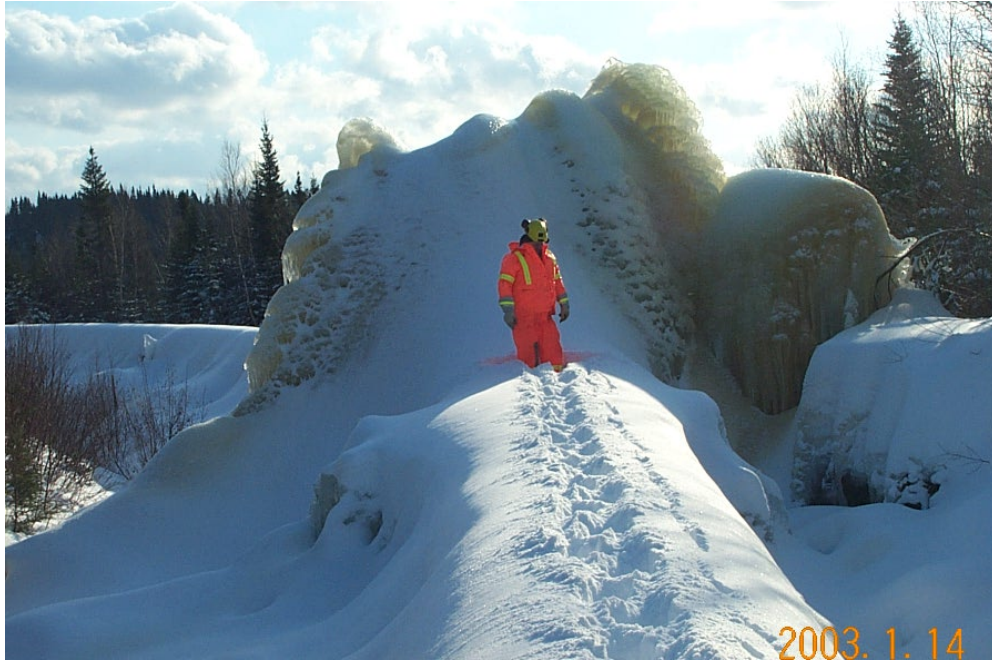
Figure 8: Ice Build-up on Penstock due to Water Leakage
