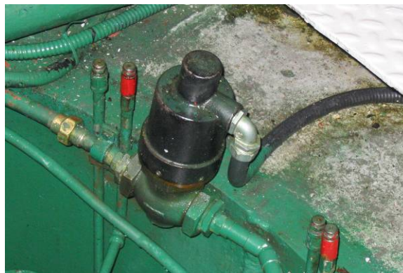
Figure 15 – Solenoid Valve
