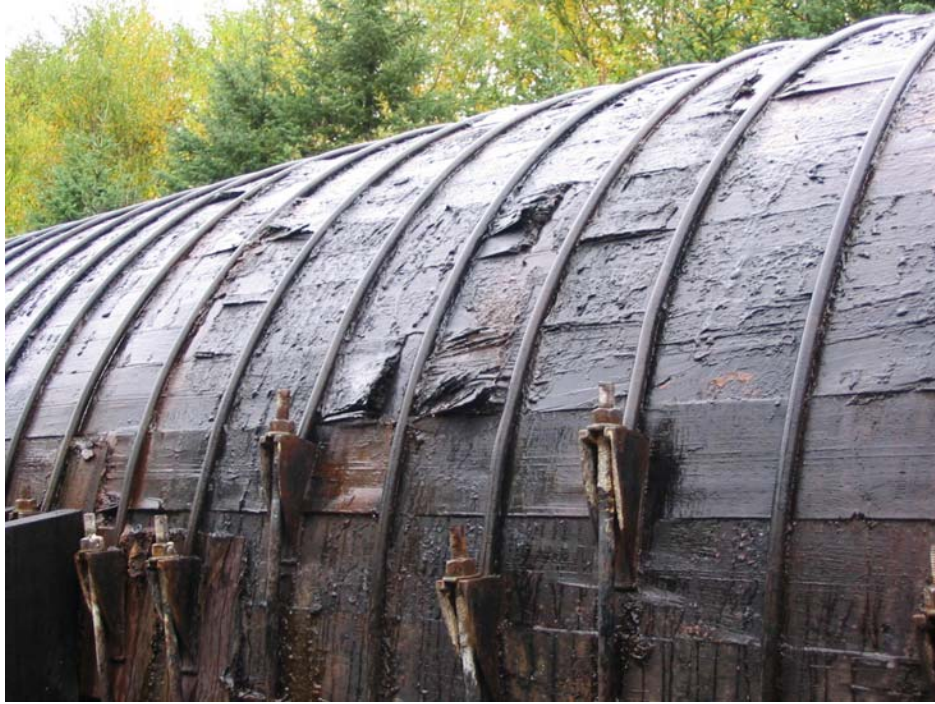
Figure 12: Crushing of Woodstaves
