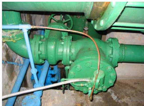
Figure 3 - Bypass Valve
