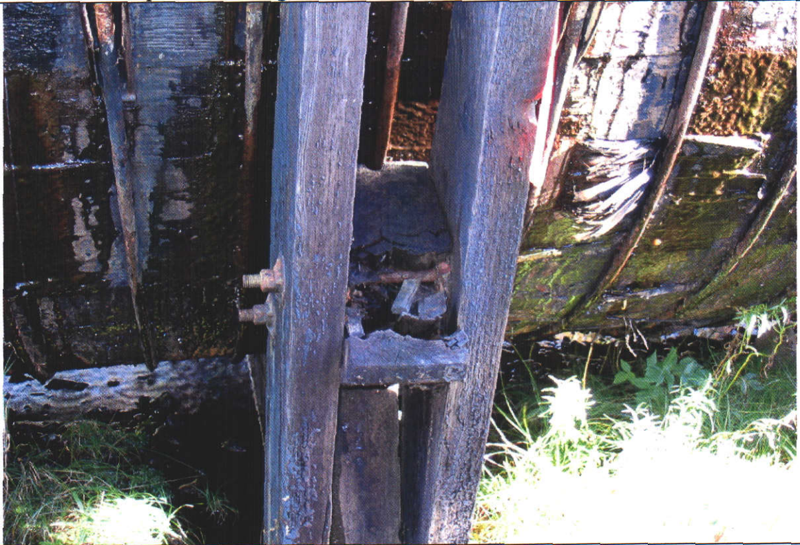
20. Wood stave penstock saddle deterioration.
