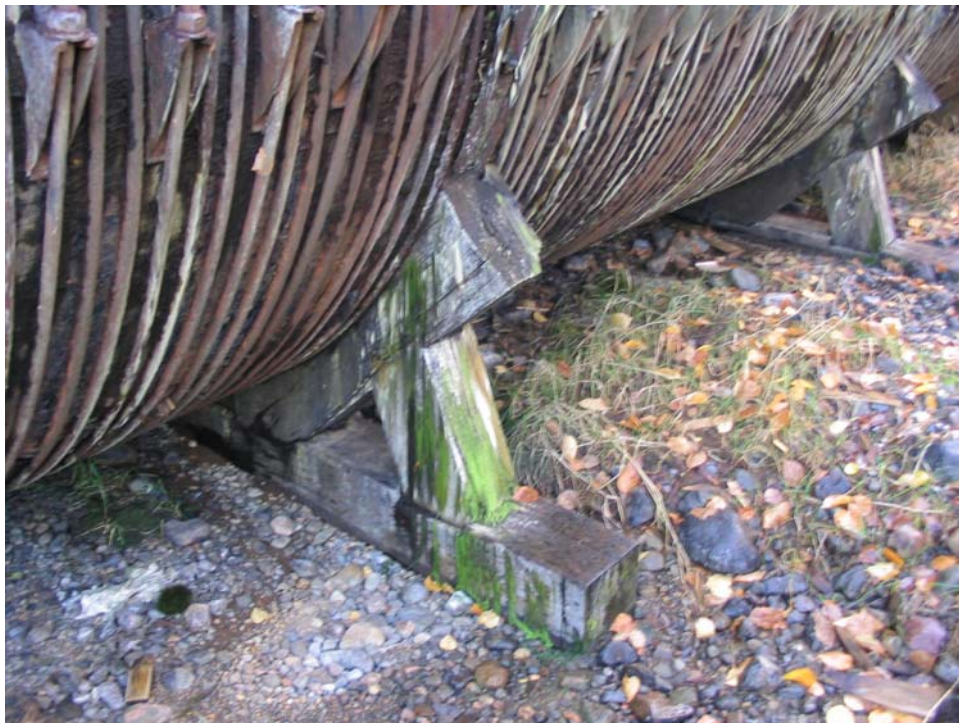
Figure 11: Settlement of Penstock Supports
