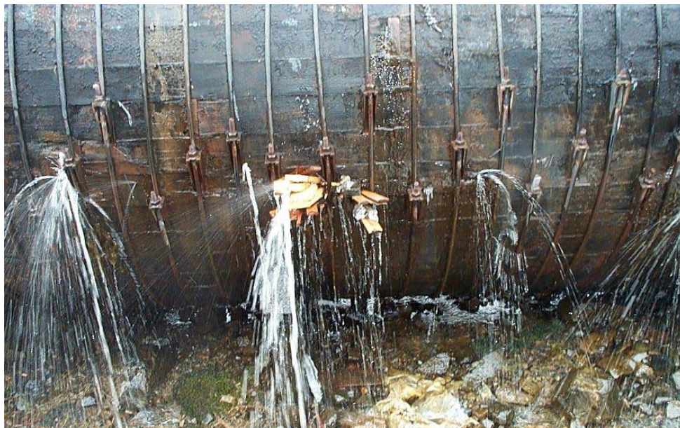
Figure 17: Leaking Woodstaves
