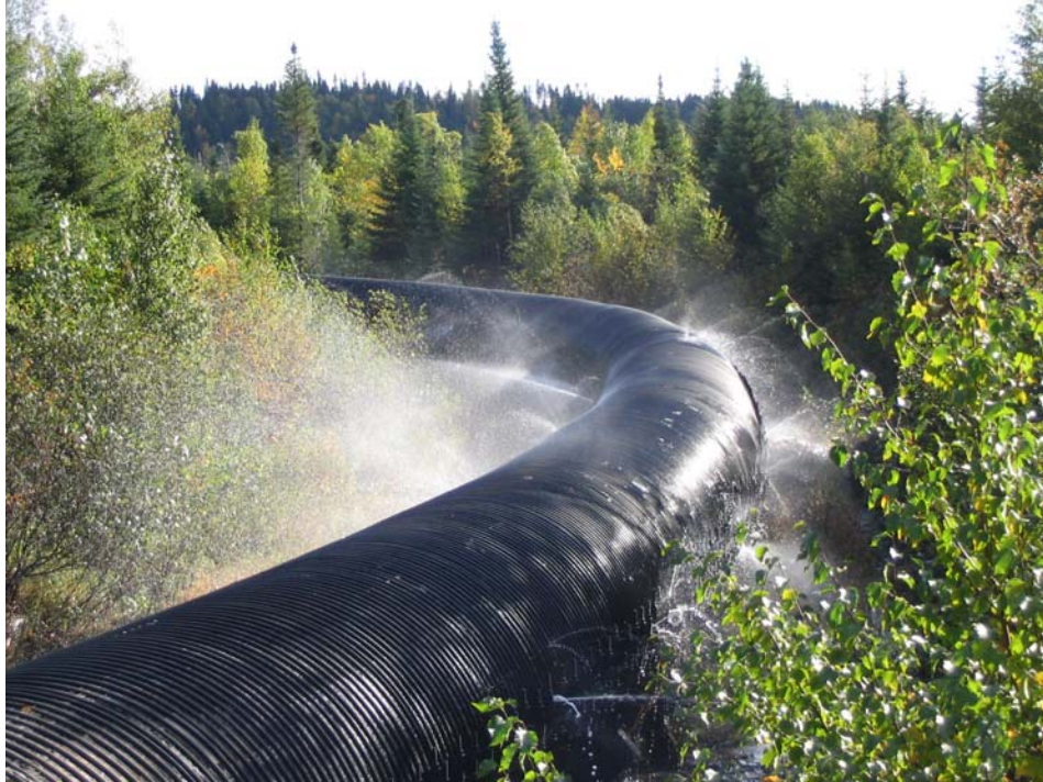
Figure 5: Water Leakage from Penstock
