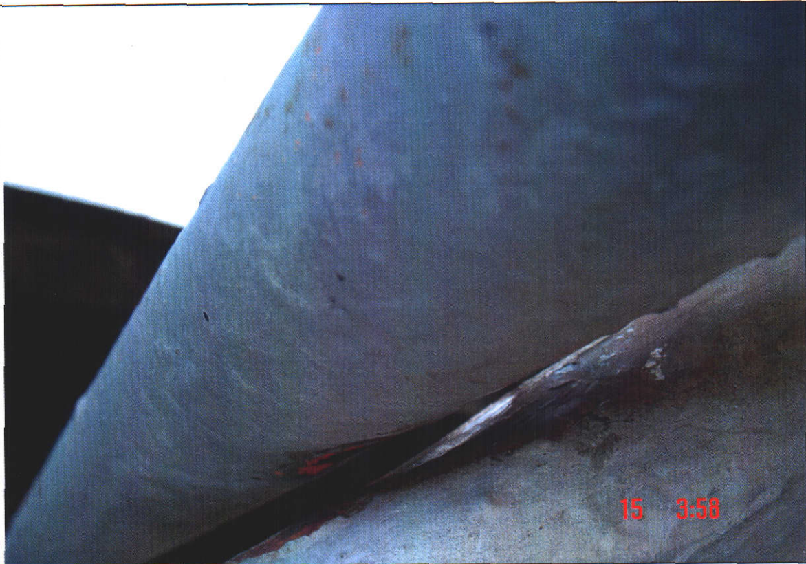
3. Wear of rod bracing.
