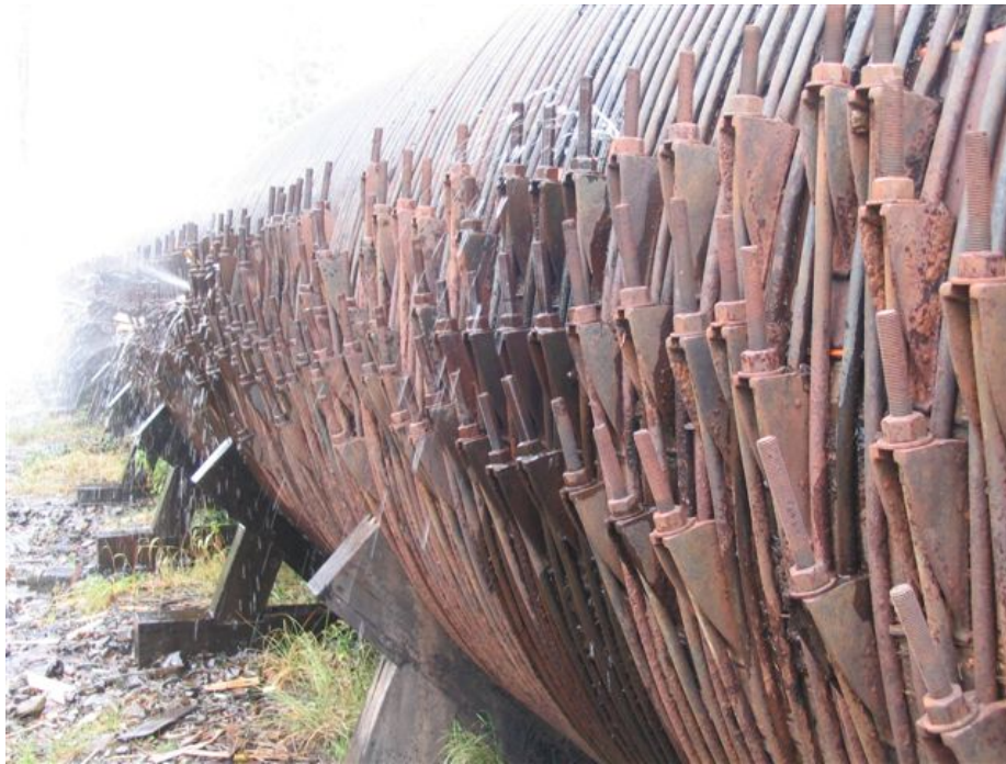
Figure 16: Leakage at Lower Section of Penstock
