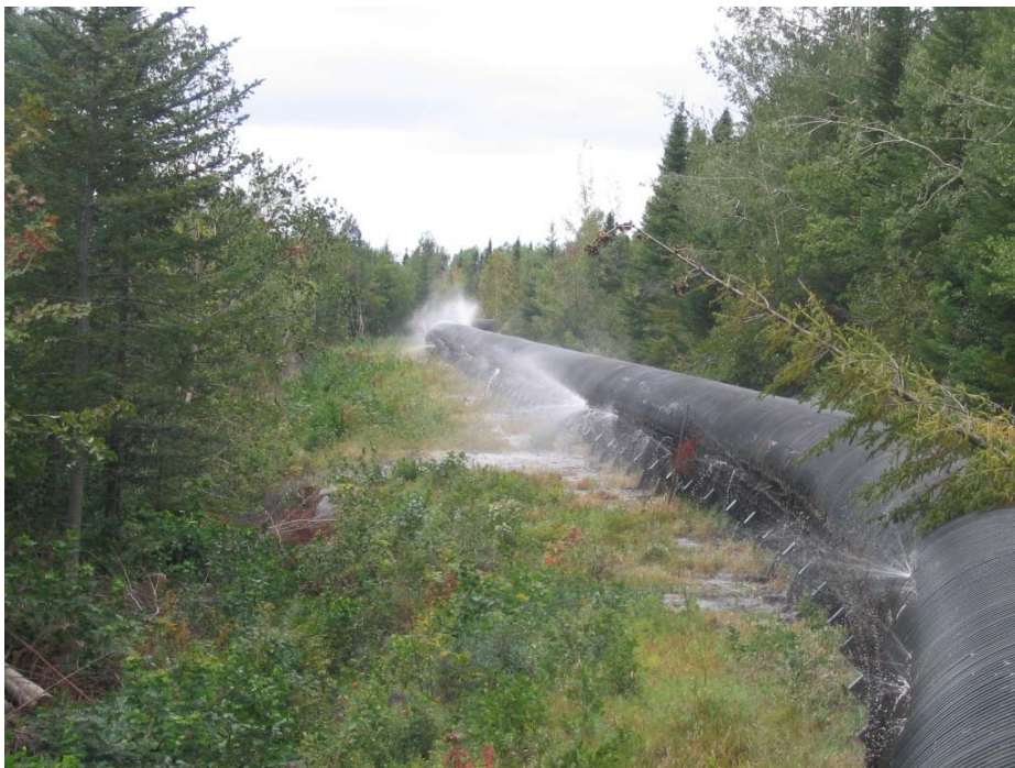
Figure 4: Water Leakage from Penstock
