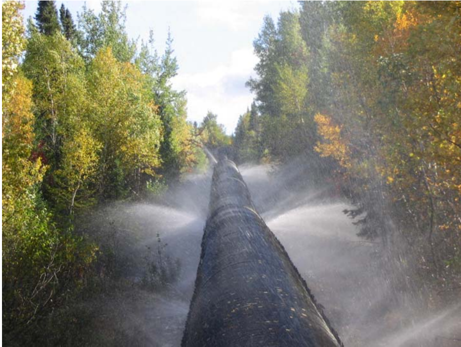
Figure 3: Water Leakage from Penstock
