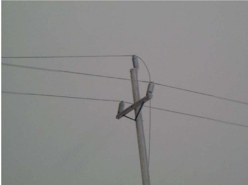
Figure 7 - Broken conductor - ice build up December 2003 110L
