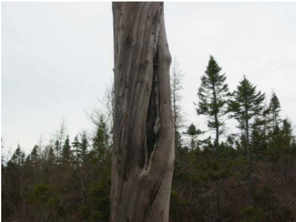
Figure 7 Deteriorated pole 407L
