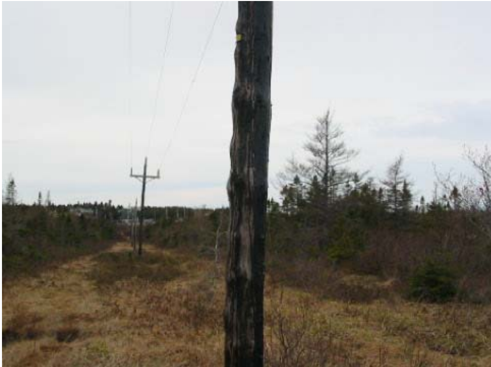
Figure 6 Deteriorated pole 407L
