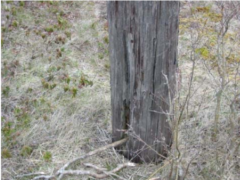
Figure 2 Deteriorated pole 407L
