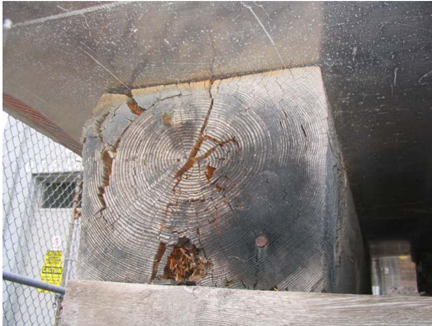
Picture #3 Topsail T1, rotting timber foundation
