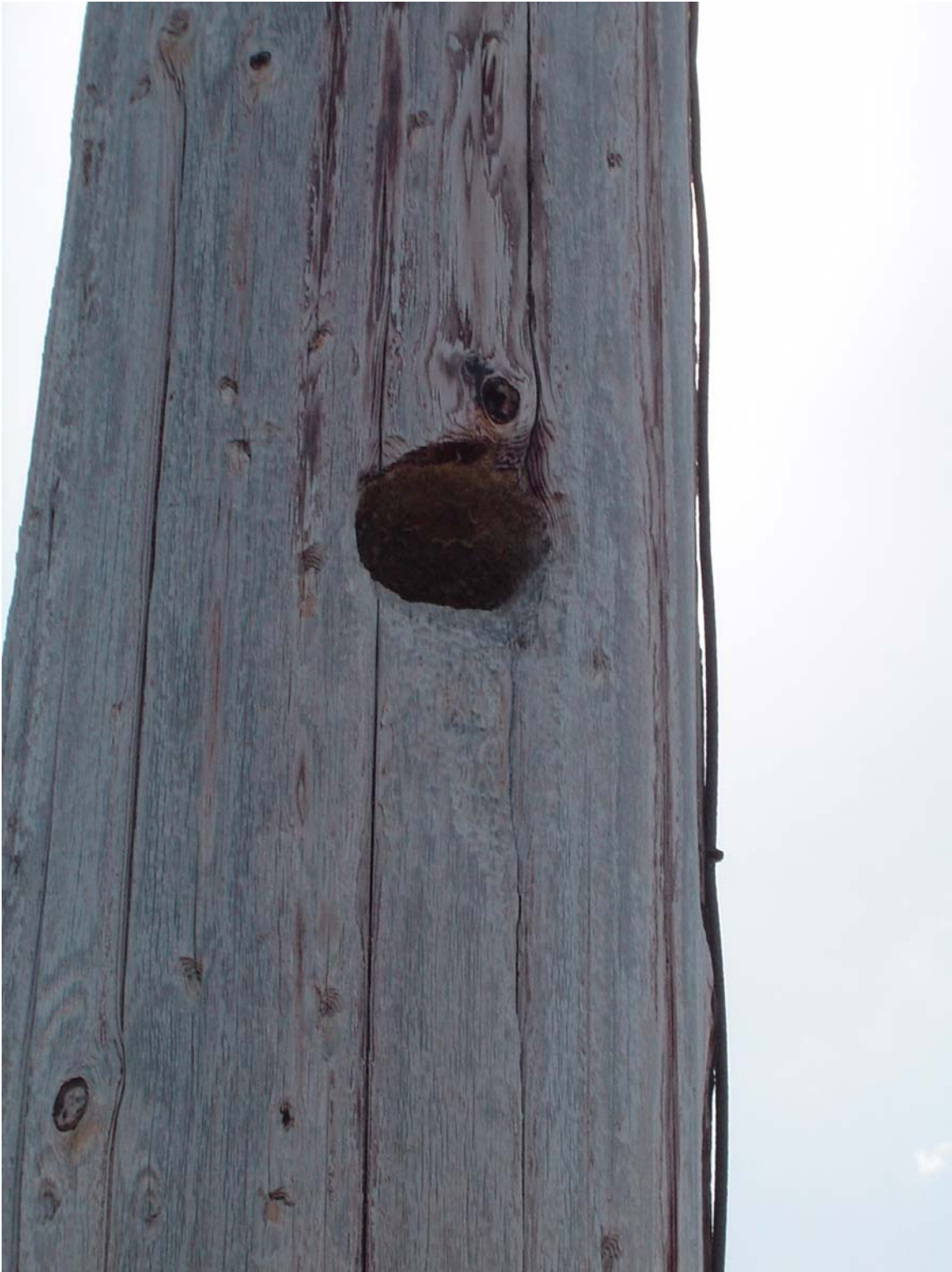
Figure 5 Woodpecker damage 43L
