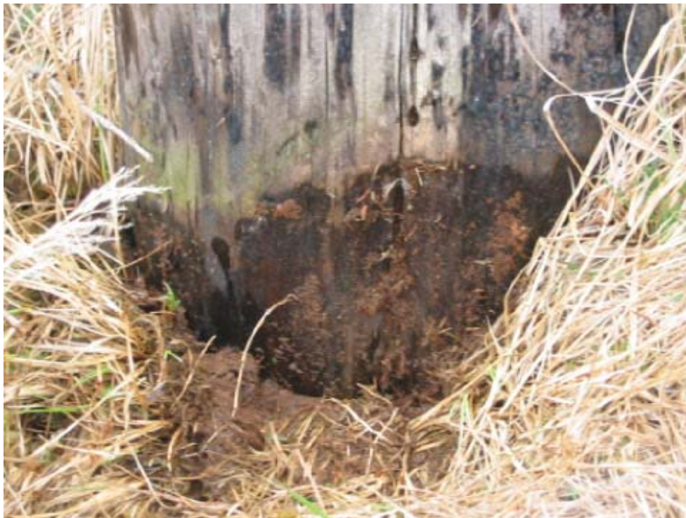
Figure 5 Ground line decay 407L
