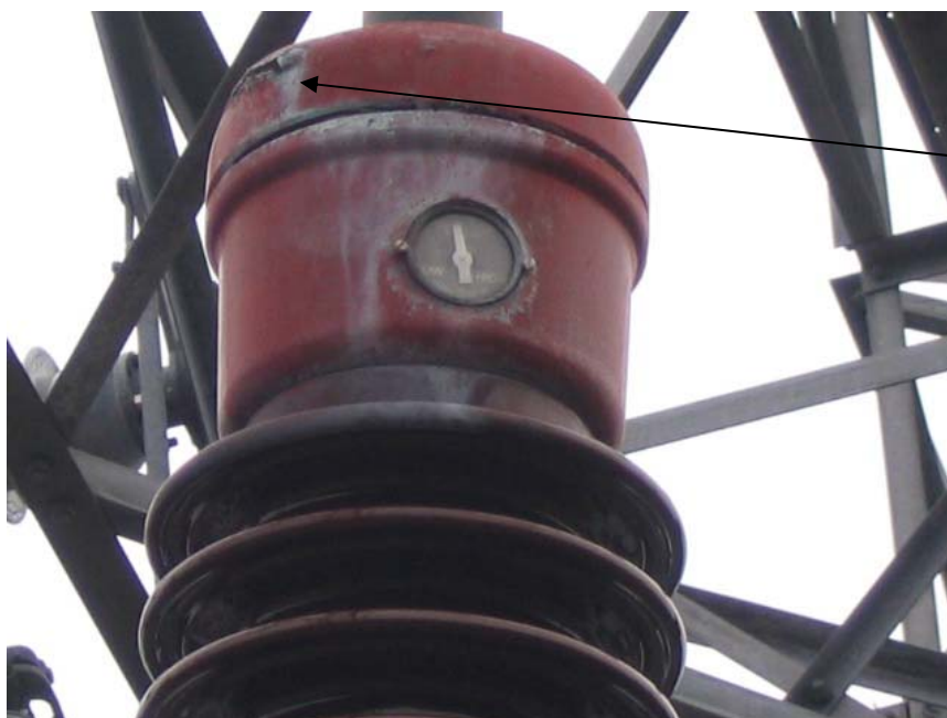
Picture 2 Bushing Deterioration
