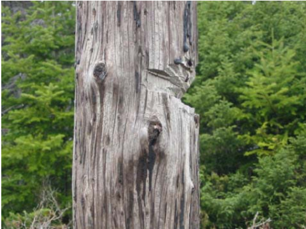
Figure 4 Vandalized pole 407L
