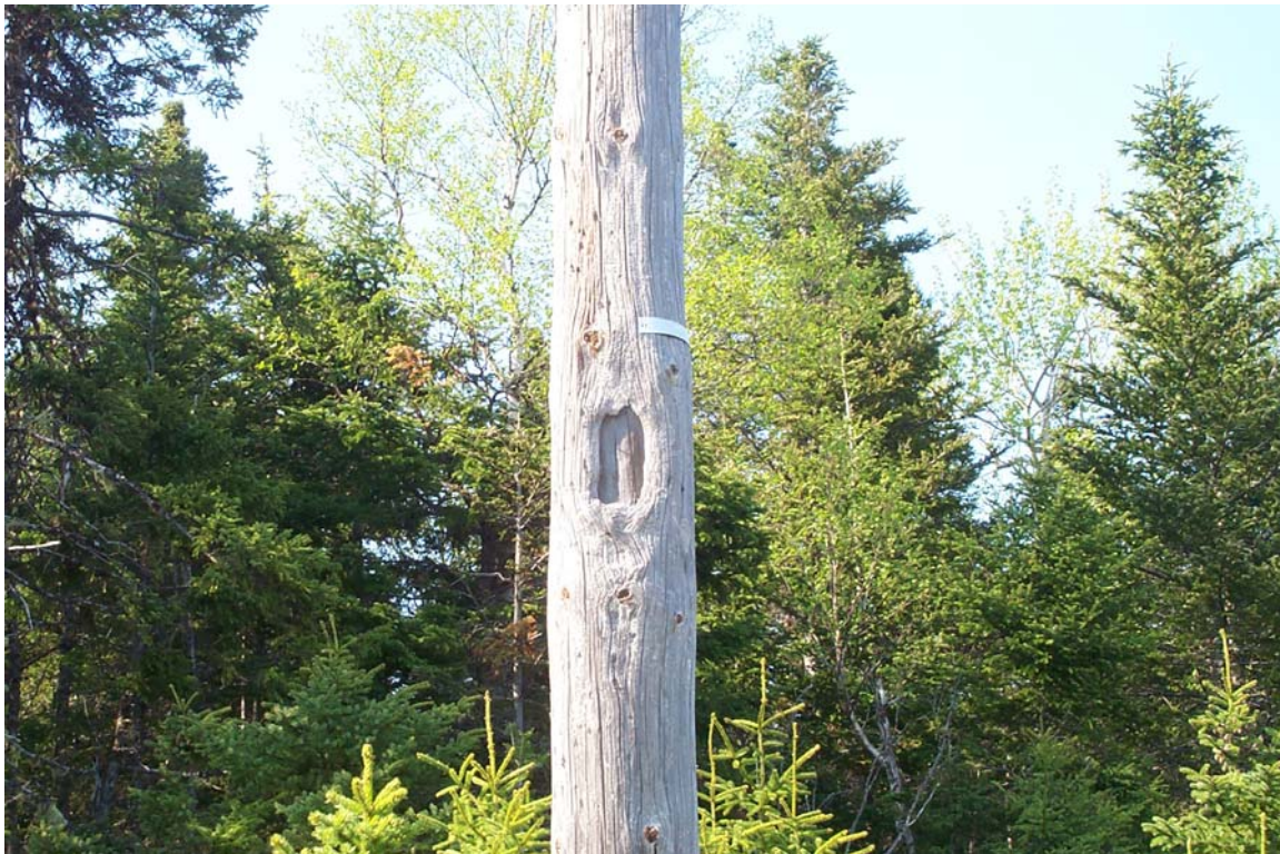
Figure 4 Deteriorated pole 110L
