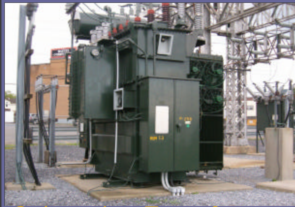
Substation Transformer
