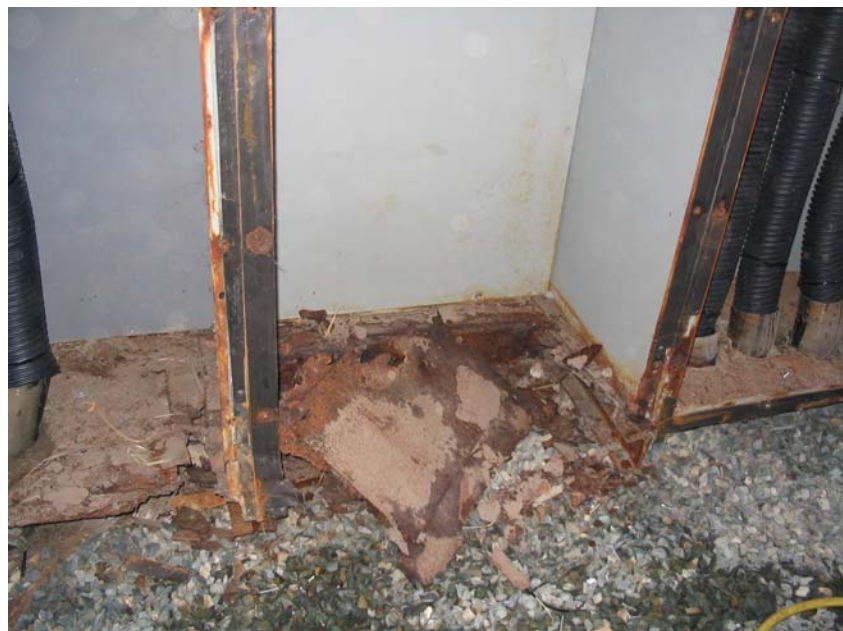
St. John's Main Substation Deteriorated Metal Clad Switchgear Picture #2
