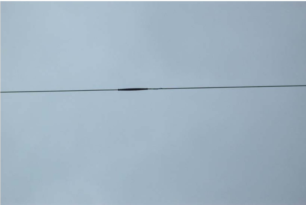
Another location with “Bird Caging” with a splice in the conductor. Picture #2
