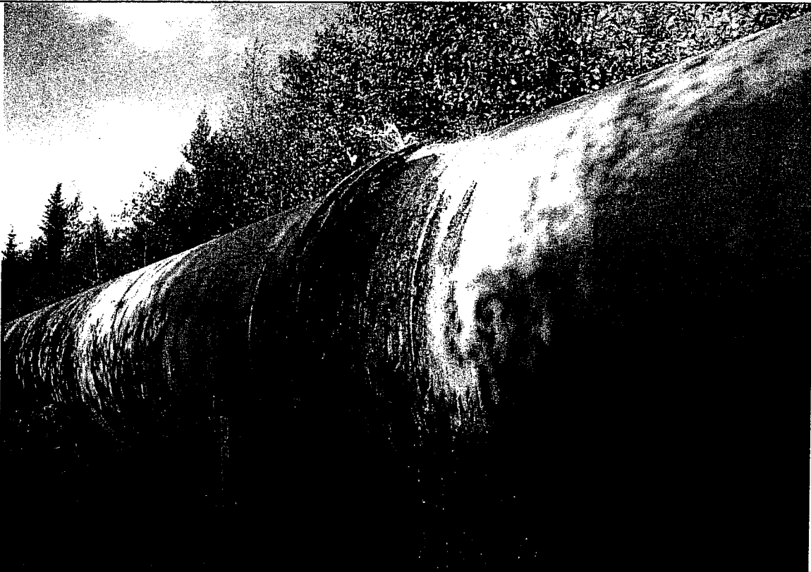
12. Expansion joint #2 leaking at top.
