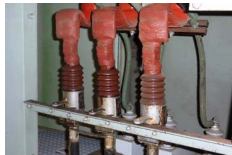
Unit #1 Generator Cable Terminations
