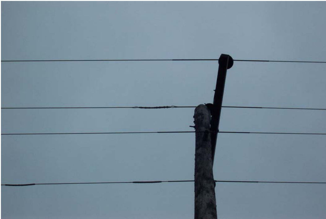
Center Phase has “Bird caging” along old splice. Note previous repair on outside phase. Picture #1
