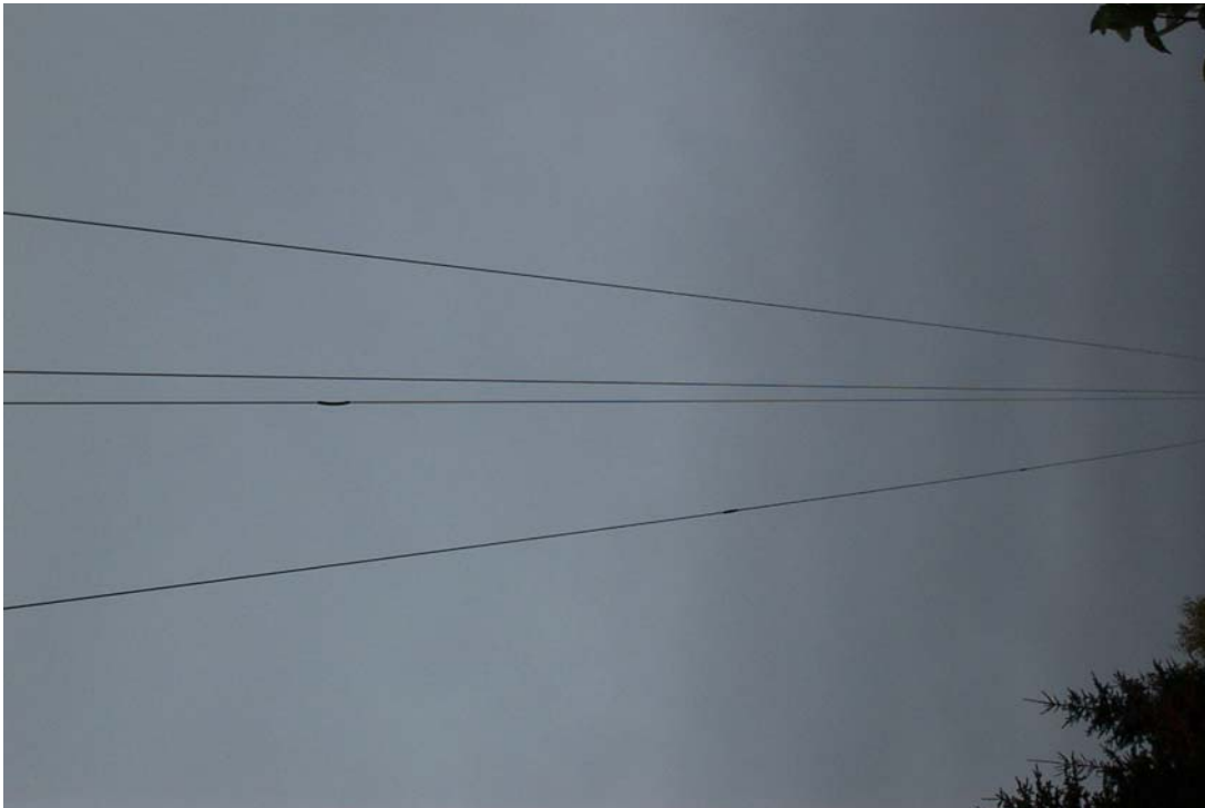
Another Span with 3 splices in the #2 ACSR. Picture #3
