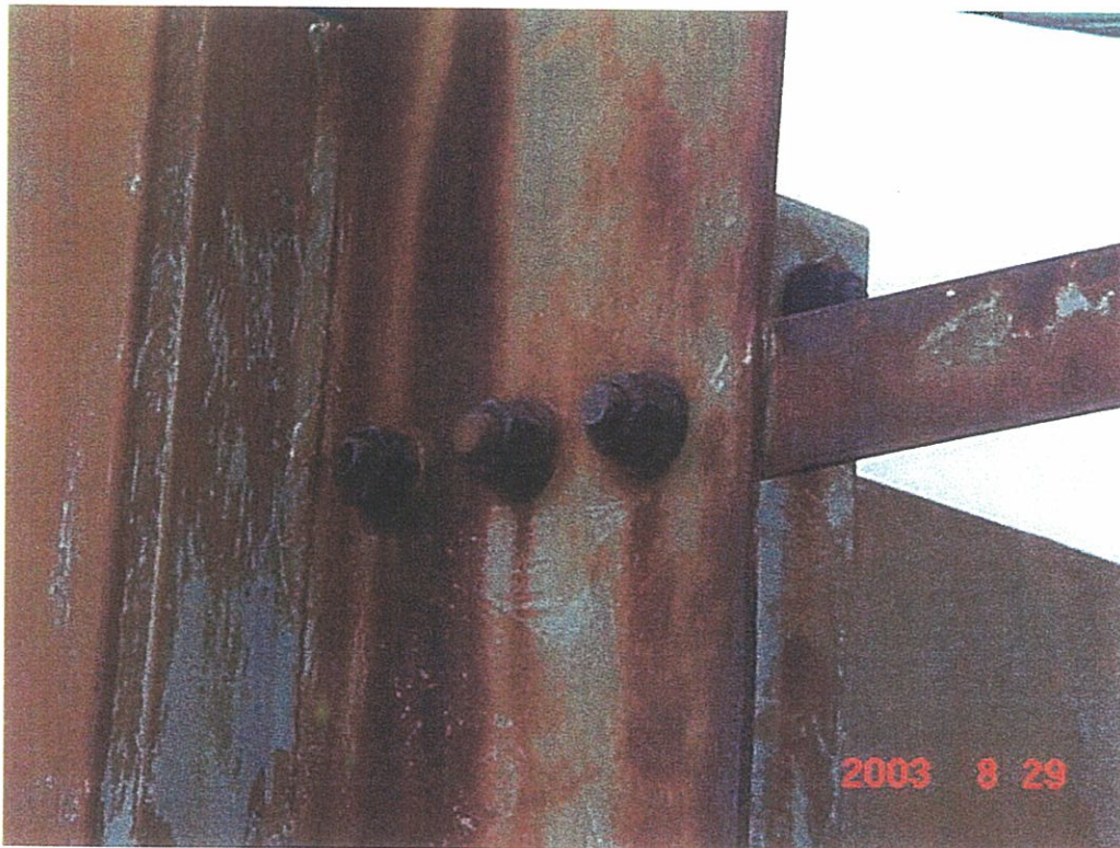
Take Off Tower for T1, bolted connection, leg to horizontal brace, light corrosion.
