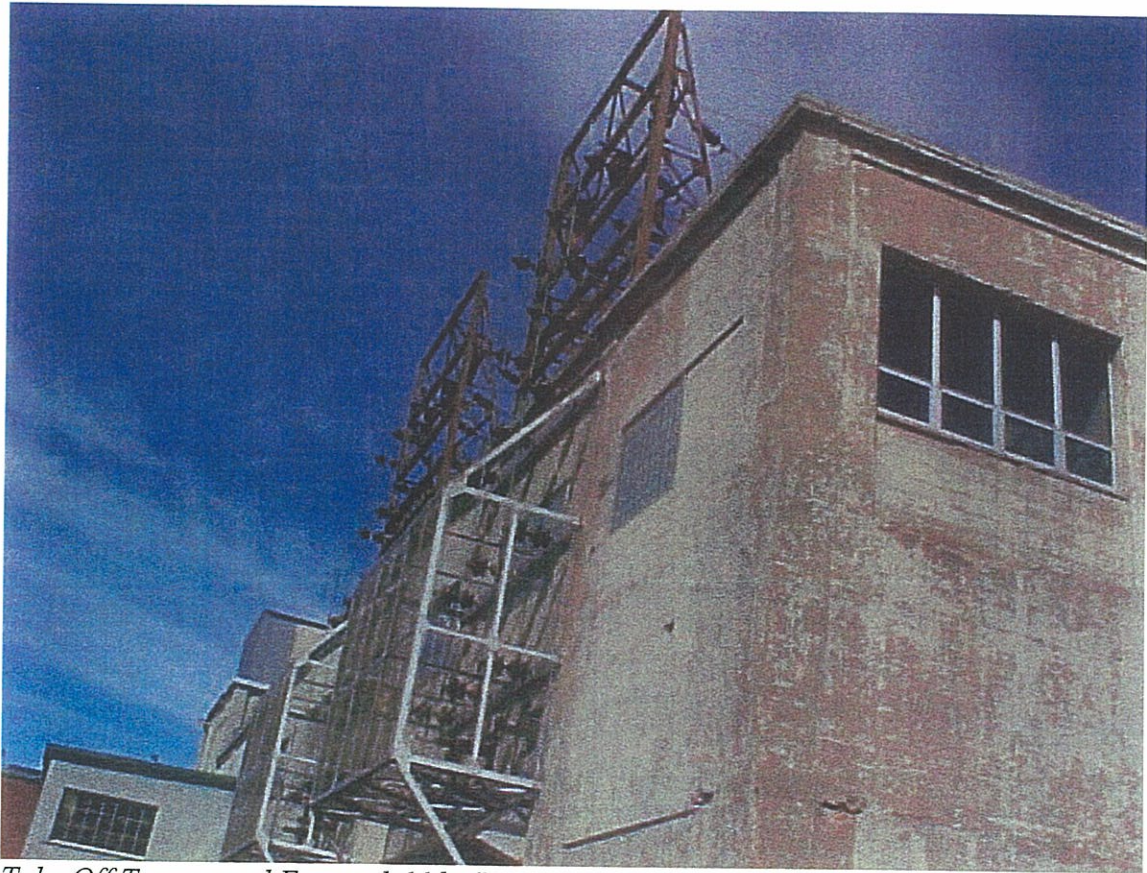
Take Off Towers and External 66 kv Bus associated with the Frequency Converter at Corner Brook Pulp and Paper.
