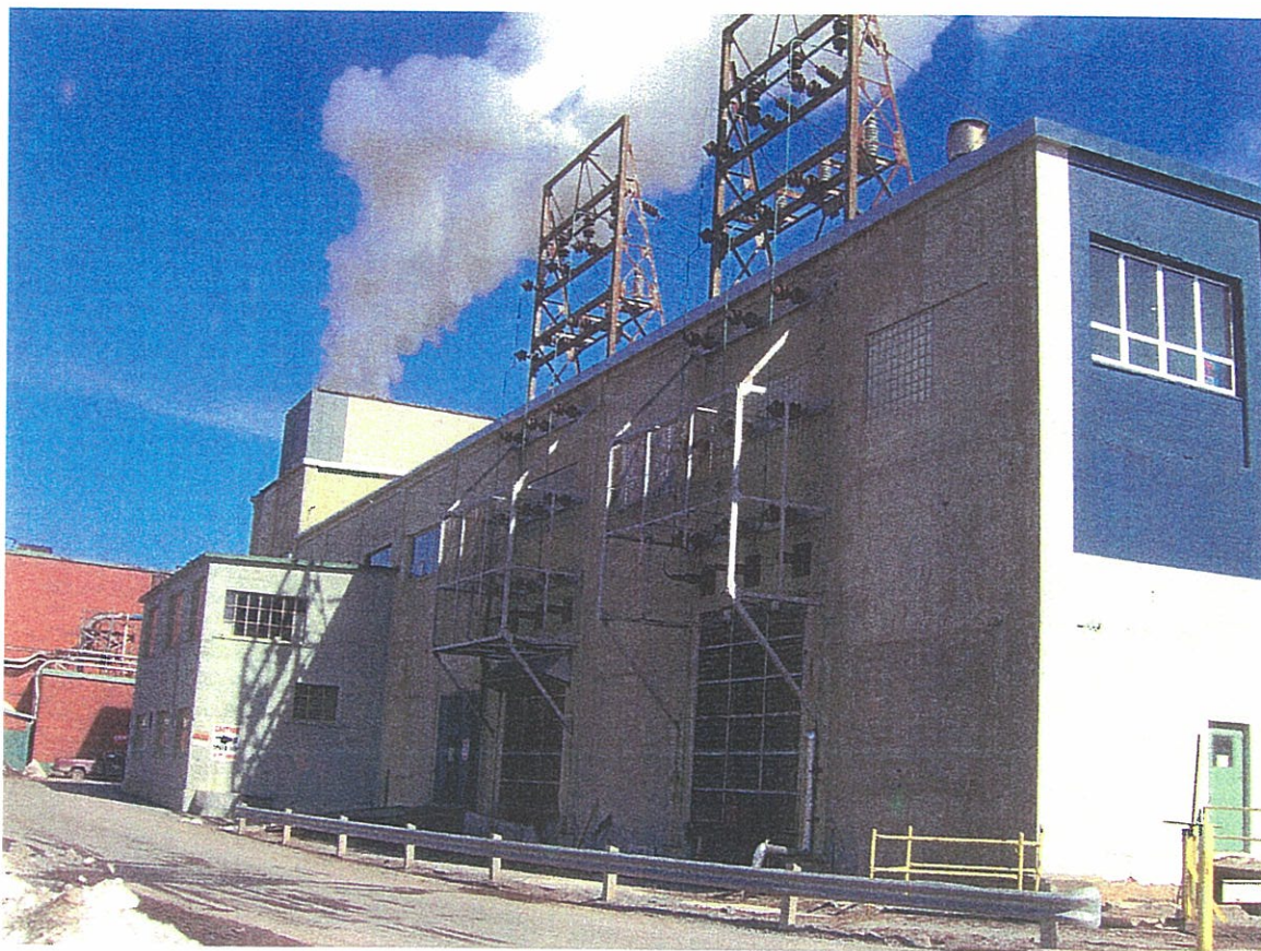
Figure 13 – Towers and External 66 kV Bus (2005)
