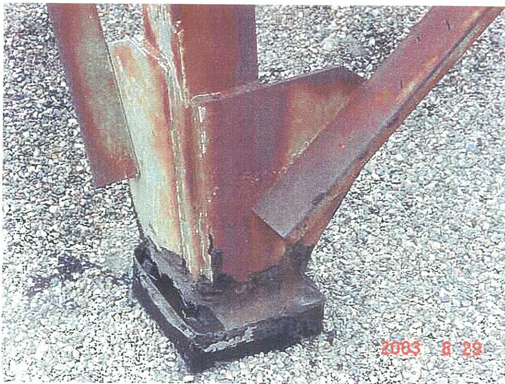
Take Off Tower for T2, leg anchor, light corrosion and mild pitting.
