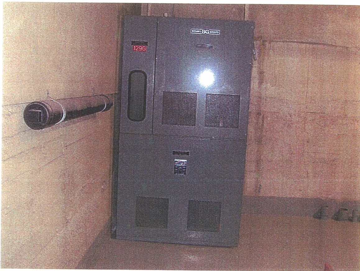
Figure 7 – Neutral Grounding Transformer (2005)
