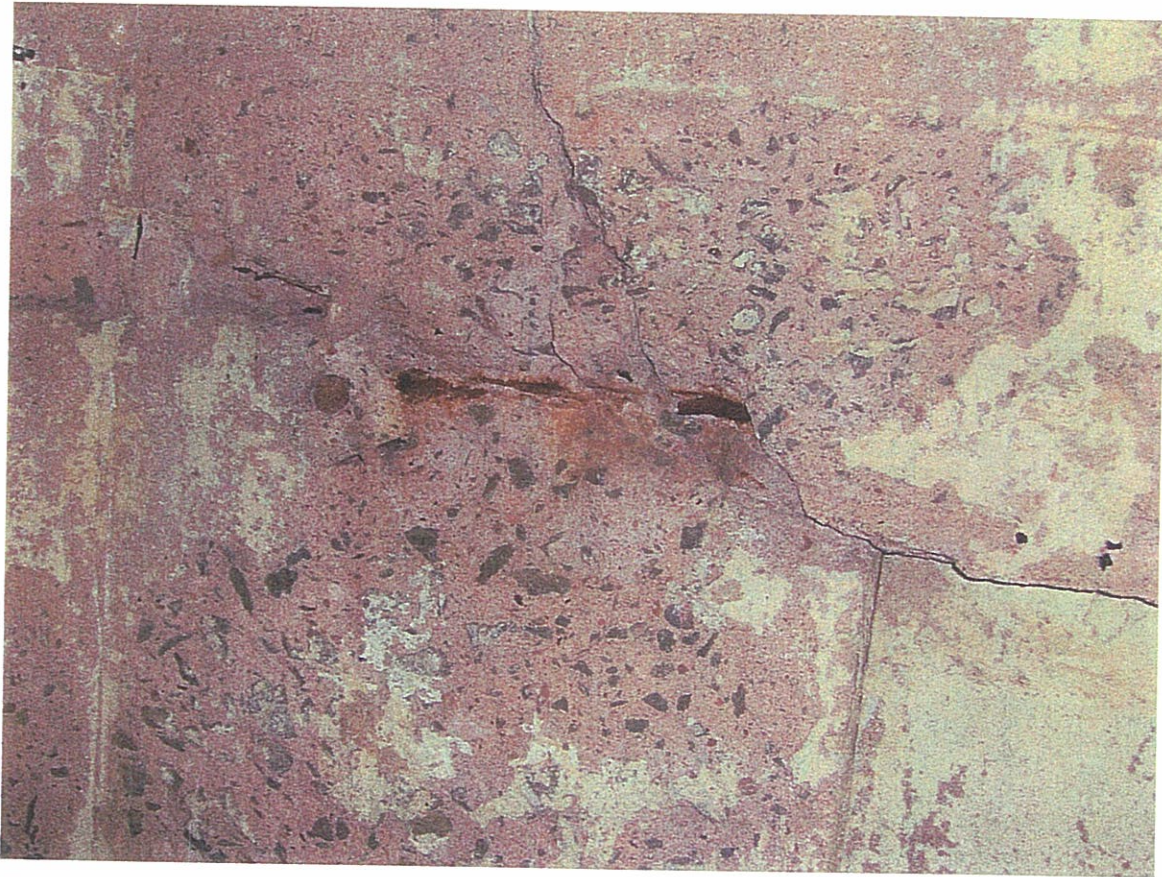
Figure 4 – Example of Crack in Wall (2005)
