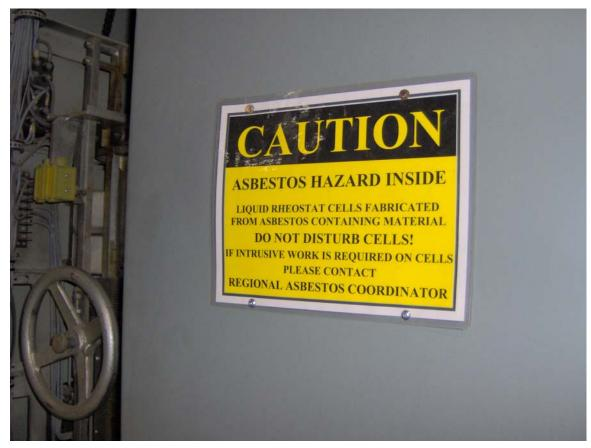
Figure 12 – Liquid Rheostat Asbestos Warning Sign (2005)
