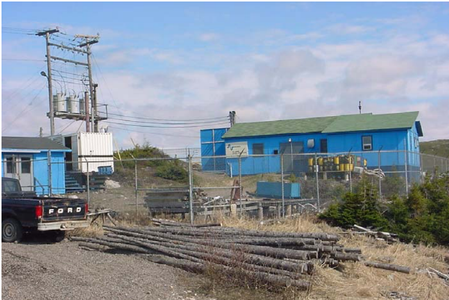
Photo #2 ---St Lewis Diesel Plant ---Note Extensions a) Office to the right and b) Storage Room to the left and rear.
