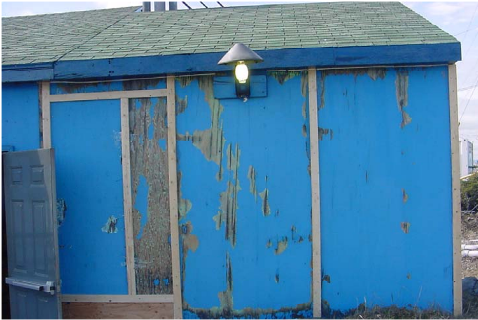
Photo #4 —St Lewis Plant—Rear View Showing Deterioration of Siding
