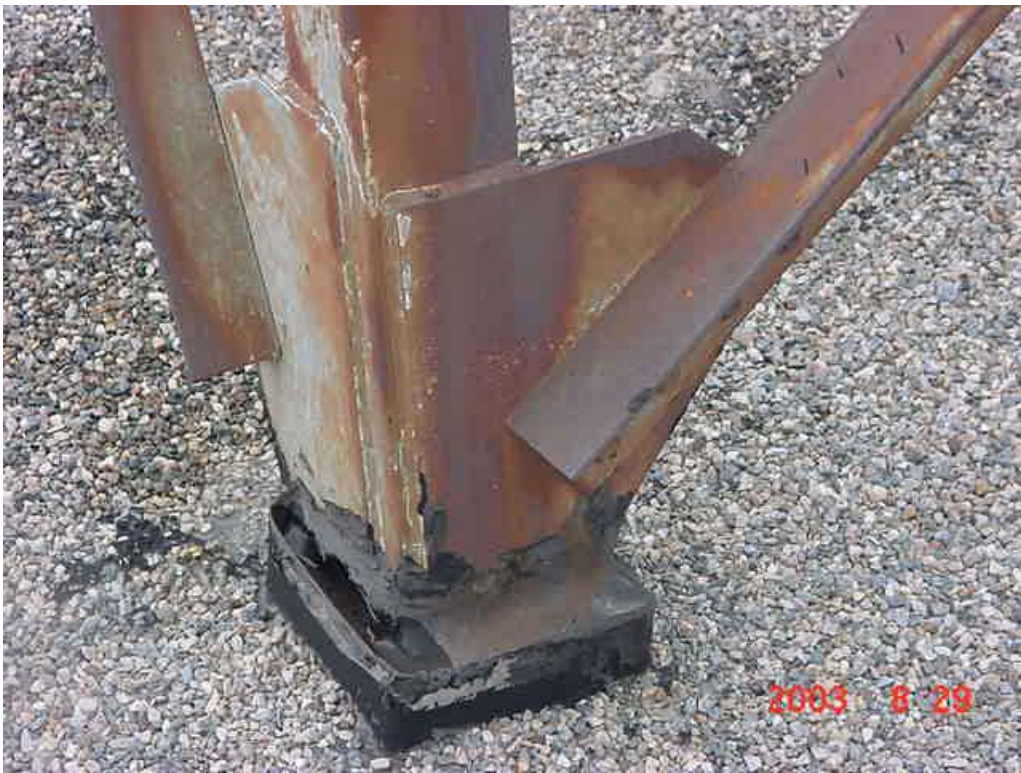
Take Off Tower for T2, leg anchor, light corrosion and mild pitting.
