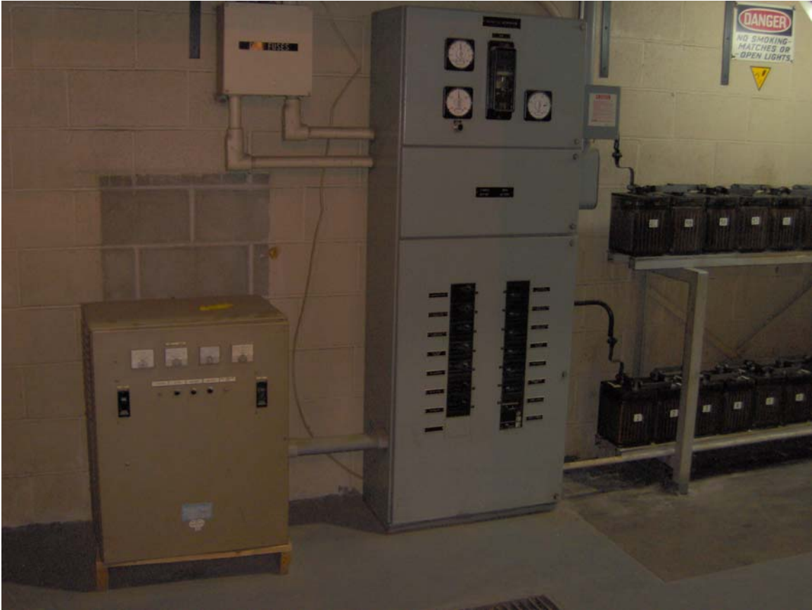
Figure 9 – Battery Charger & DC Panel (2005)
