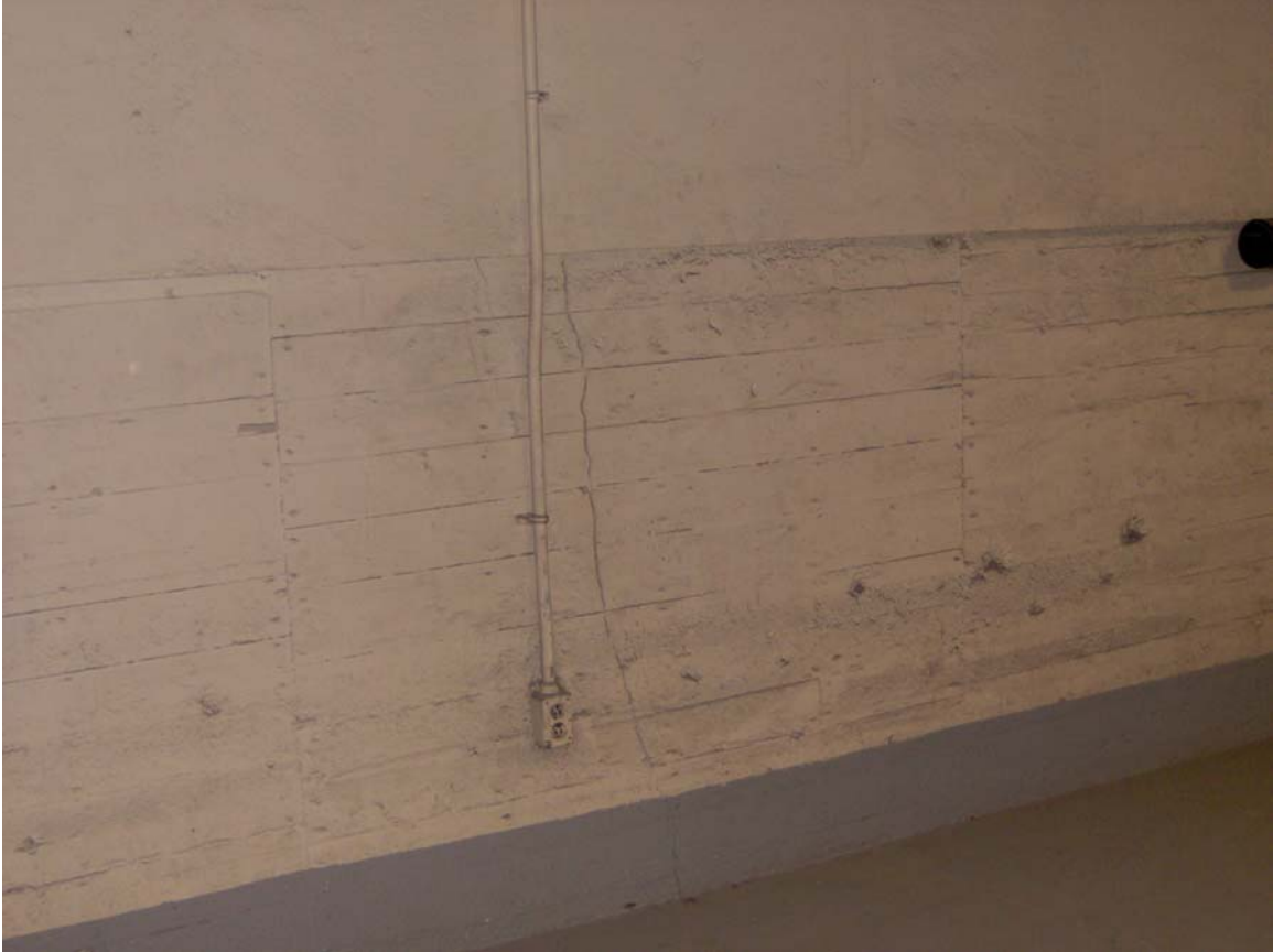
Figure 6 – Example of Crack in Wall (2005)
