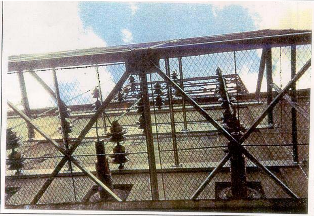
Photo 3: Damaged bushings outside the converter building - August 19, 1998
