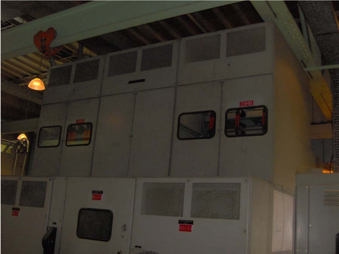
Figure 17 – Frequency Converter Switchgear (2005)
