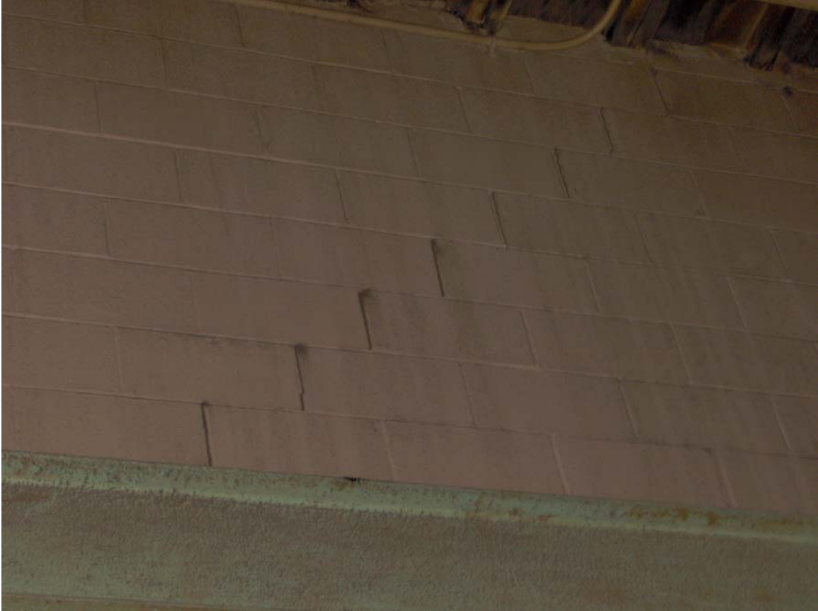
Figure 5 – Example of Crack in Wall (2005)
