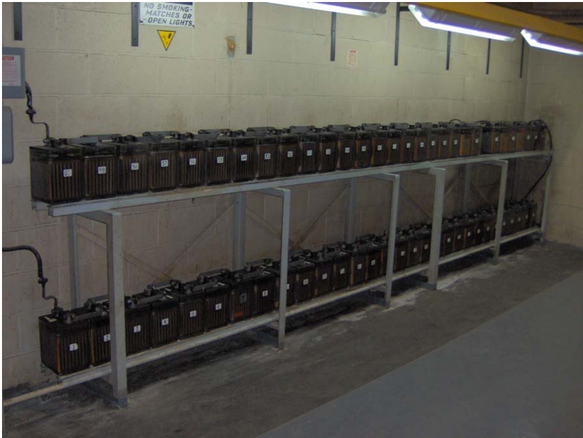
Figure 10 – Battery Bank {Scheduled For Replacement} (2005)
