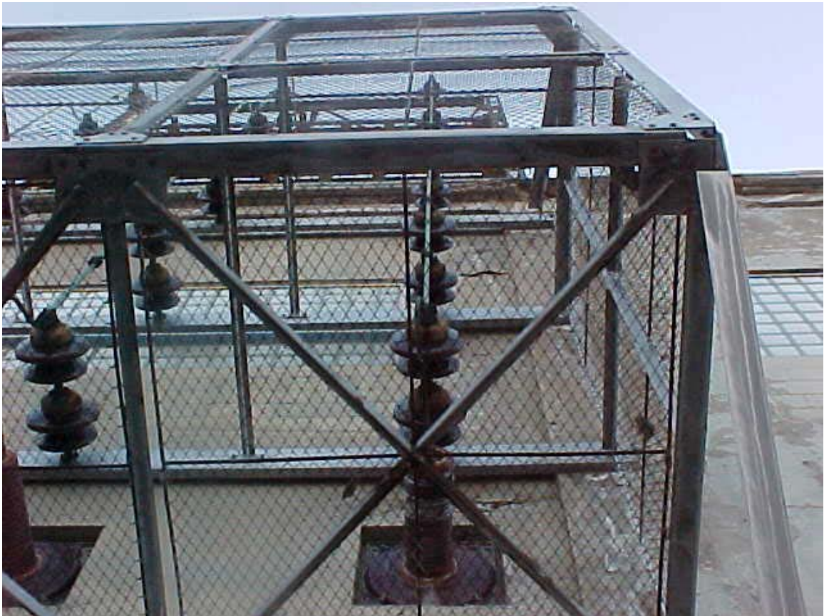
C.O.B. pincap insulators, 66 kv Bus CBPPL frequency converter building.
