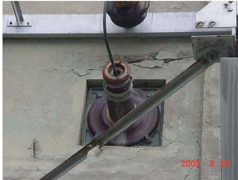
Damaged A phase entrance insulator.
