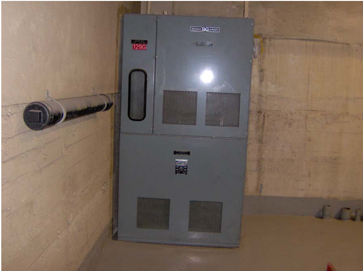
Figure 7 – Neutral Grounding Transformer (2005)
