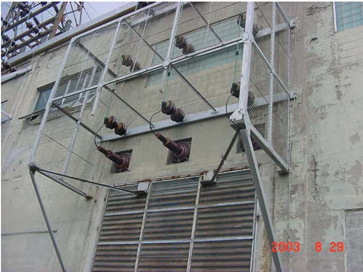
Protective Structure for T2 External 66 kv Bus, steel frame and wire mesh removed.
