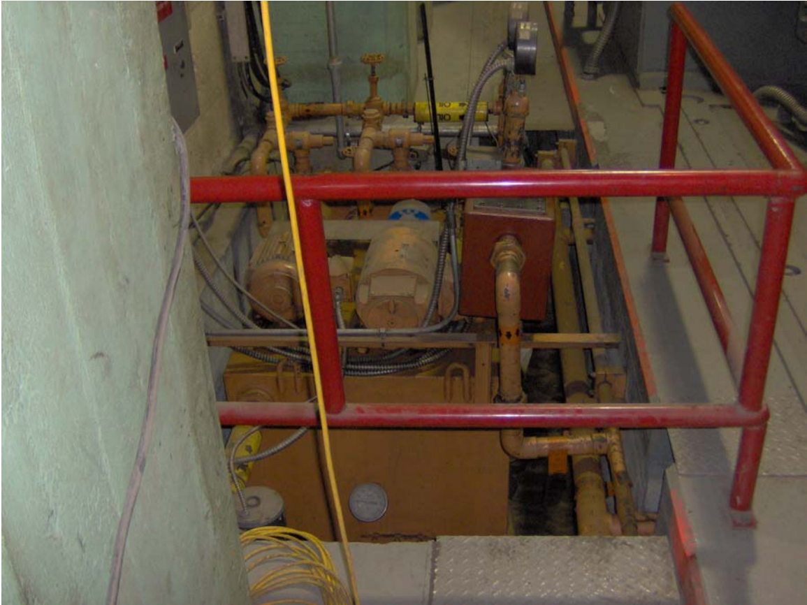
Figure 15– Main Lube Oil Pump (2005)
