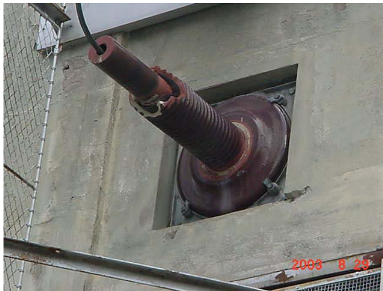
Damaged C phase entrance insulator.
