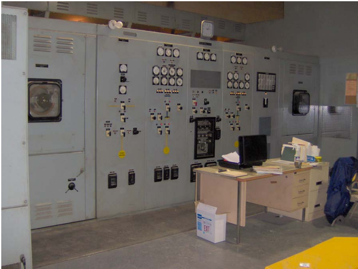
Figure 18 – Frequency Converter Switchgear (2005)
