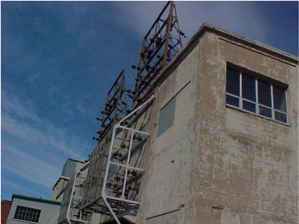
Take Off Towers and External 66 kv Bus associated with the Frequency Converter at Corner Brook Pulp and Paper.
