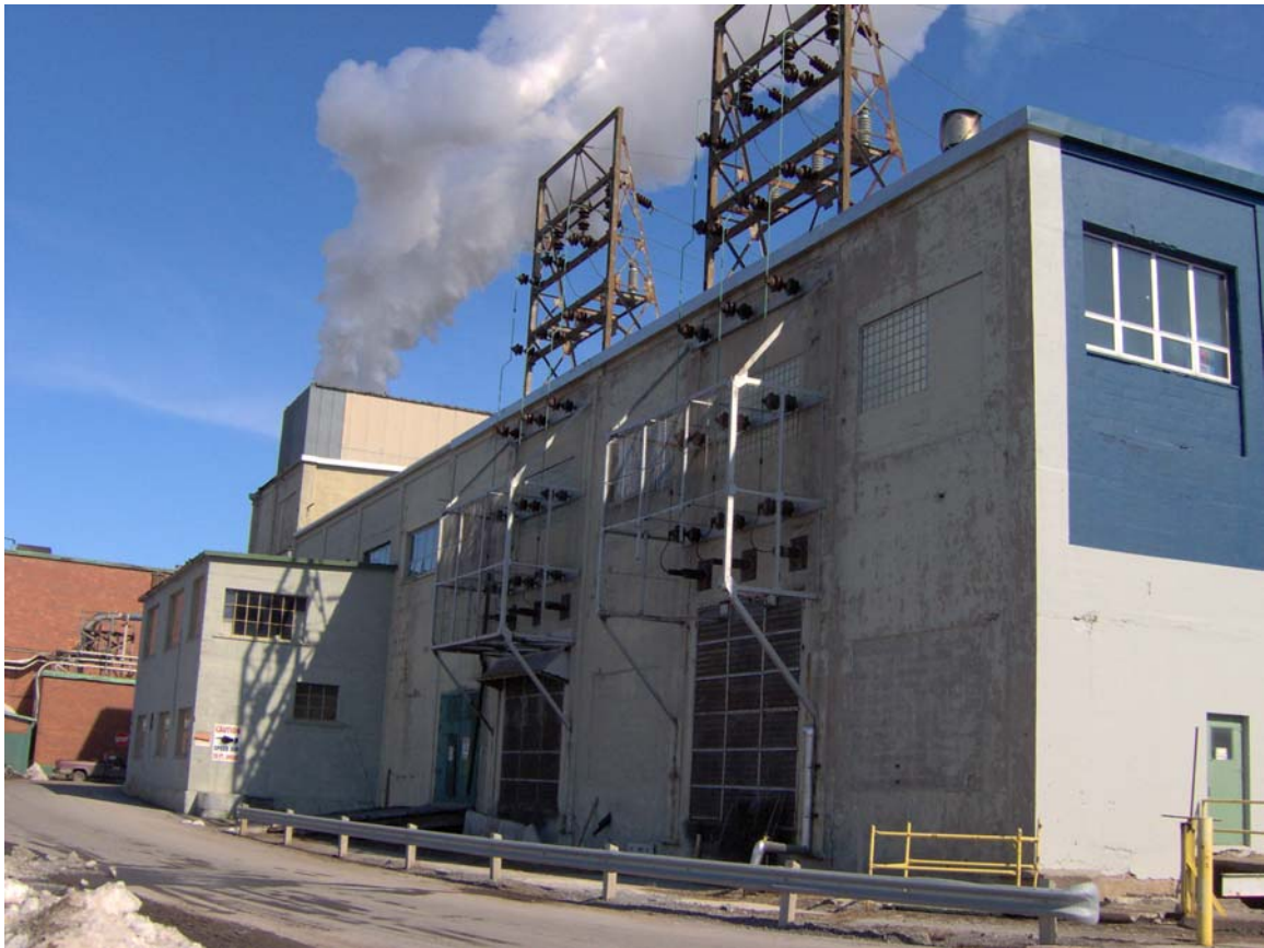
Figure 13 – Towers and External 66 kV Bus (2005)
