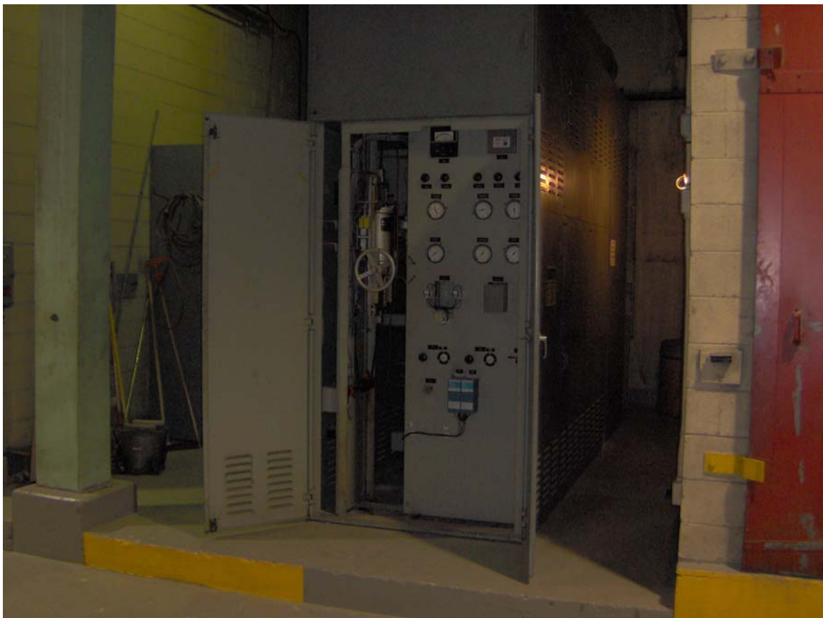
Figure 11 – Liquid Rheostat (2005)
