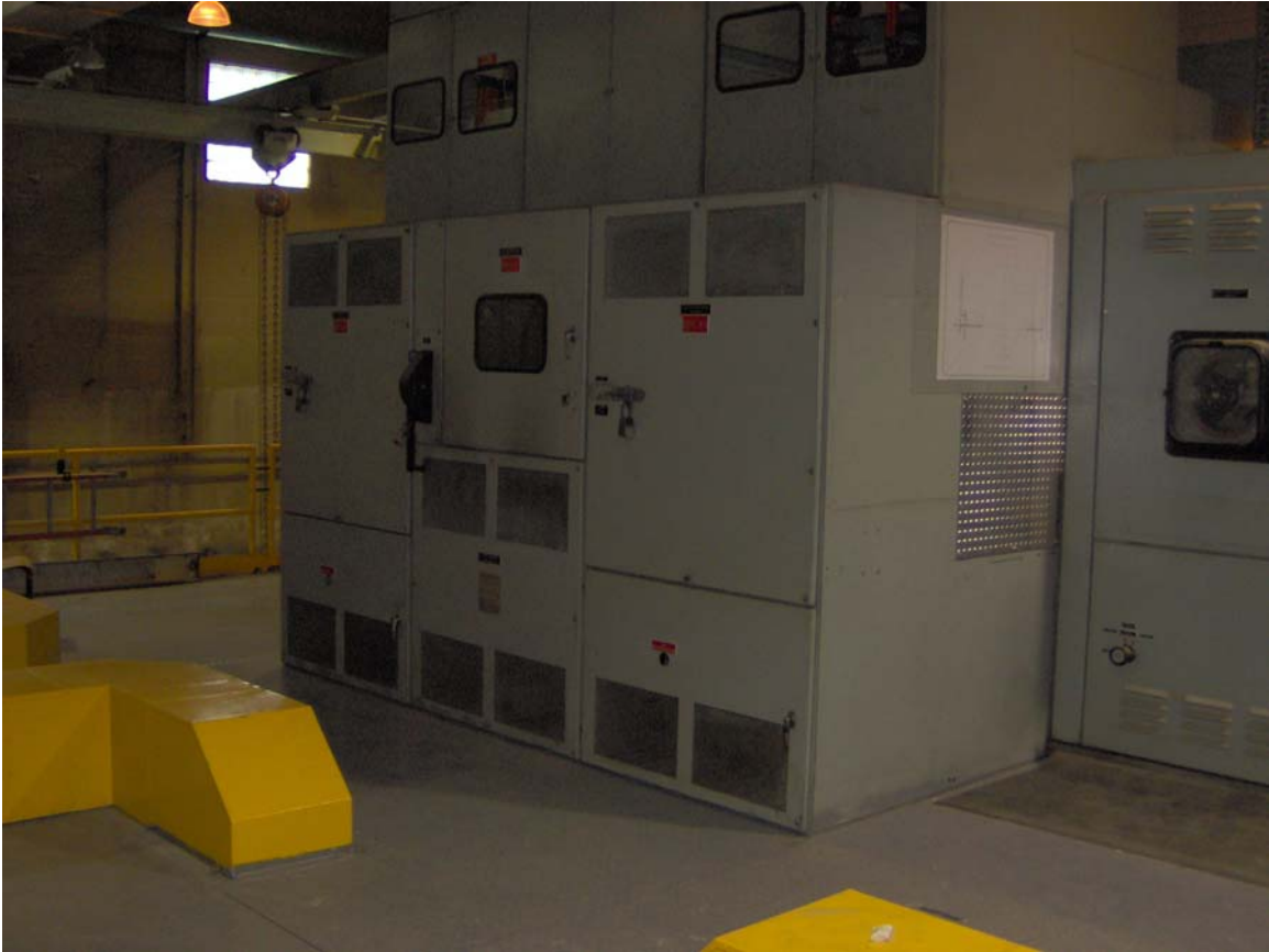
Figure 16 – Frequency Converter Switchgear (2005)
