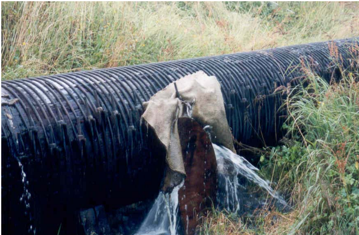
Photo #10: Water leaking from penstock, August 2000.
