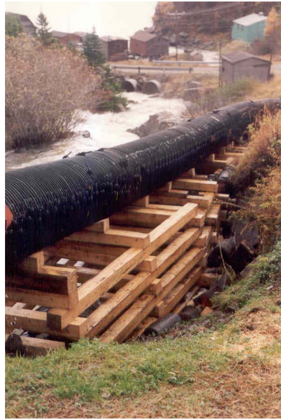
Photos #30 & #31: Timber support added under penstock after erosion of embankment, October 1992.
