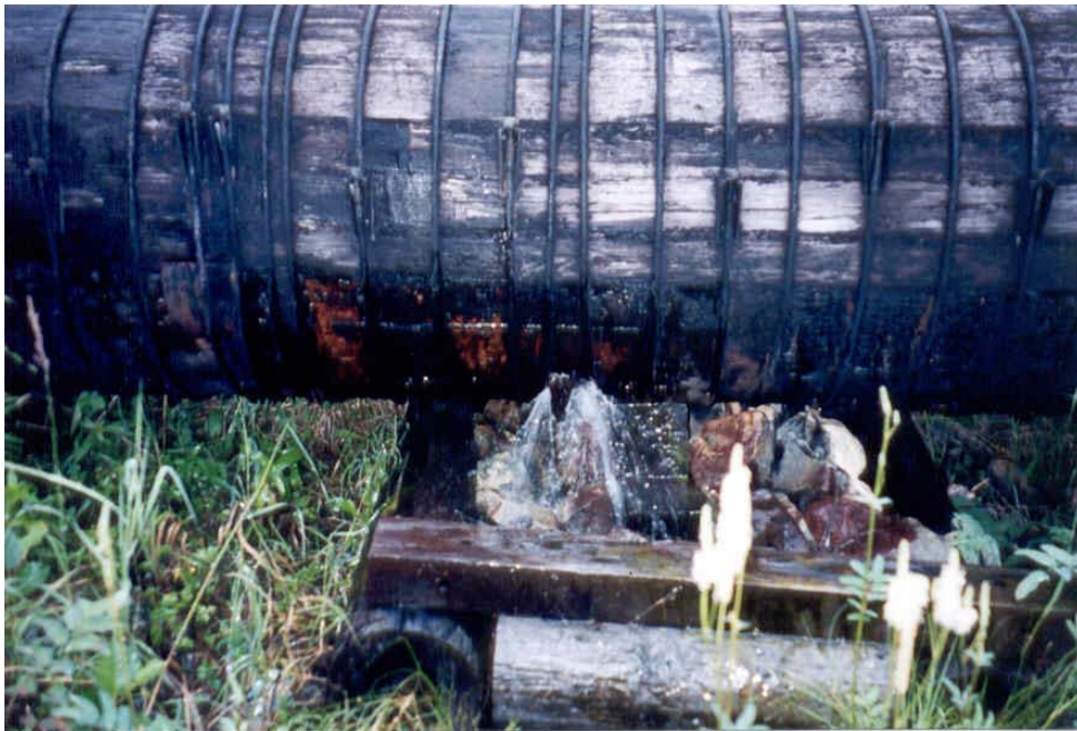
Photo #9: Water leaking from penstock, August 2000.
