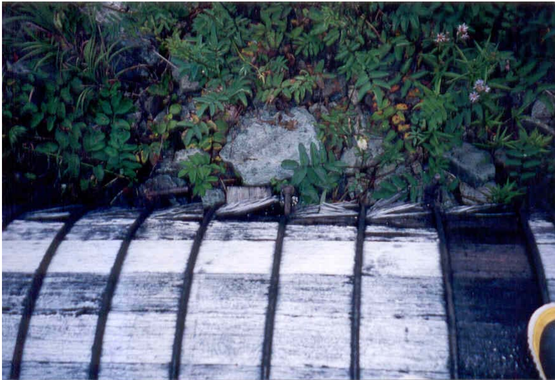
Photo #3: View of brooming between metal bands, August 2000.
