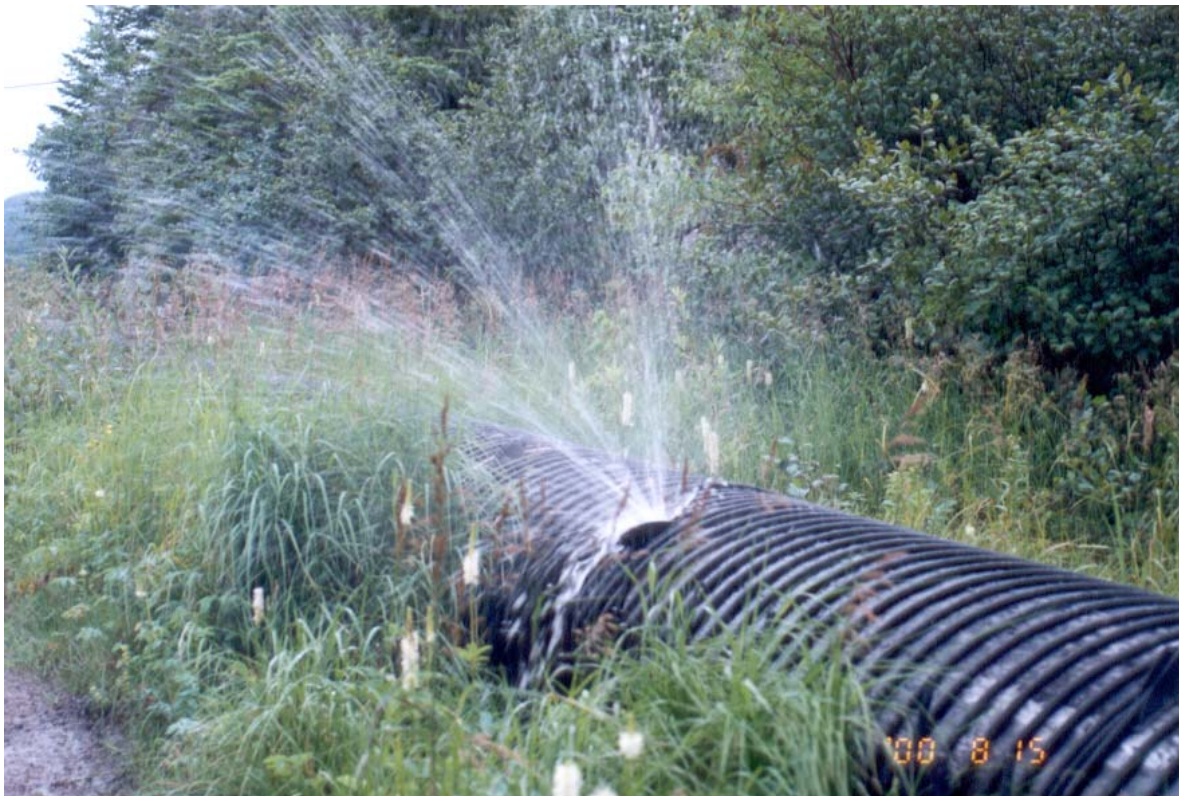
Photo 11: View of water leaking from penstock, August 2000.
