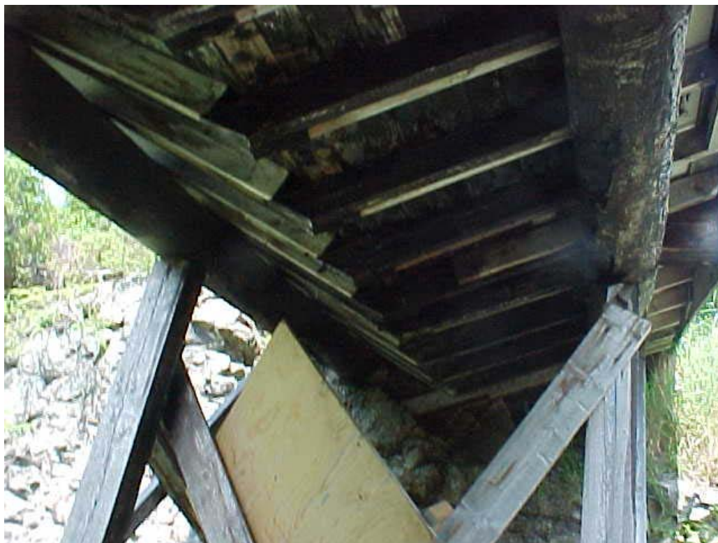
Photo 19: Support structure for penstock enclosure, July 2002.
