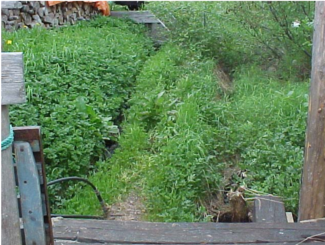
Photo #5: Vegetation growth around and on penstock, June 2001.
