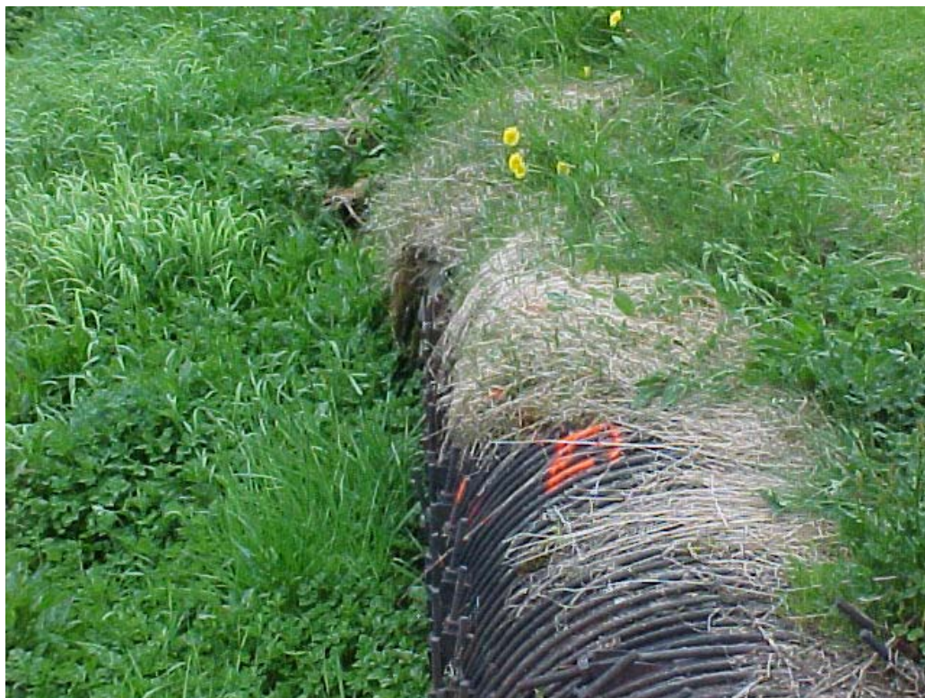
Photo #22 Buried section of penstock in community, June 2001.
