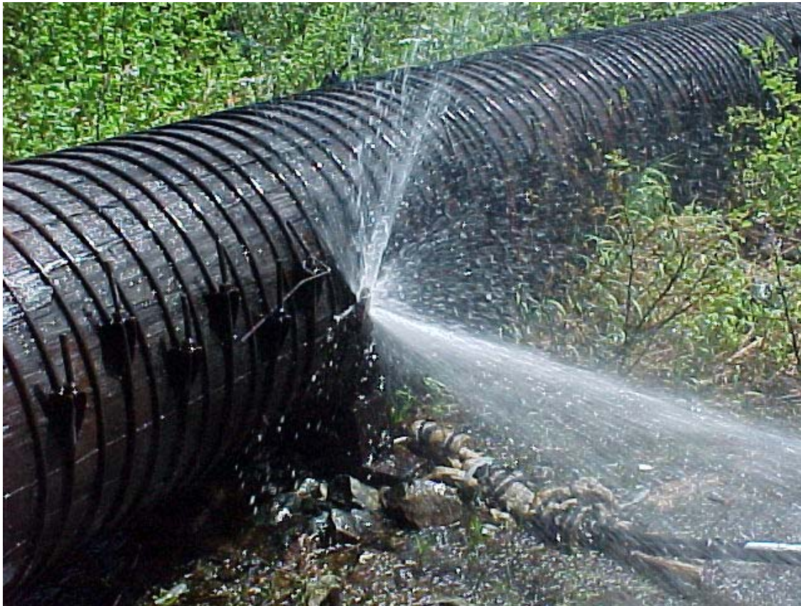
Photo #28: Location of abandoned water tap in penstock, June 2001.
