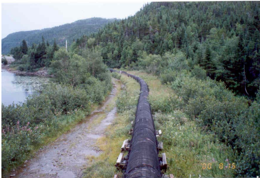
Photo #1: View of penstock, August 2000.
