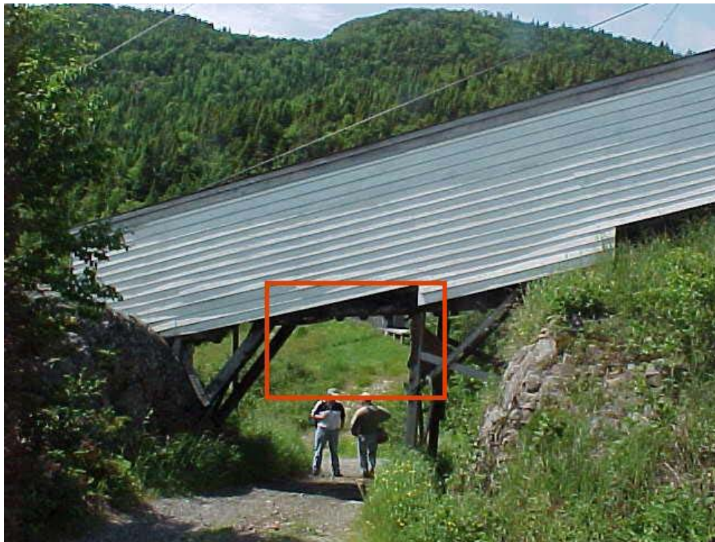
Photo 18: Penstock enclosure over access road, July 2002. Highlighted area indicates location of ice formation shown in Photo #15.
