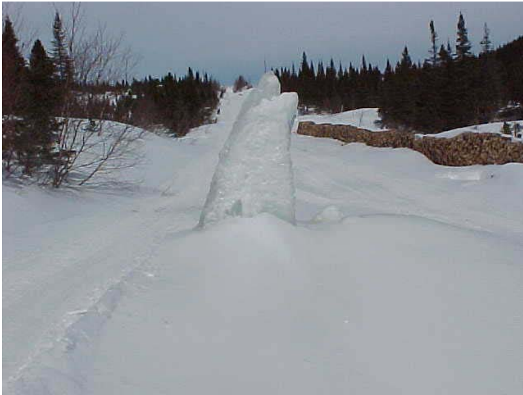
Photo 14: Ice formation above penstock, April 2001.
