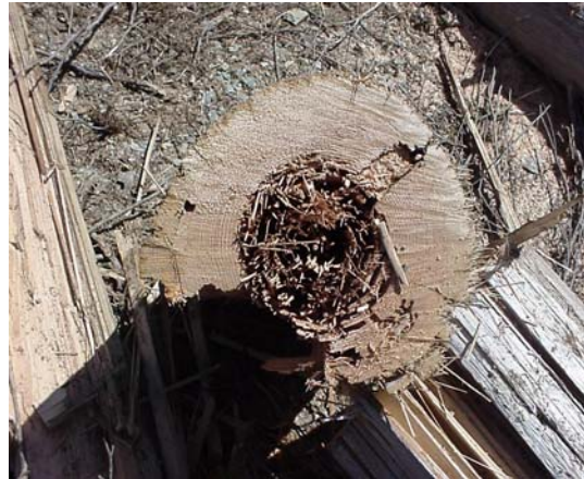
Fig. 3.19b – Carpenter Ant Damage
