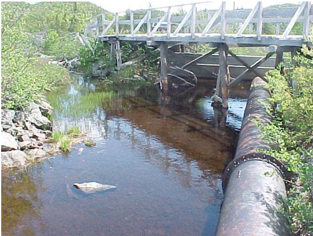
Photo #16: Accumulation of water behind concrete cut-off dam, June 2001.
