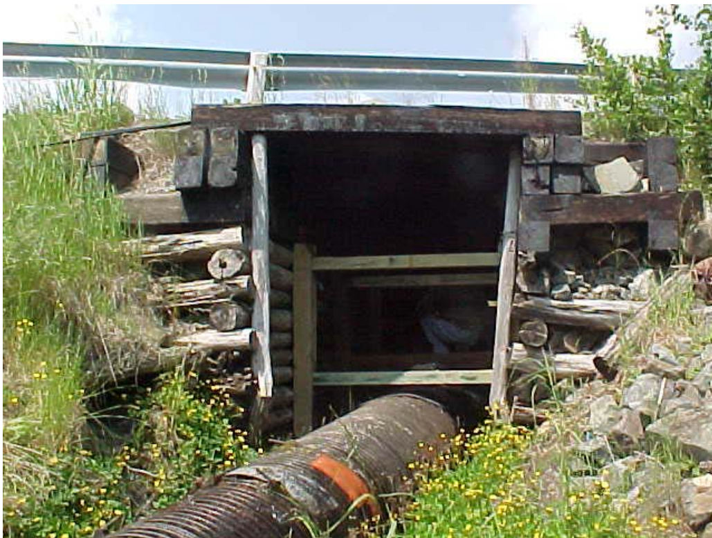
Photo 24: Road bridge over penstock, note timber reinforcement between abutments, July 2002.
