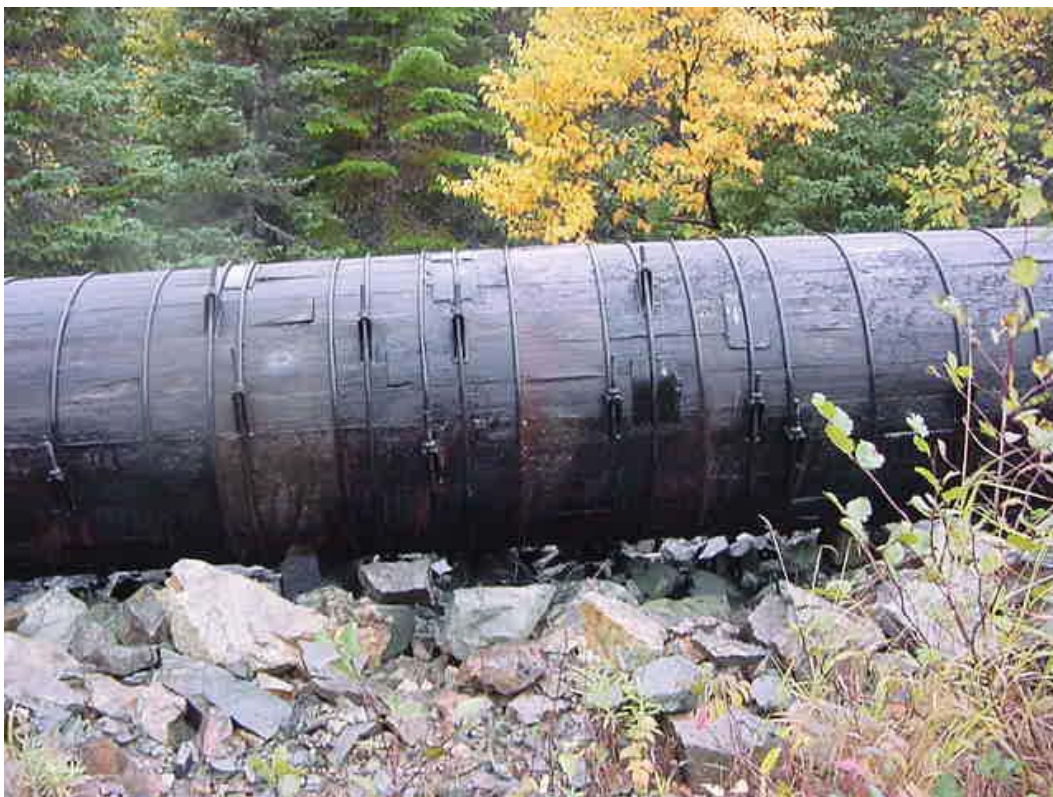
Photo #13: Metal patches placed under new bands to stop leaks, October 2003.
