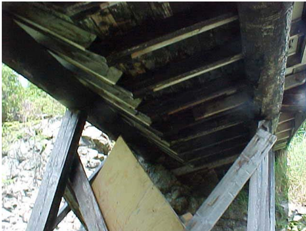
Photo 19: Support structure for penstock enclosure, July 2002.
