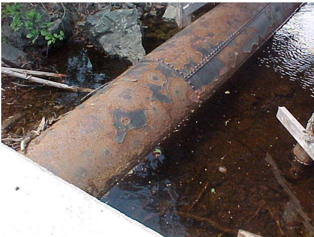
Photo #17: Steel section of penstock, partially submerged in water, June 2001.
