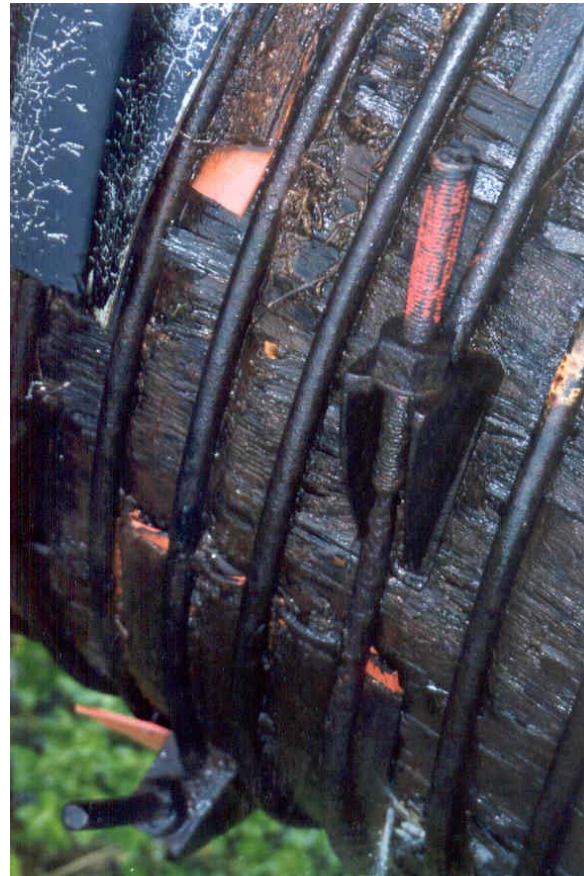
Photo #8: View of corrosion on metal bands, August 2000.
