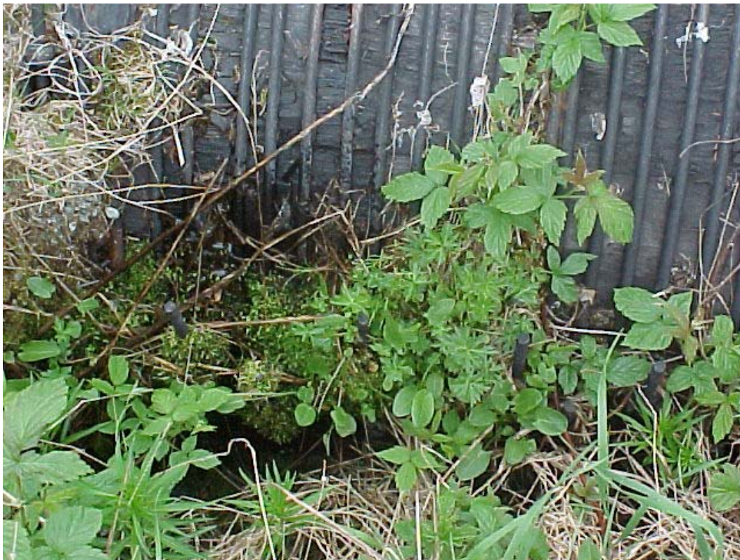
Photo #6: Moss and other vegetation growing directly on penstock, June 2001.
