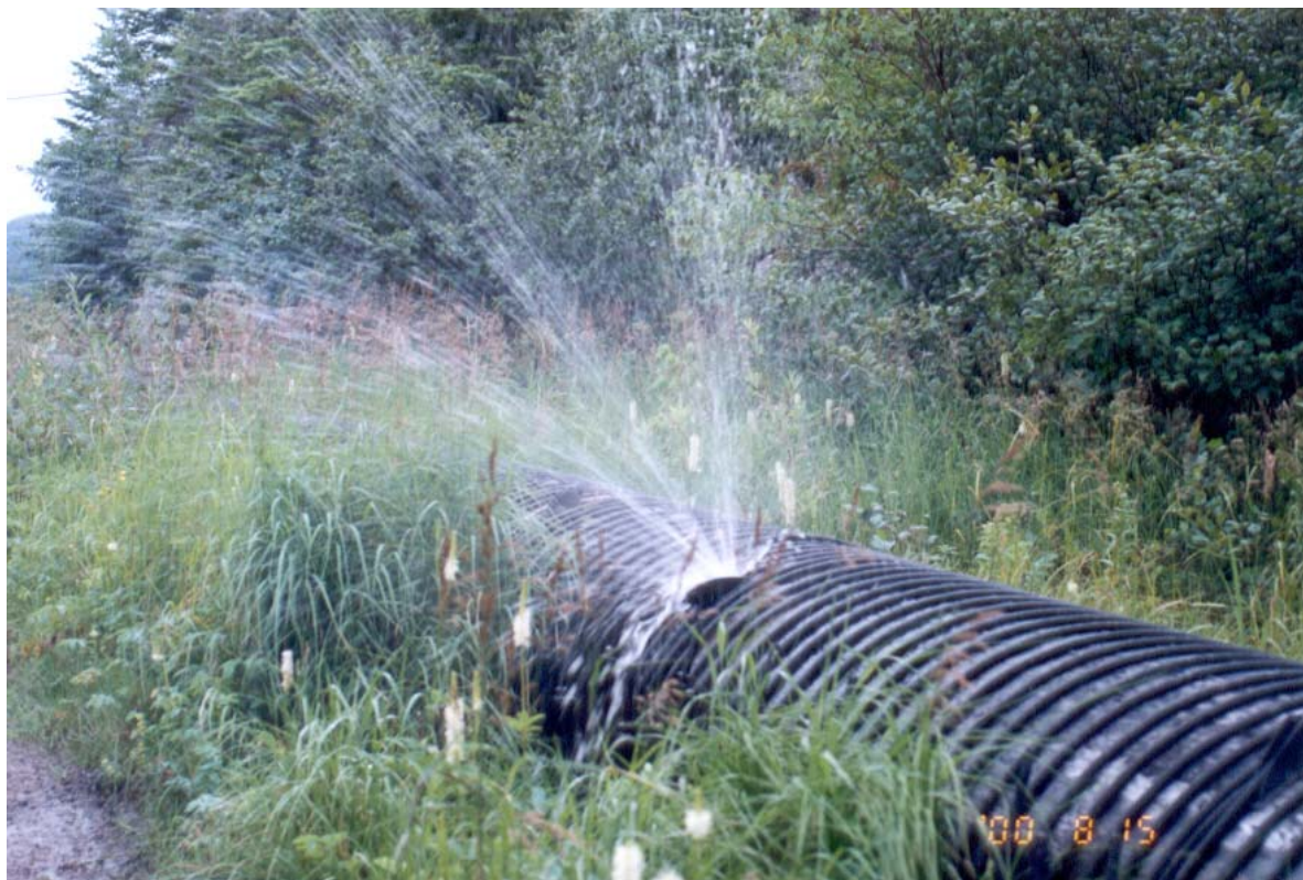
Photo 11: View of water leaking from penstock, August 2000.
