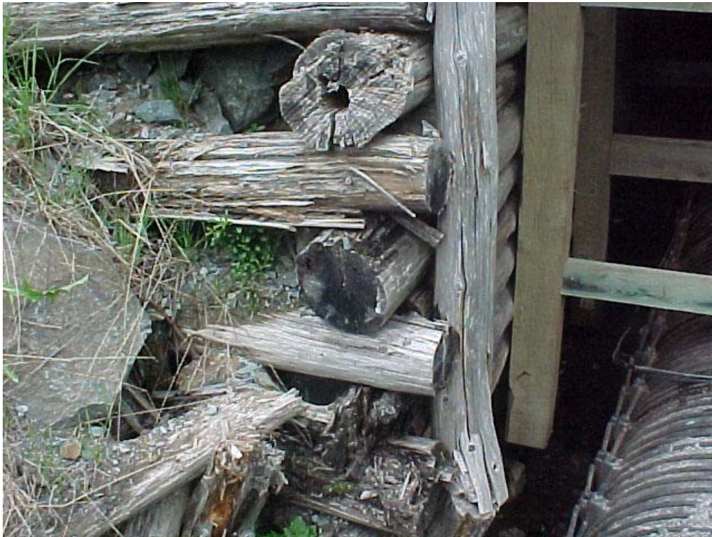
Photo 23: View of bottom portion of bridge abutment, June 2001.
