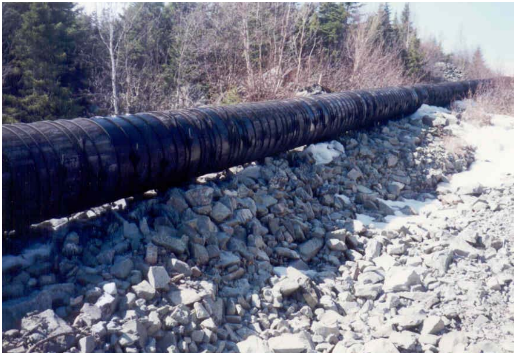
Photo #32: View of rocks and gravel washed up against penstock, April 1996.
