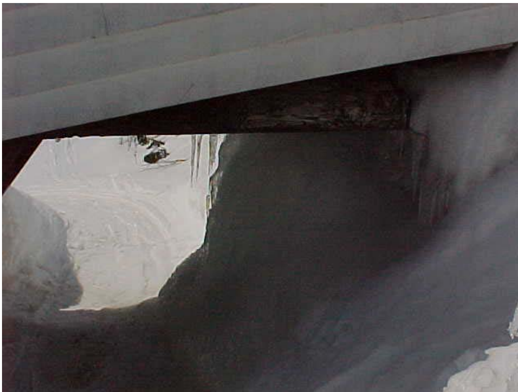
Photo 15: Ice formations under penstock enclosure, April 2001. For location of ice formation refer to Photo #18.
