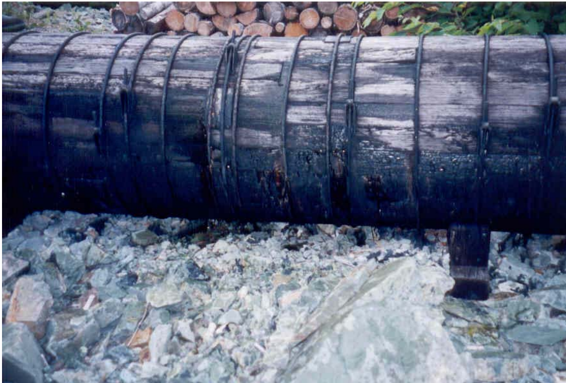
Photo #33: View of rocks and gravel under penstock, August 2000.
