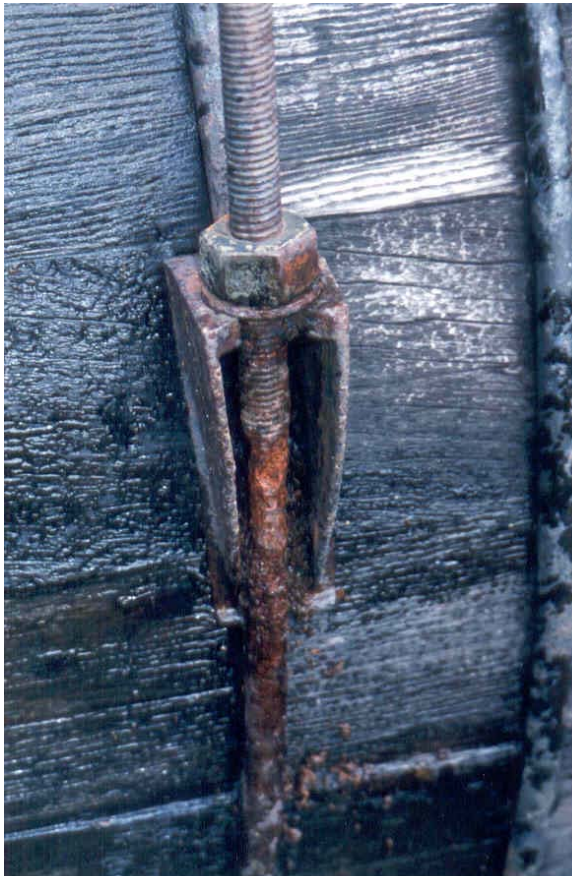
Photo #7: View of corrosion below threads, August 2000.
