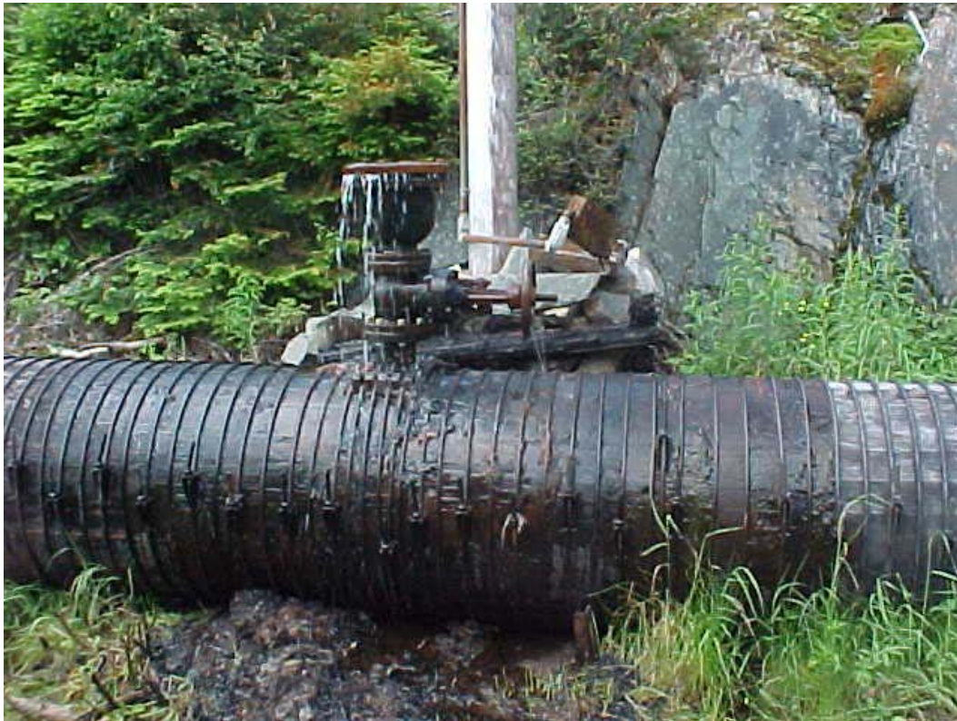
Photo 35: Vacuum breaker valve after fire, July 2002.
