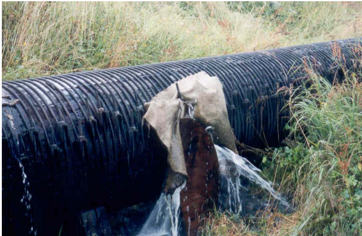
Photo #10: Water leaking from penstock, August 2000.
