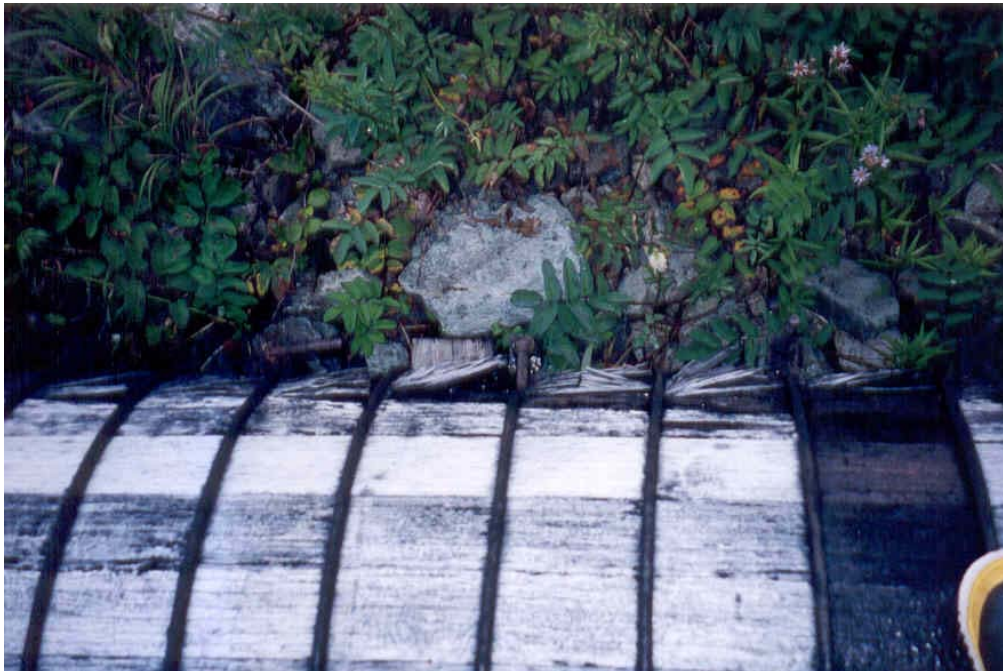
Photo #25: Loss of protective coating on penstock and bleaching of the wood, August 2000.
