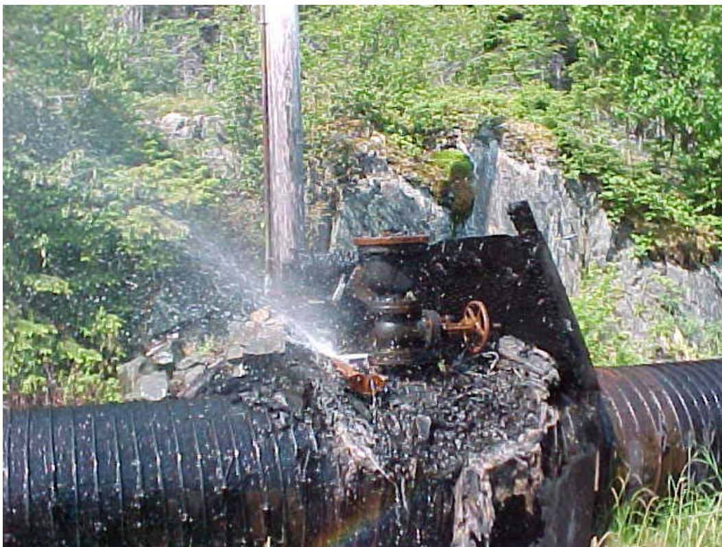
Photo 34: Fire damage to vacuum breaker valve enclosure, July 2002.
