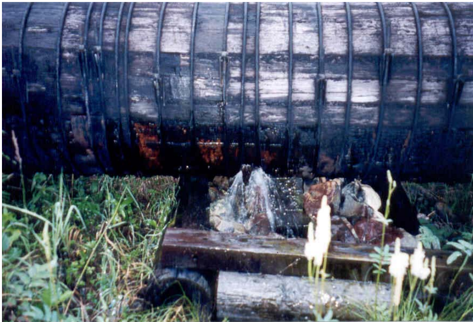
Photo #9: Water leaking from penstock, August 2000.
