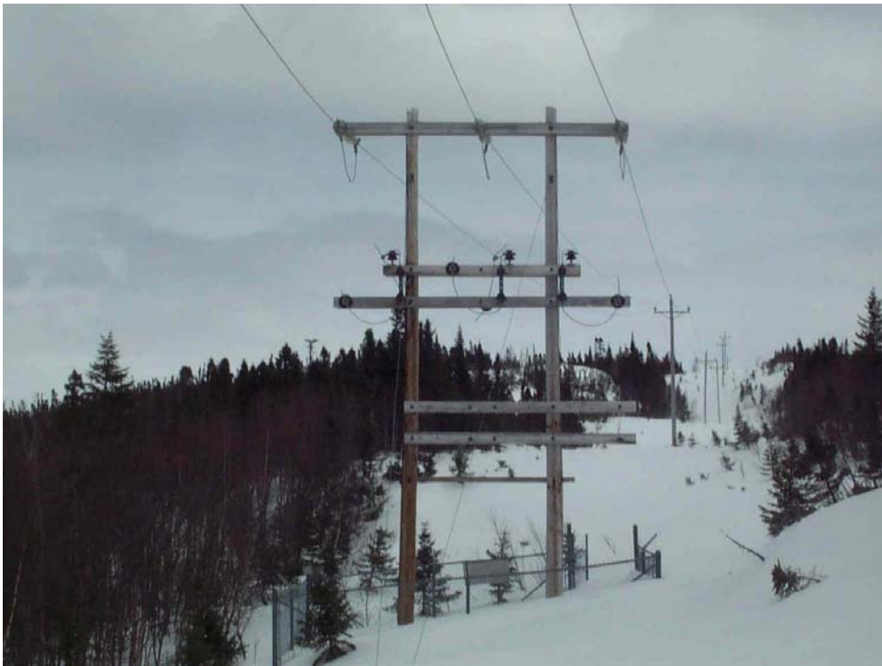
Figure 5 Old Whalesback mine substation site
