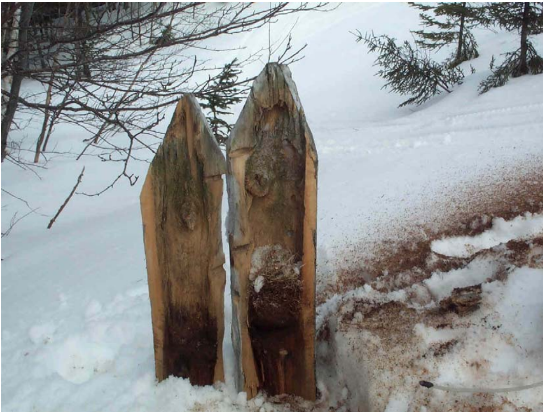
Figure 11 First 3 feet of pole replace in 2001. The top was completely hollow with bird's nest inside
