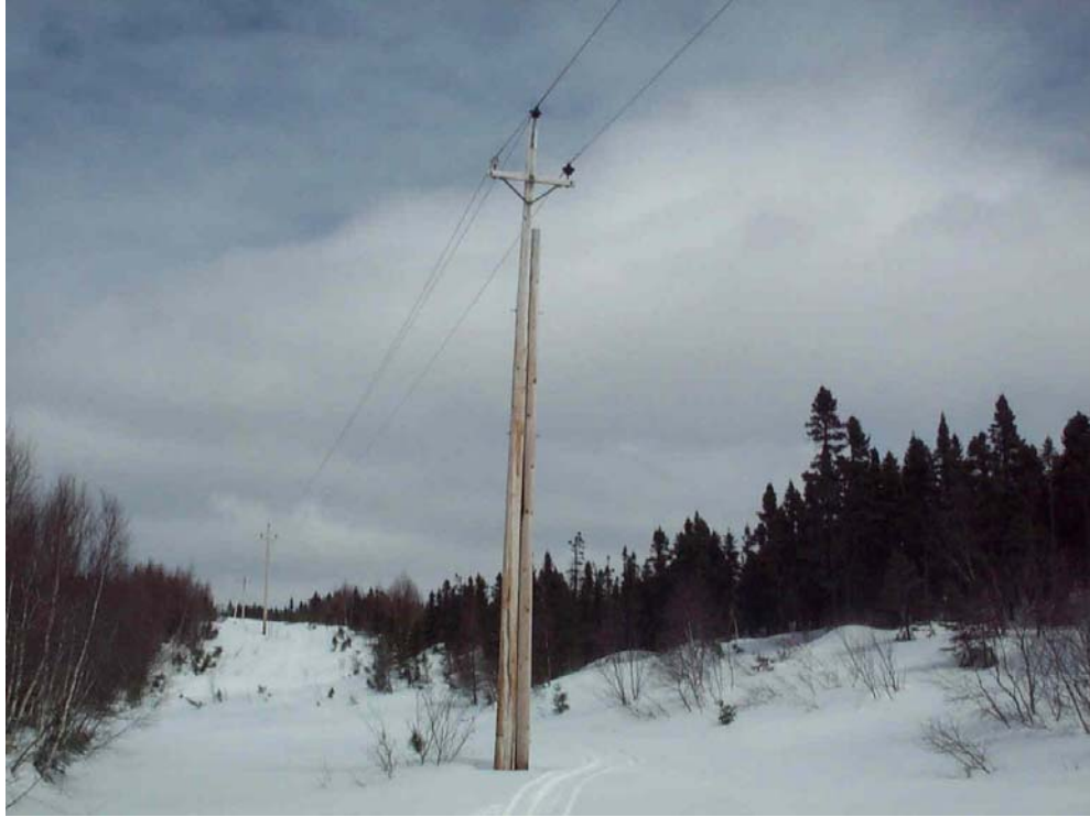
Figure 10 A second structure with a repair by bolting second pole
