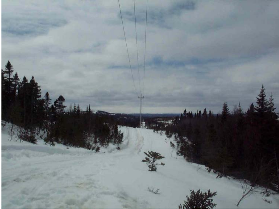
Figure 4 Note span length
