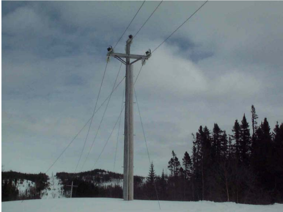
Figure 6 This and following 3 figures show a split pole with repair by bolting second pole
